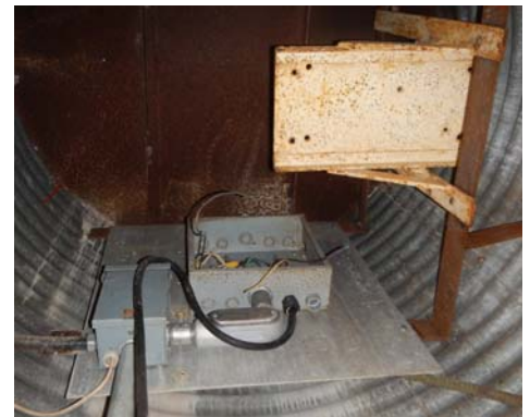
Below: existing hydro disconnected
