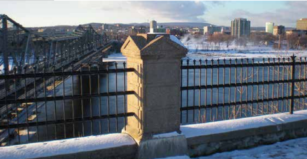
Masonry Wall with Iron Fence
