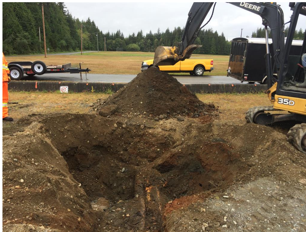
Photo 6: Facing west – looking at logs and subsurface conditions encountered within excavation where petroleum hydrocarbons were identified
