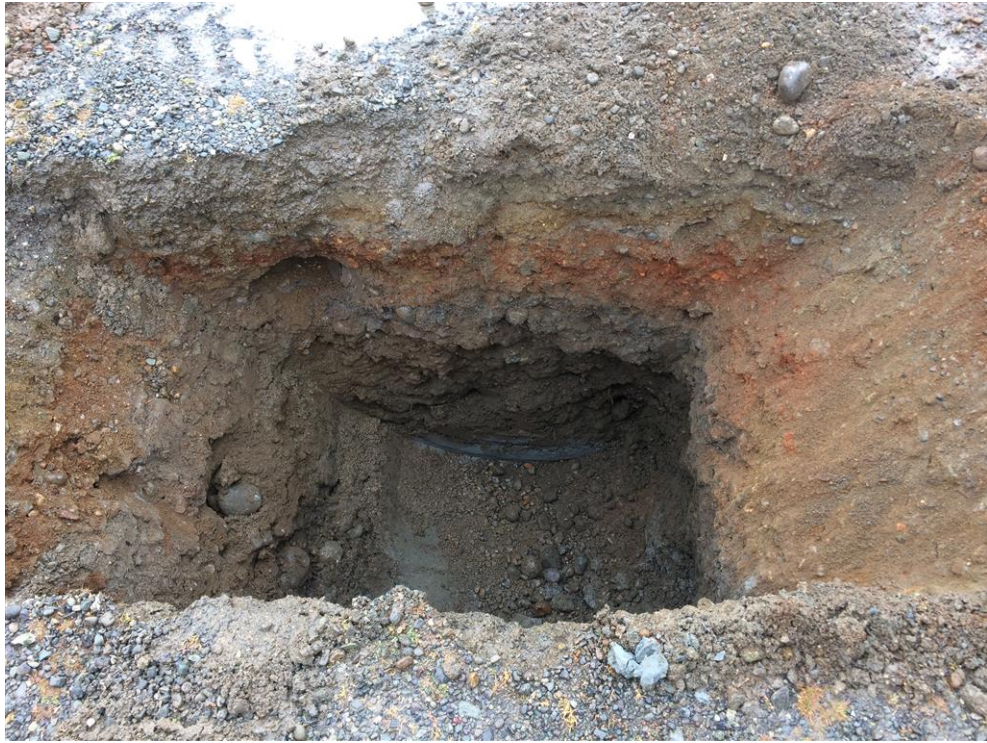
Photo 7: Looking at subsurface conditions encountered within test pit TPE
