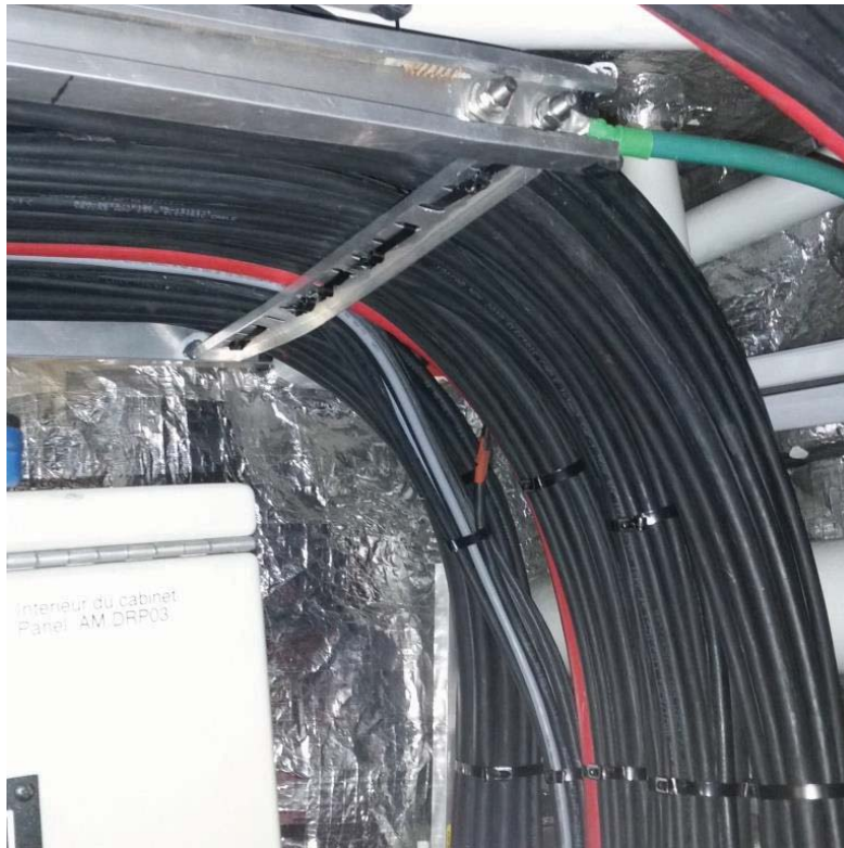
Figure 1: obstruction multi cable transit in control room
