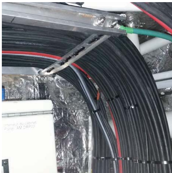
Figure 6: obstruction multi cable transit in control room
