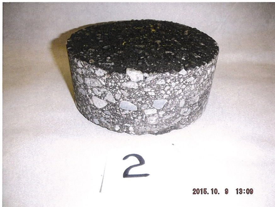
Photo 2: HA15-02 Asphalt Core, 65mm thick
