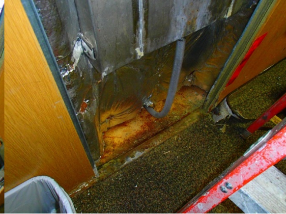
Figure 18: Flexible hose connection under reservoir
