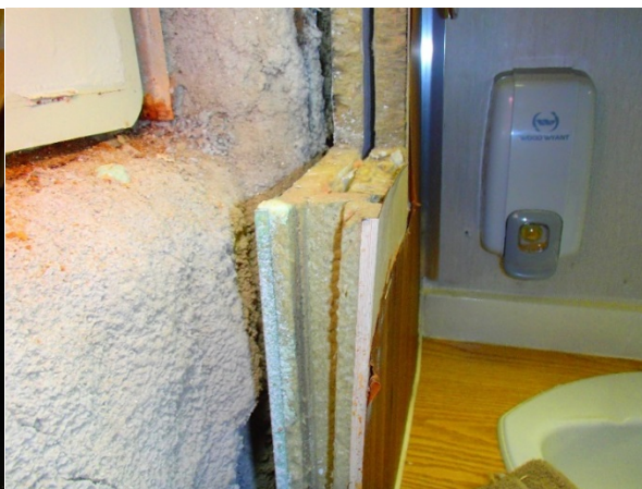
Figure 14 : Panneau type Joiner 50mm (2")
