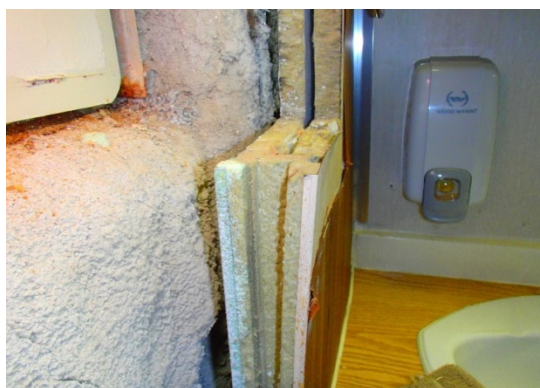
Figure 14: Typical 50mm (2'') Joiner panel
