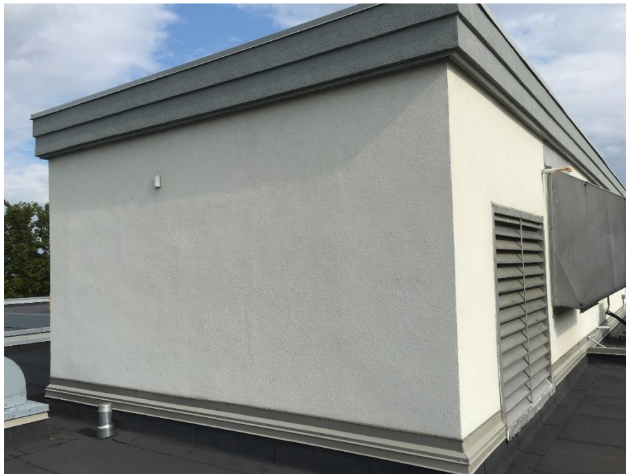
Photo 4: Exterior stucco on the north Penthouse Mechanical Room, contains 0.5-5% Chrysotile.
