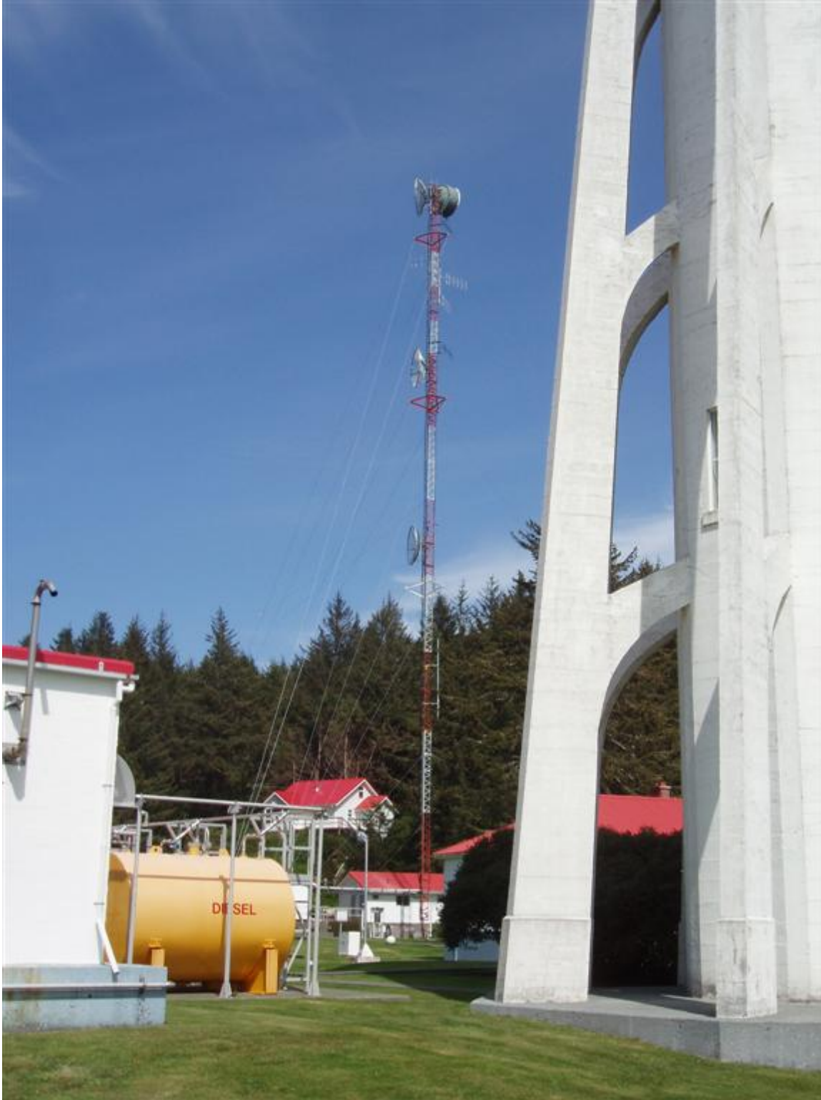
Existing Communications Tower
