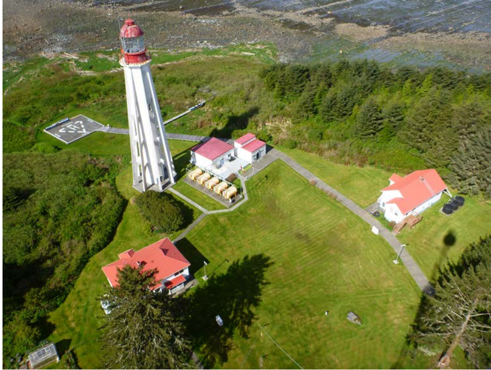
View from existing tower
