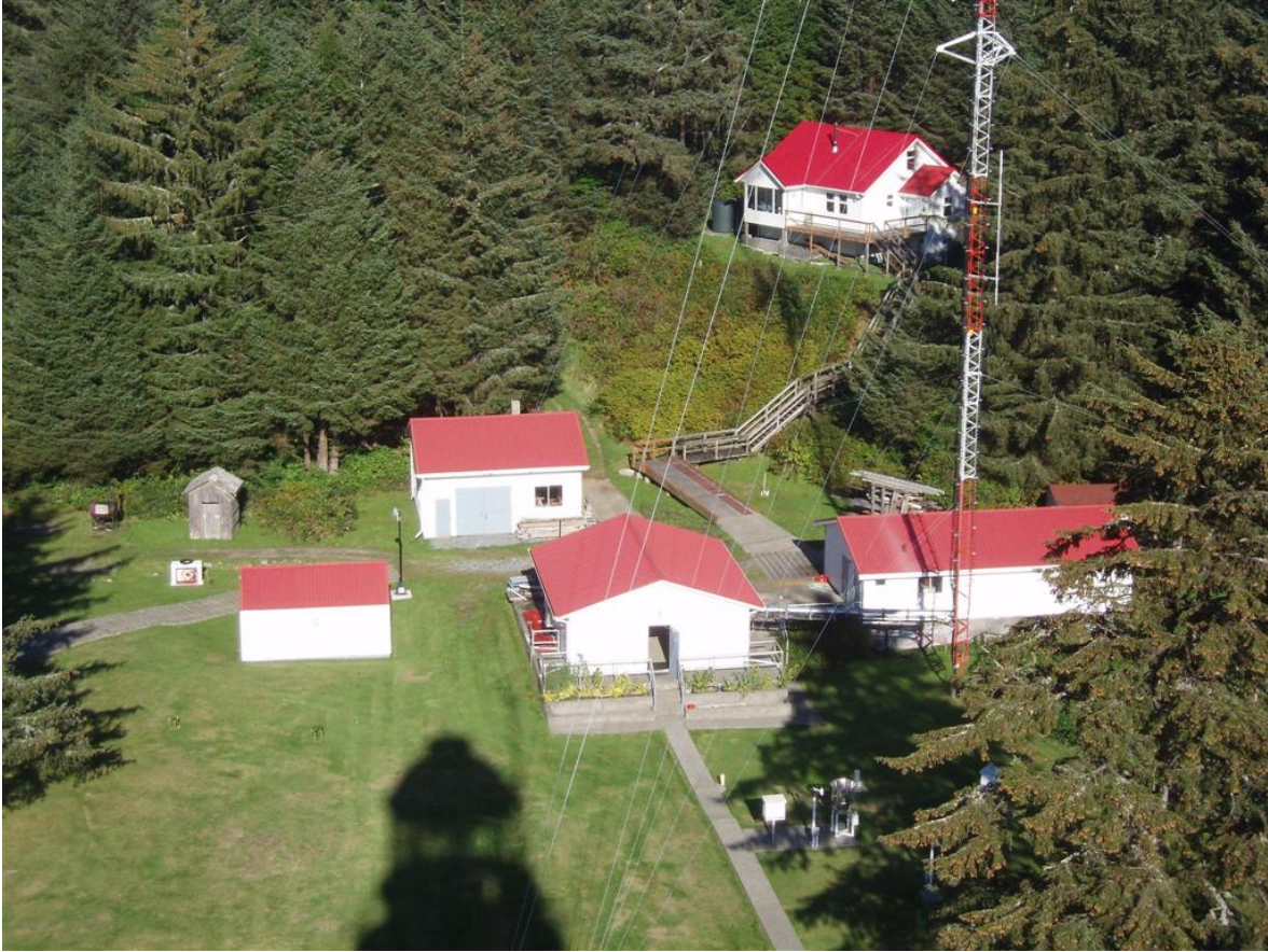
Crew House (top), Radio Building (center) and Existing Tower
