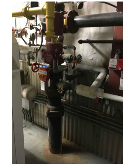
5A M102 FIRE SPRINKLER SYSTEM
