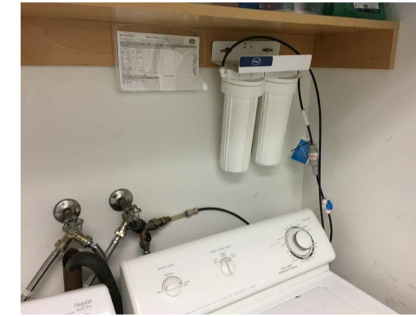
3B M102 WATER SUPPLY TO WATER COOLER
