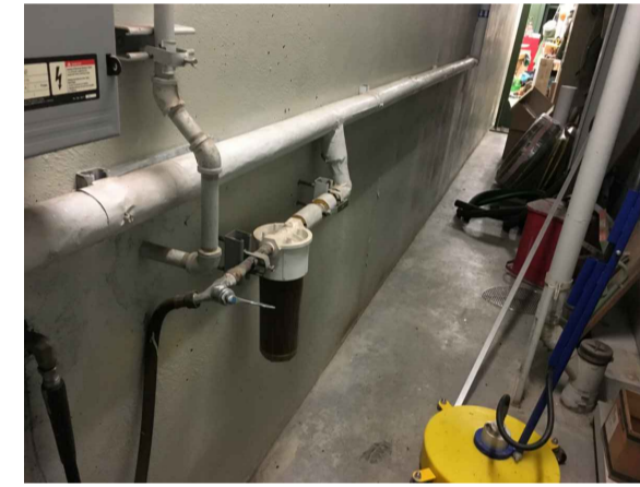
3A M102 WATER SUPPLY TO PRESSURE WASHER
