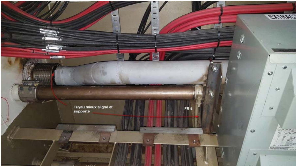
Figure 3: support bracket for vent line Fr 5
