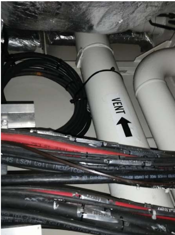
Figure 1: vent line installed in the steering compartment
