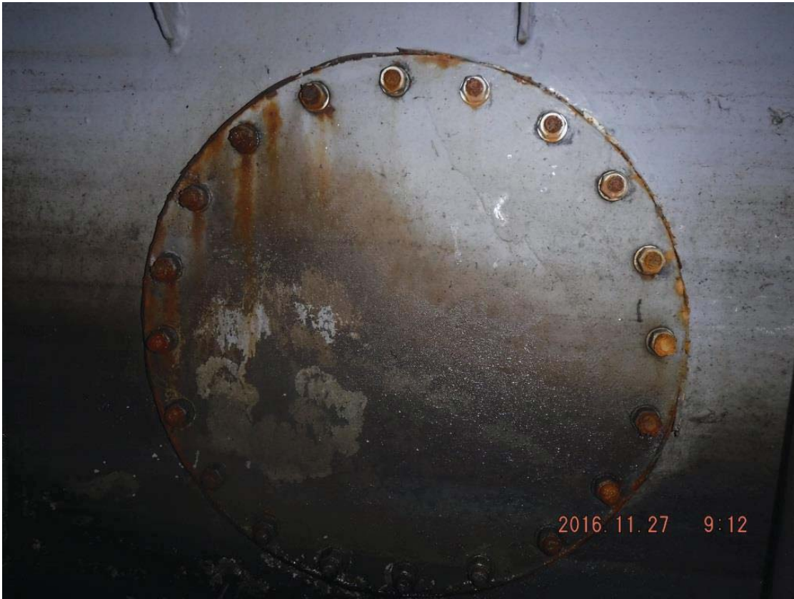
Figure 7: manhole to the black water tank inside the the grey water tank
