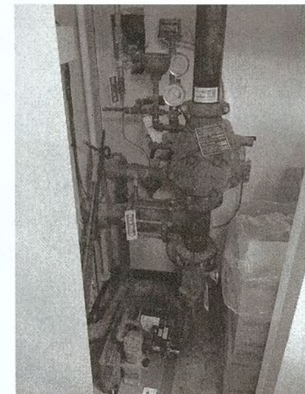
1B M102 FIRE SPRINKLER SYSTEM
