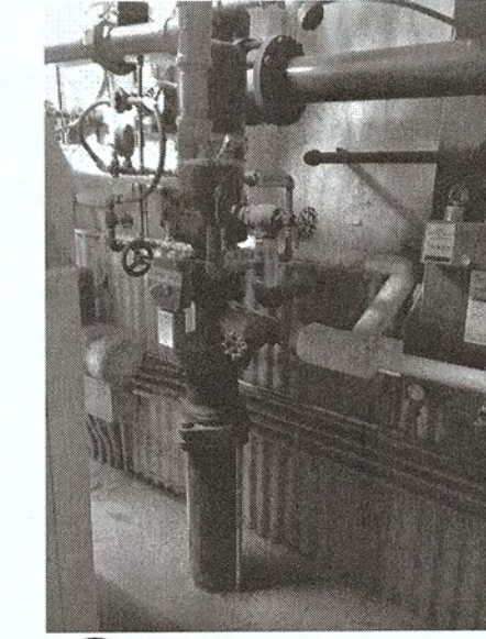
5A M102 FIRE SPRINKLER SYSTEM
