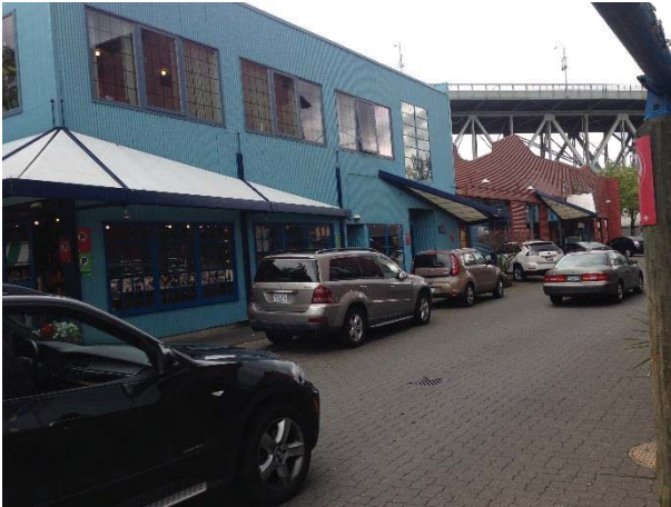
Photo 1: View of the Net Loft building (south side).
