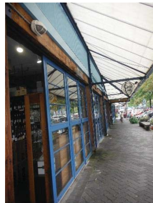
Photo 6: View of the Net Loft building (west side).
