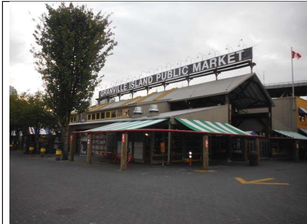
Photo 1: View of the Public Market building (west portion).
