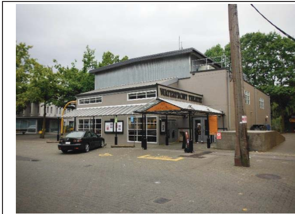
Photo 1: View of the Waterfront Theatre building from Cartwright Street.
