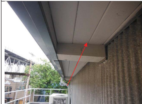
Photo 3: Sample B3-L4 of white paint present at the wooden panels (Roof). The paint contains more than 0.06% lead.
