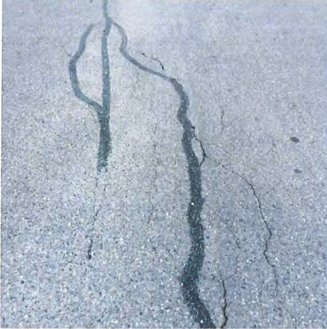
Photo 3: Longitudinal crack and alligator cracking of asphalt
