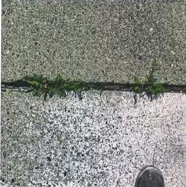
Photograph 2 – exposed aggregate, slab edge broken and vegetation growth
