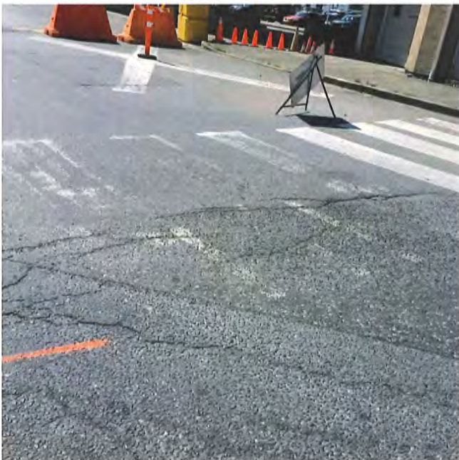
Photograph 5 – Cracked asphalt of commercial lane and light vehicles
