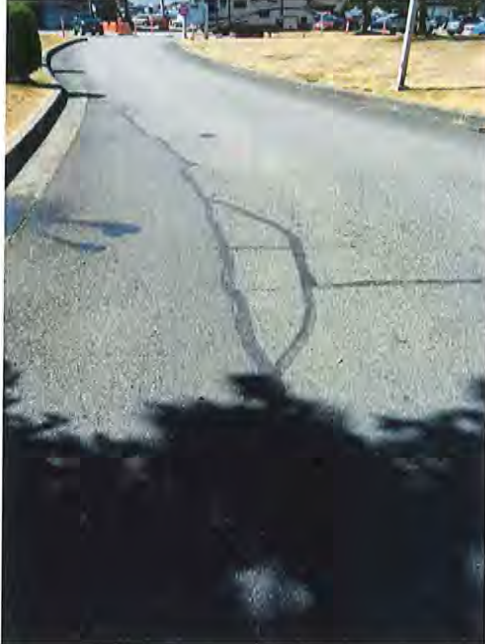
Photo 8: Transverse crack in pavement
