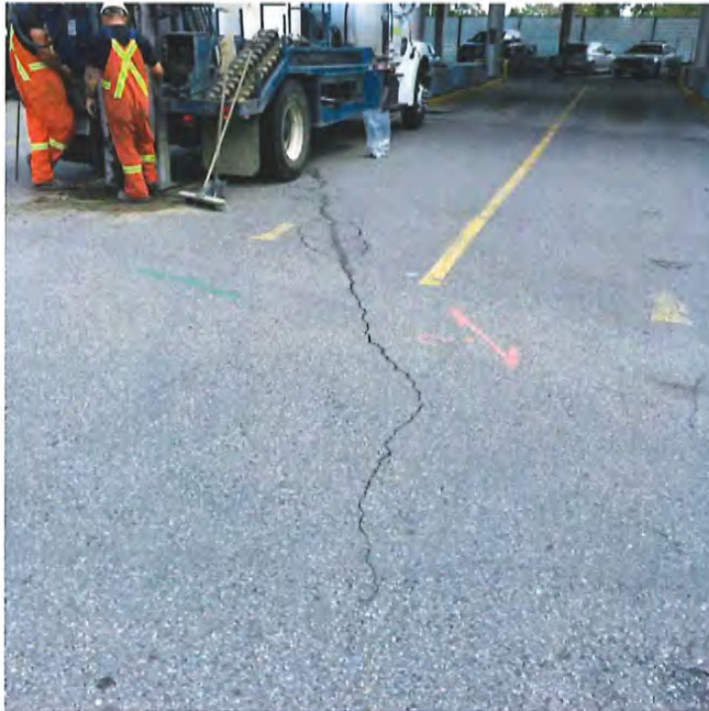
Photo 3: Longitudinal crack and alligator cracking of asphalt
