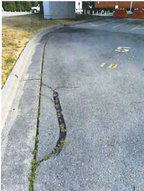
Photo 6: Cracking along curb
