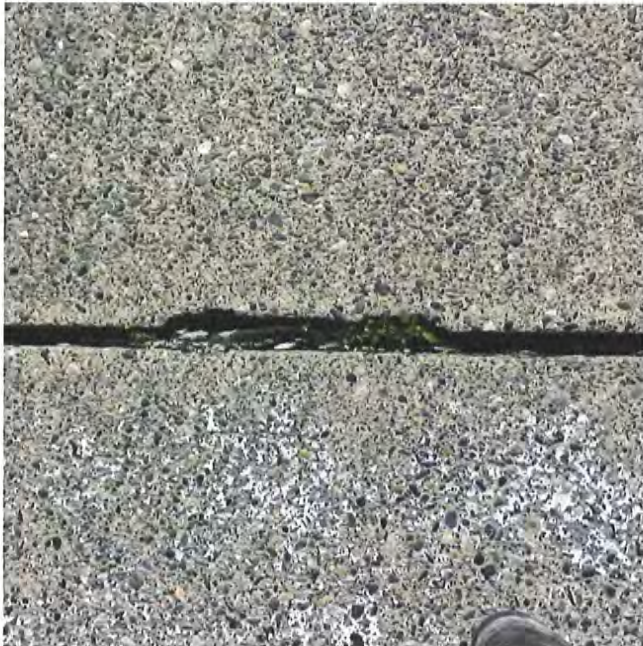
Photograph 2 – exposed aggregate, slab edge broken and vegetation growth
