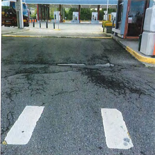
Photo 5: Cracking of asphalt along bus travel path
