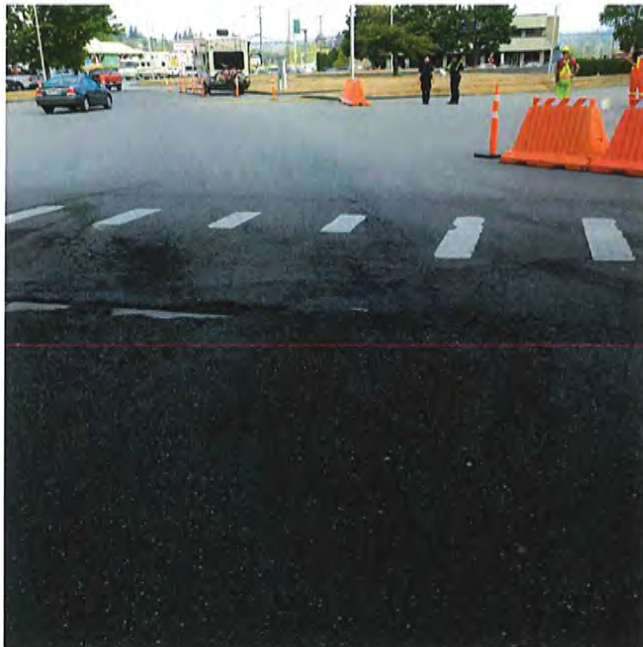
Photo 5: Cracking of asphalt along bus travel path
