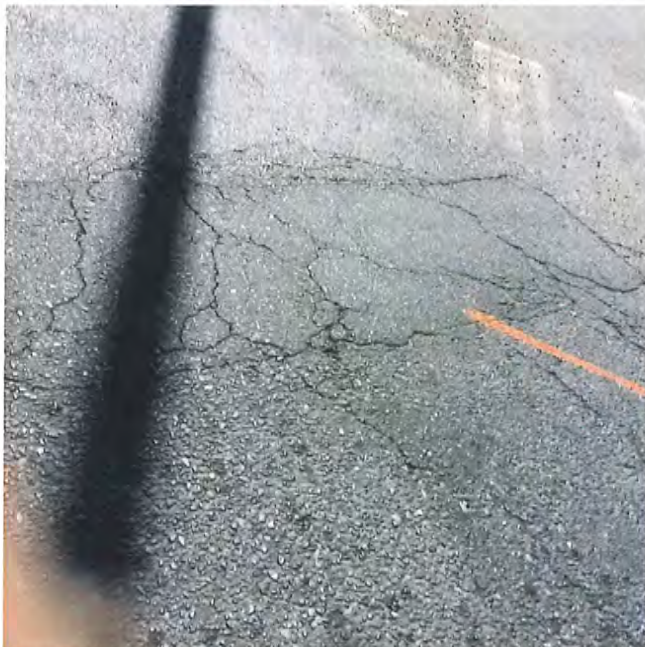
Photograph 5 – Cracked asphalt of commercial lane and light vehicles
