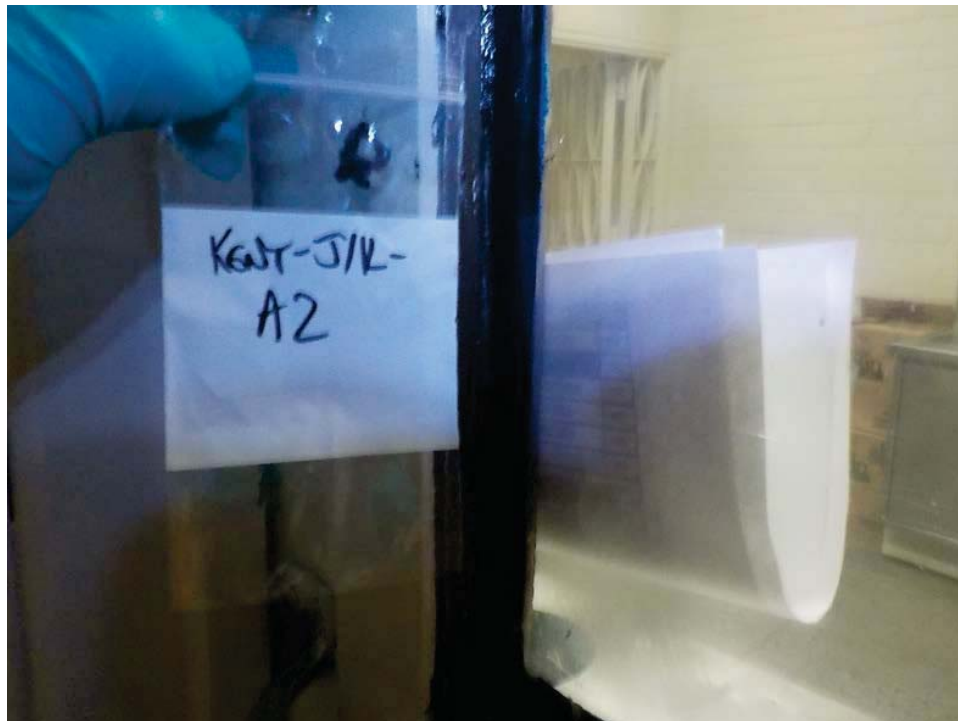
Photograph 4: Non-Asbestos grey mastic between the window pane and frame on the door facing Living Unit J kitchen.
