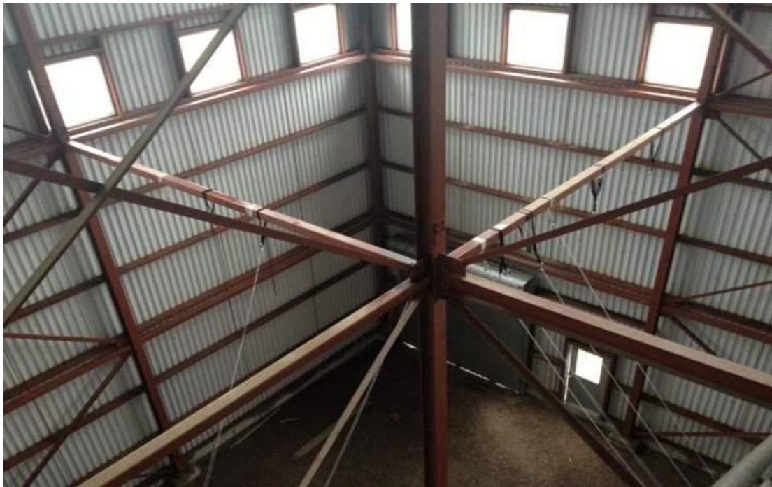
Alternate (2 nd ) Training Building for Customized Working Aloft Course
