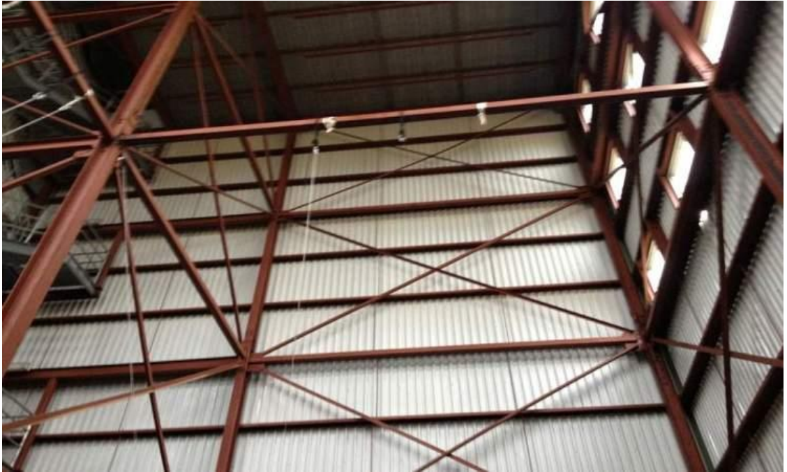
Alternate (2 nd ) Training Building for Customized Working Aloft Course
