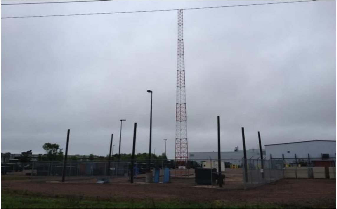
Self Support Communications Tower (Site Two)
