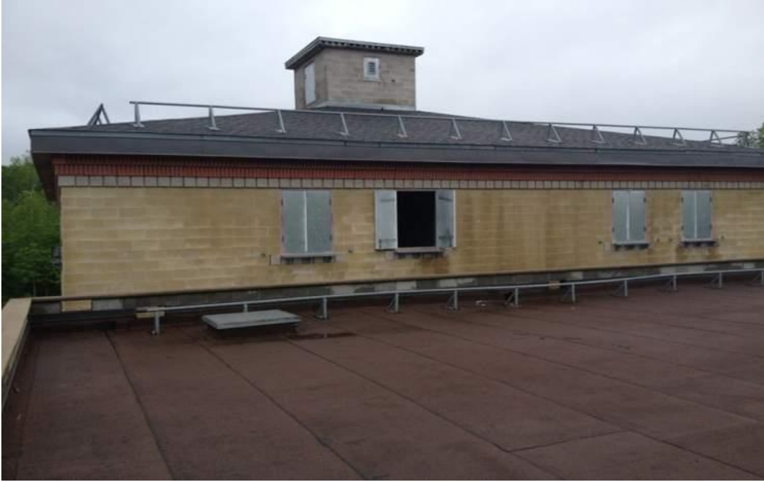
Rooftop with Anchors for Customized Training (Site One )
