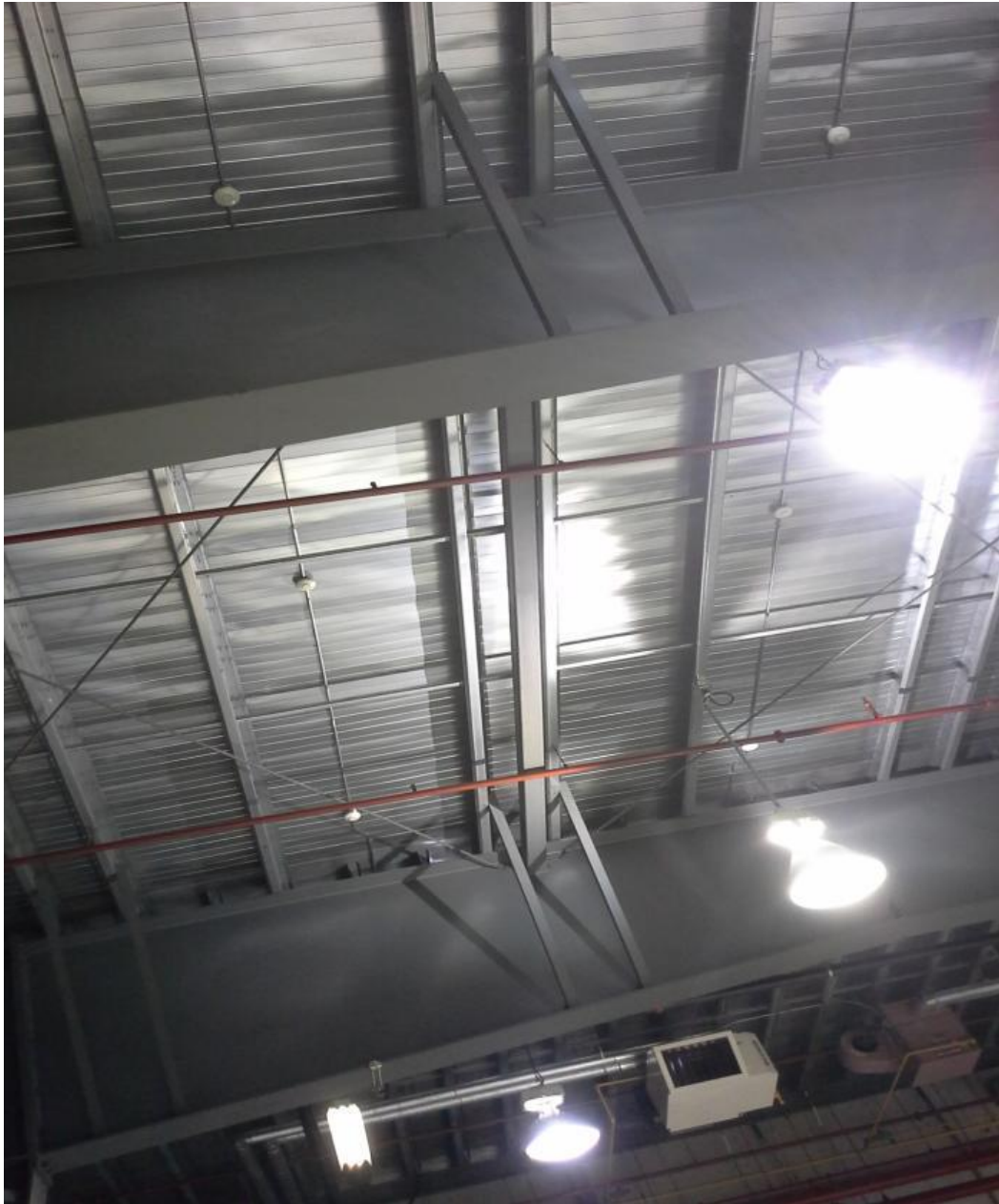
Primary Training Hall for Customized Working Aloft Course
