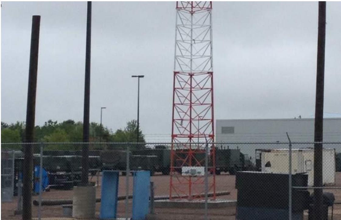
Self Support Communications Tower
