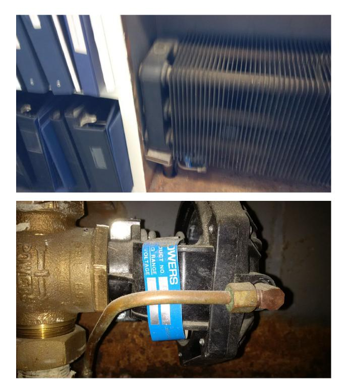
Typical photos of existing through the floor piping where new DDC hydronic control valves are to be installed.
