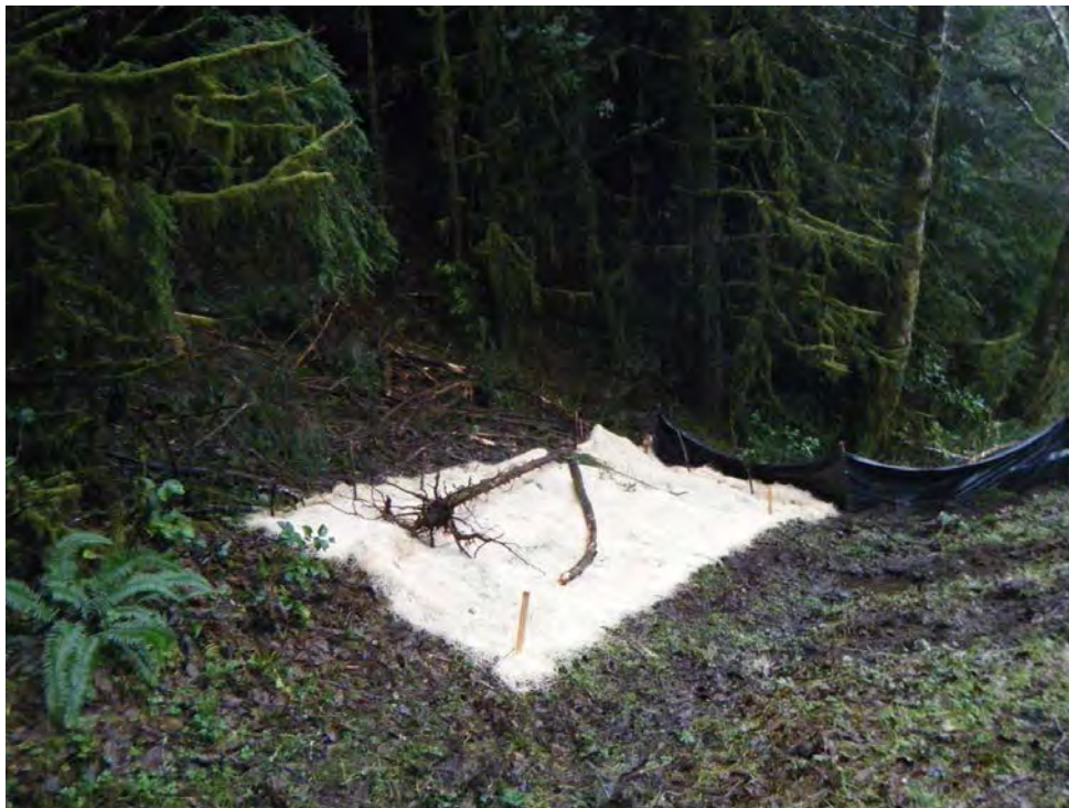
Photo 18: Typical erosion protection measures during test pitting (22-Nov-2016)
