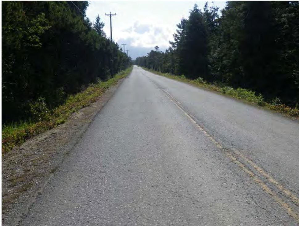
Photo 1: Upper Wick Road looking east from ~Sta. 0+320 (27-May-2016)
