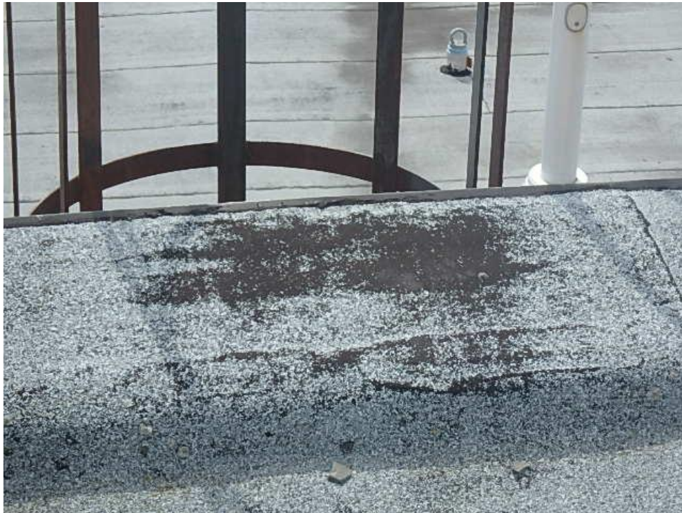
Photograph 29: Roof Area 3.1 – damaged membrane due to lack of protection at top of ladder.
