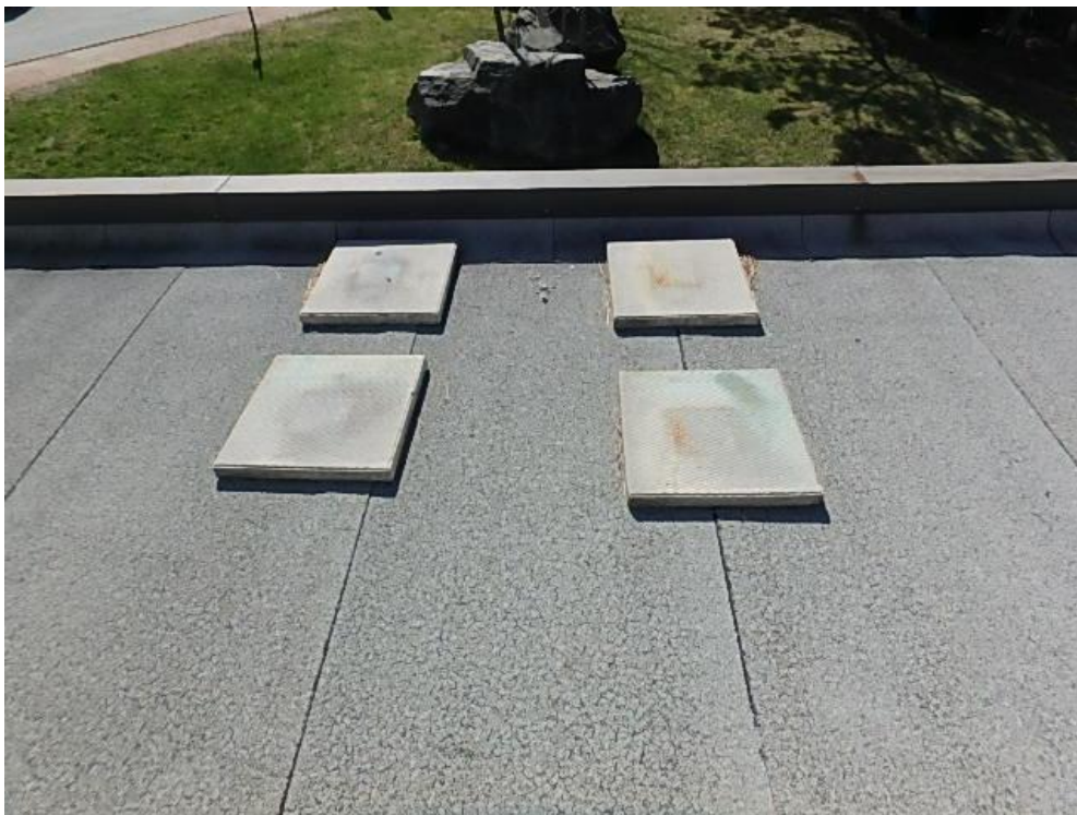
Photograph 12: Roof Area 1.1 – unused pavers sitting directly on membrane
