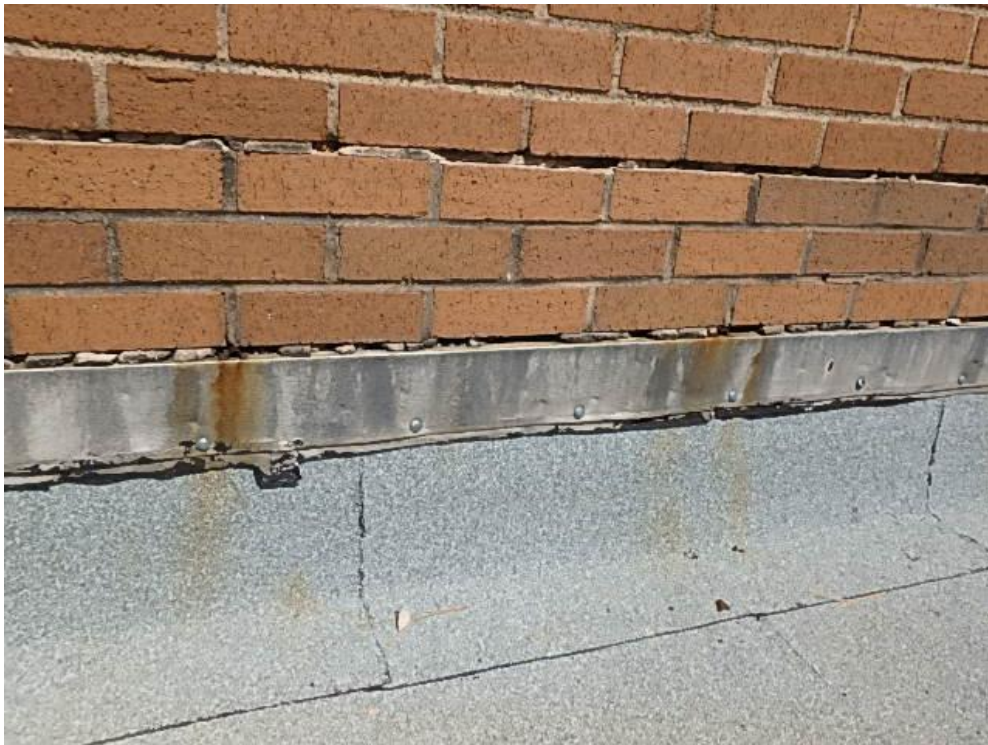
Photograph 42: Roof Area 2.3 – sealant missing at reglet and improperly sealed between flashing and membrane.
