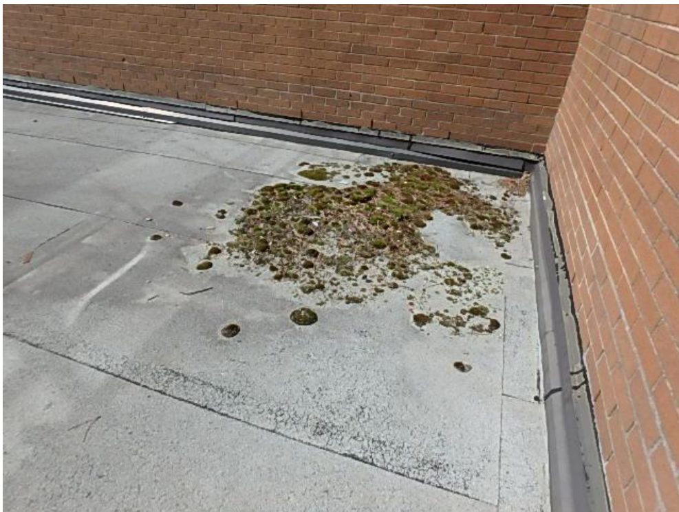
Photograph 6: Roof Area 1.1 – debris and vegetation growth at corner and showing poorly sealed reglet detail along wall transition
