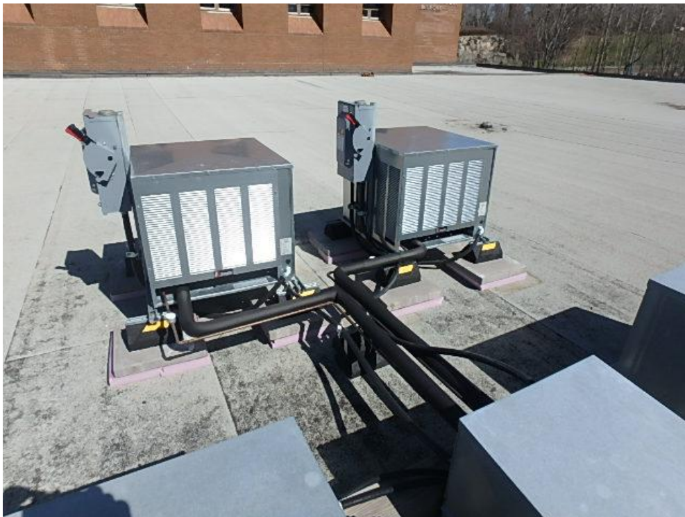
Photograph 10: Roof Area 1.1 – HVAC units on pavers with insulation membrane protection and conduits running to adjacent doghouse penetration.
