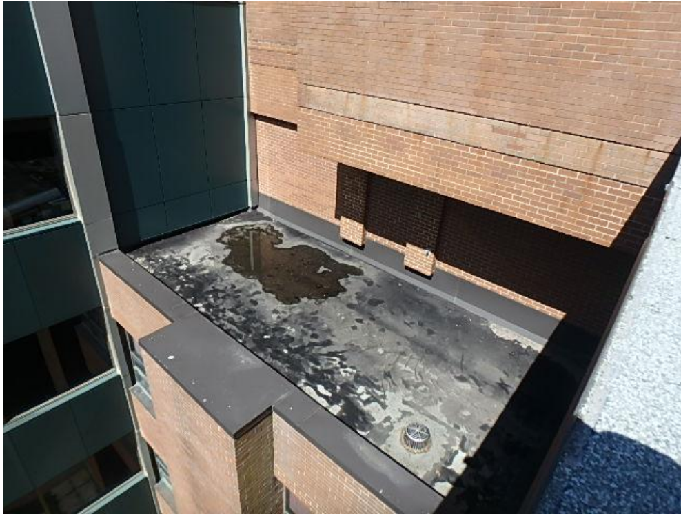
Photograph 45: Roof Area 2.4 – Roof area above entrance with no access from building or by ladder. There is evidence of ponding and membrane cracking in multiple locations.
