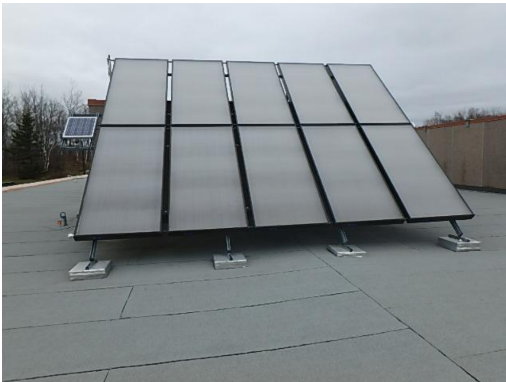
Photograph 16: Roof Area 2.1 – Solar panels on evenly spaced structural supports that are improperly flashed to cap sheet membrane.
