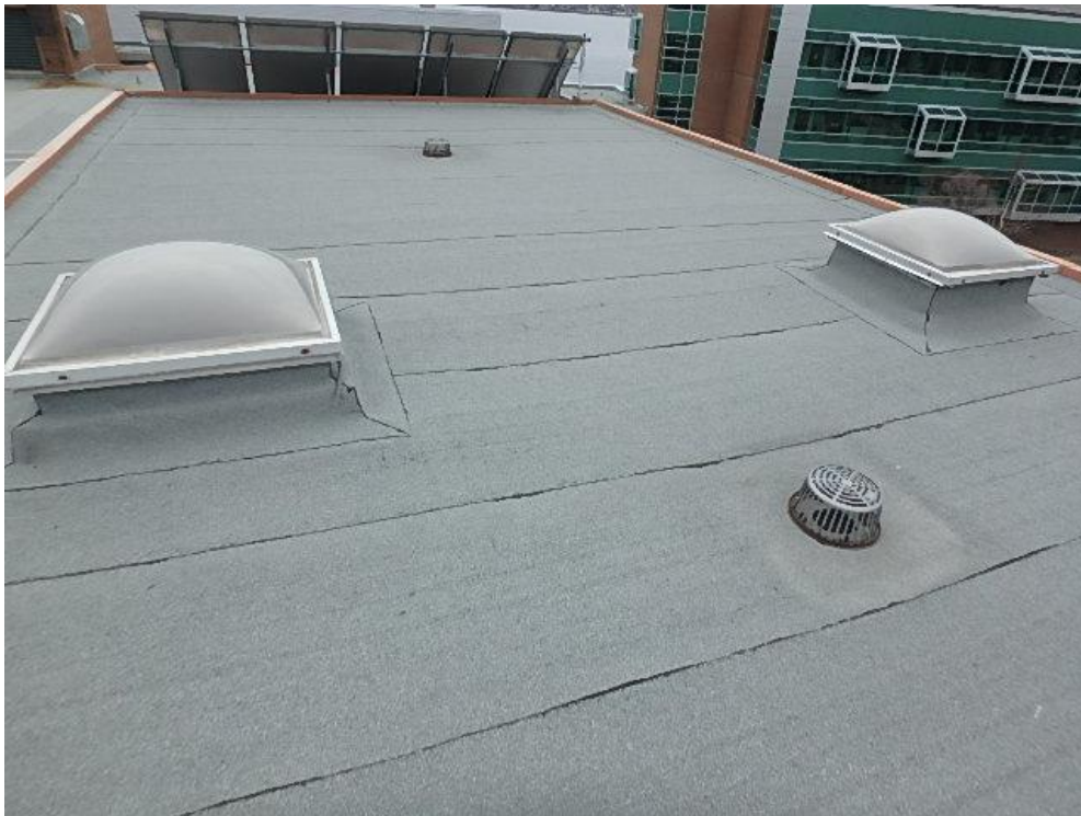
Photograph 26: Roof Area 3.2 – Overall view of roof area 3.2 facing south. Shows drains with improper cap sheet flashing, skylights, adjacent solar panels, and typical parapet. Roof is generally in good condition.
