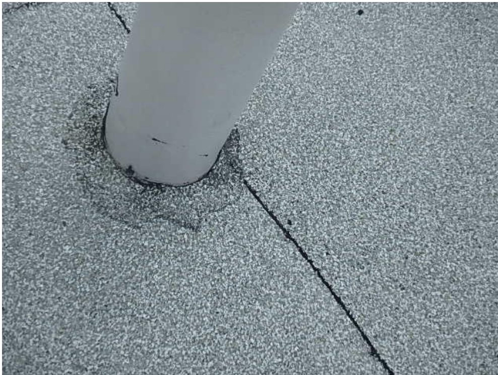
Photograph 54: Roof Area 3.1 –Typical flashing problem at plumbing stack.
