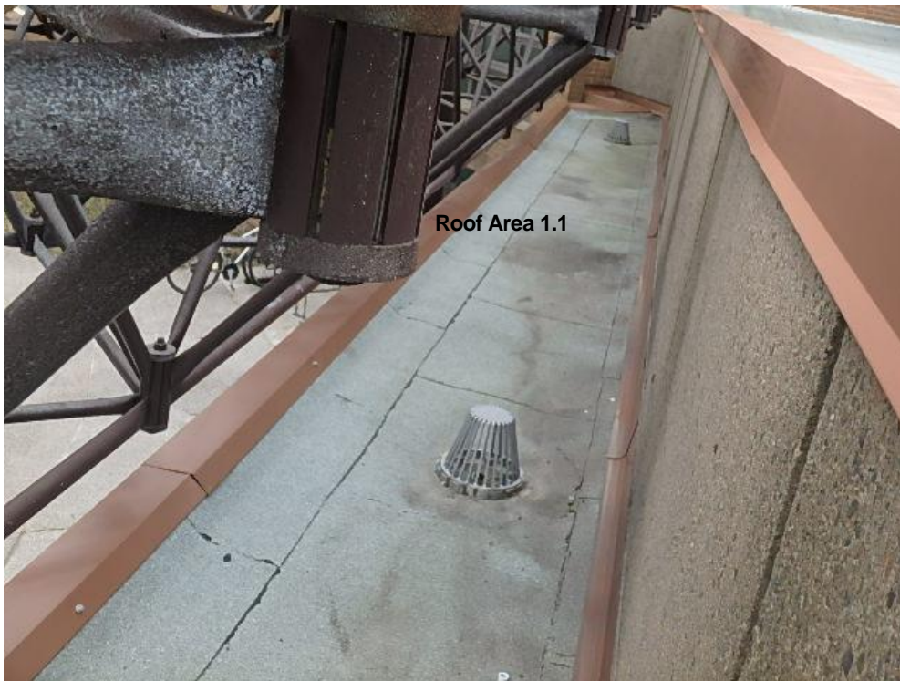
Photograph 2: Holland Building Roof Area 1.1 Ridging in membrane throughout roof area, and typical roof drains.
