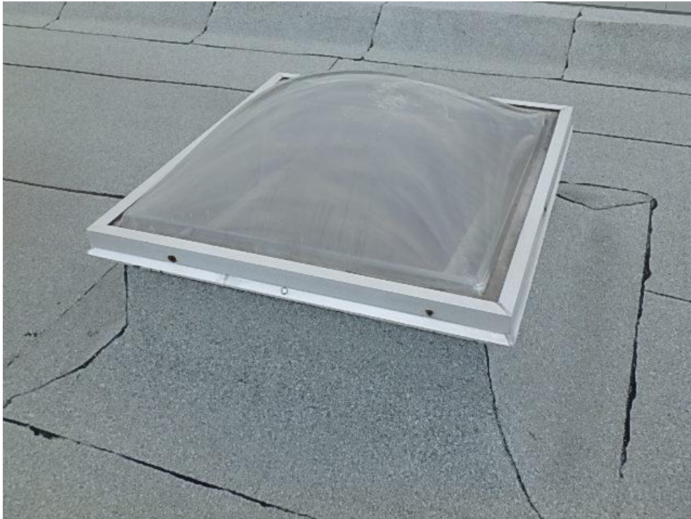
Photograph 51: Roof Area 3.1 – Skylight in good condition.
