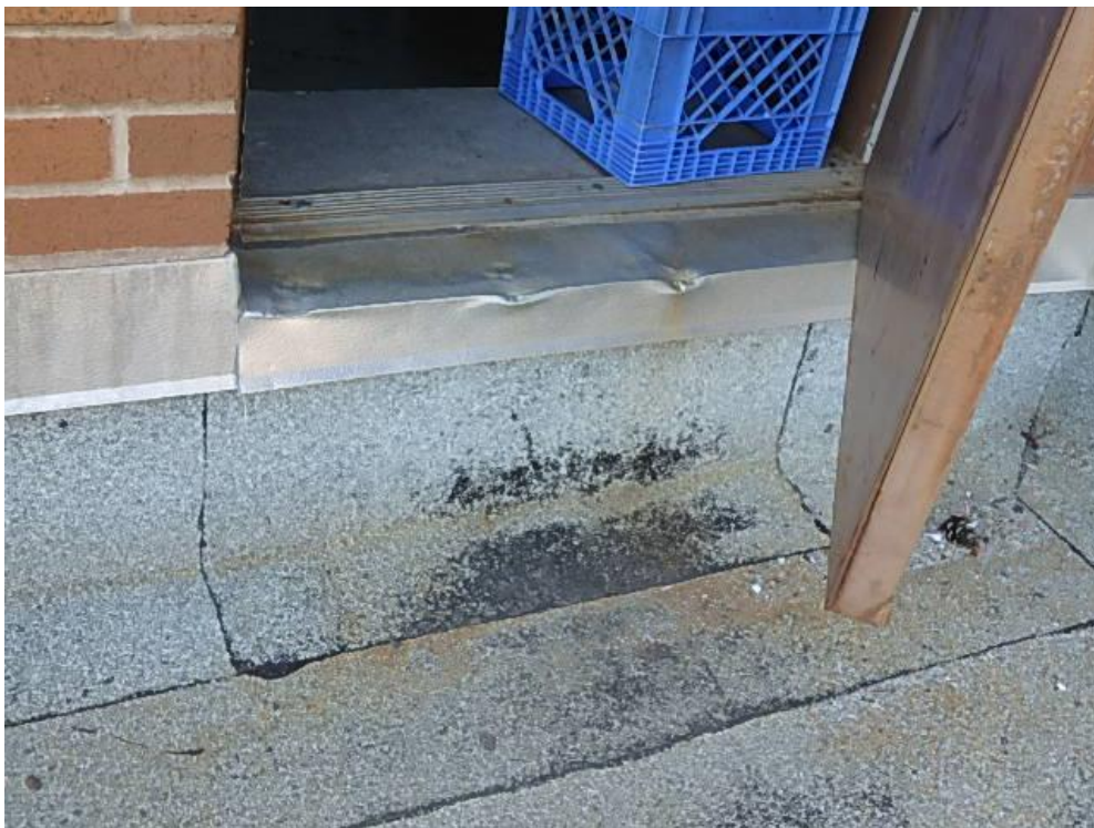
Photograph 20: Roof Area 2.1 –damaged metal flashing at doorway and worn membrane due to lack of membrane protection in front of door.
