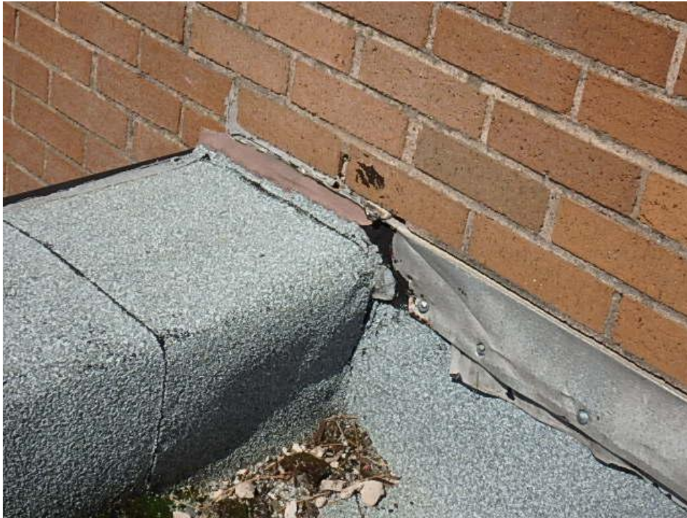
Photograph 41: Roof Area 2.3 – Parapet intersection at wall and reglet detail. Improperly sealed reglet over parapet.
