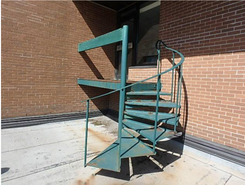
Photograph 15: Roof Area 1.1. Metal stairs and landing with rust staining of unprotected membrane below.
