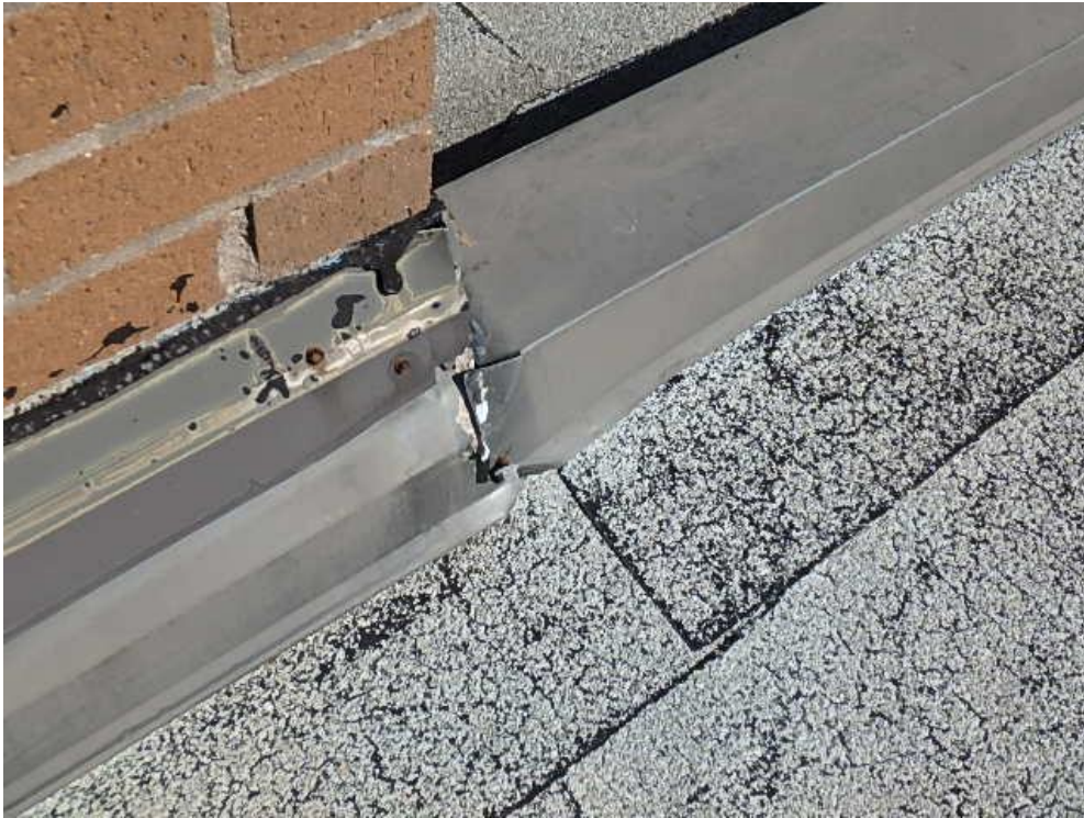
Photograph 17: Roof Area 1.1 – Cracked cap sheet flashing and damaged metal flashing.
