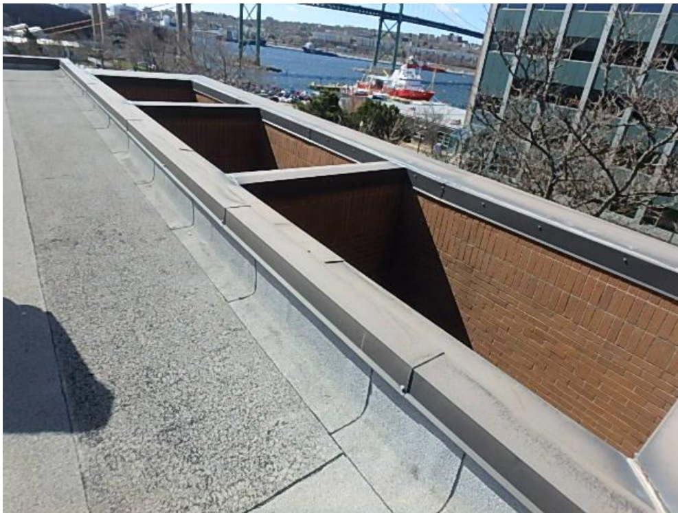
Photograph 8: Roof Area 1.1 – Typical parapet around open skylight.
