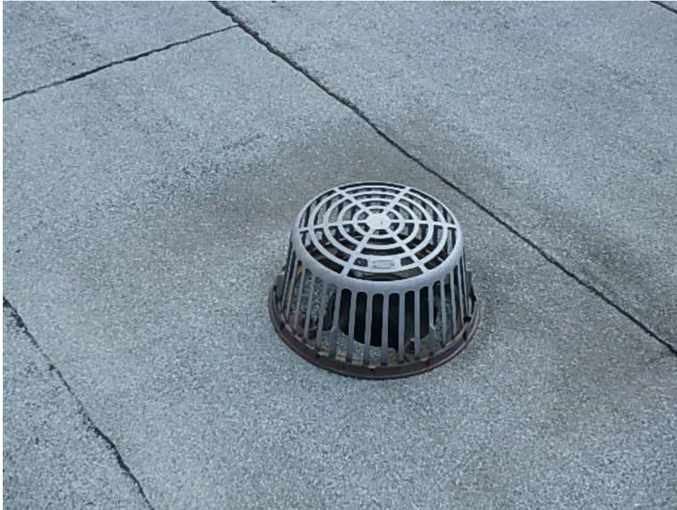
Photograph 11: Roof Area 1.1 – Typical roof drain installation with improper cap sheet detail.
