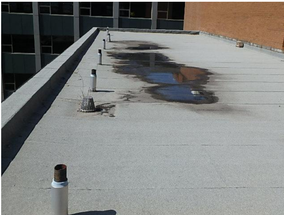
Photograph 38: Roof Area 2.3 – Showing typical, unprotected parapet membrane and ponding.
