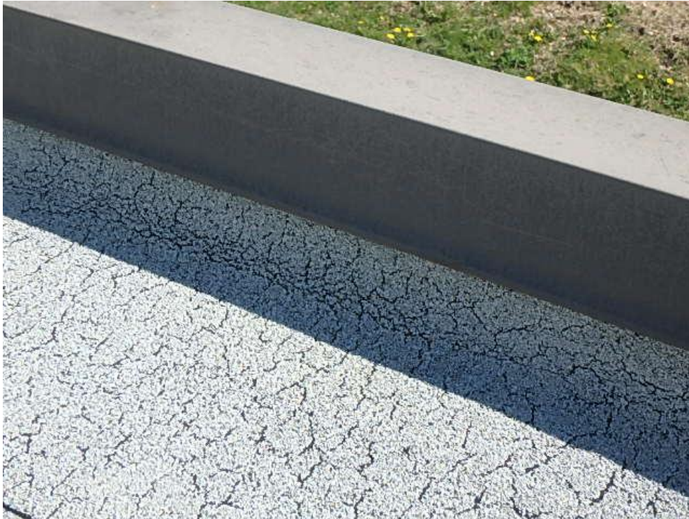
Photograph 13: Roof Area 1.1 – Typical cracking on cap sheet membrane along parapet.
