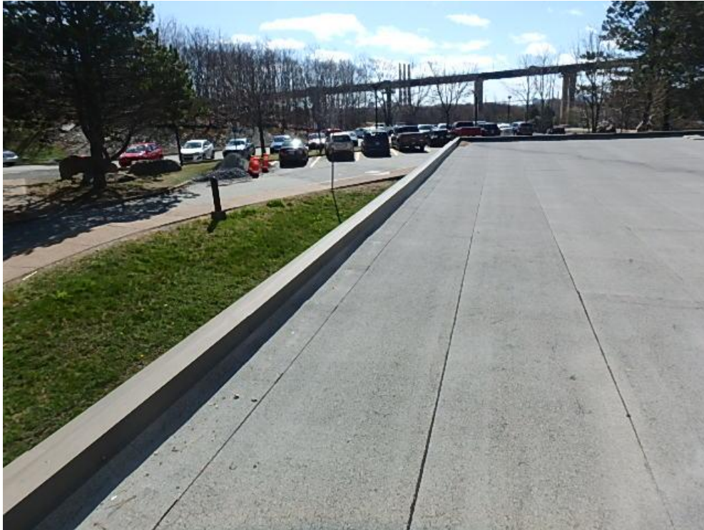
Photograph 3: Roof area 1.1 View of typical parapet along roof edge.
