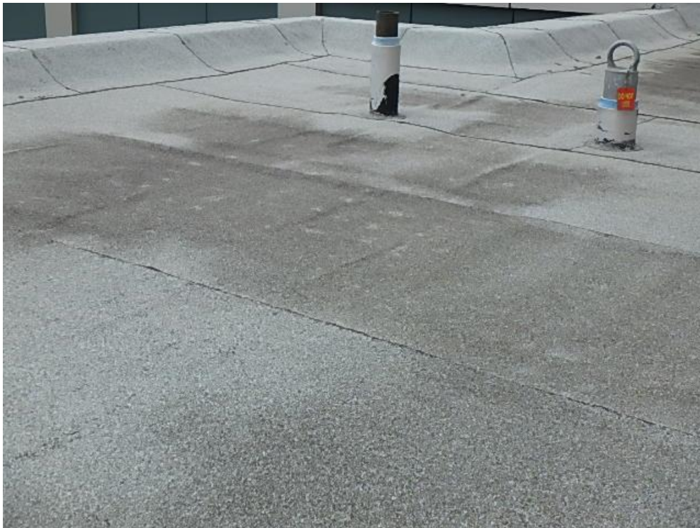
Photograph 64: Roof Area 3.3 – Evidence of ponding, ridging and blistering, and flashing problems around penetrations.
