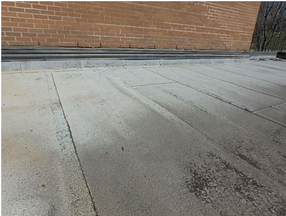
Photograph 14: Roof Area 1.1 – Ridging and blistering of roof membrane.
