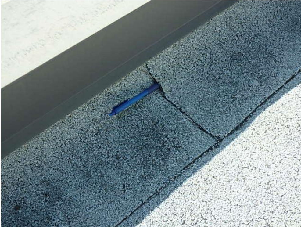
Photograph 9: Roof Area 1.1 – delamination of membrane cap sheet flashing that occurs in multiple locations along south east parapet.
