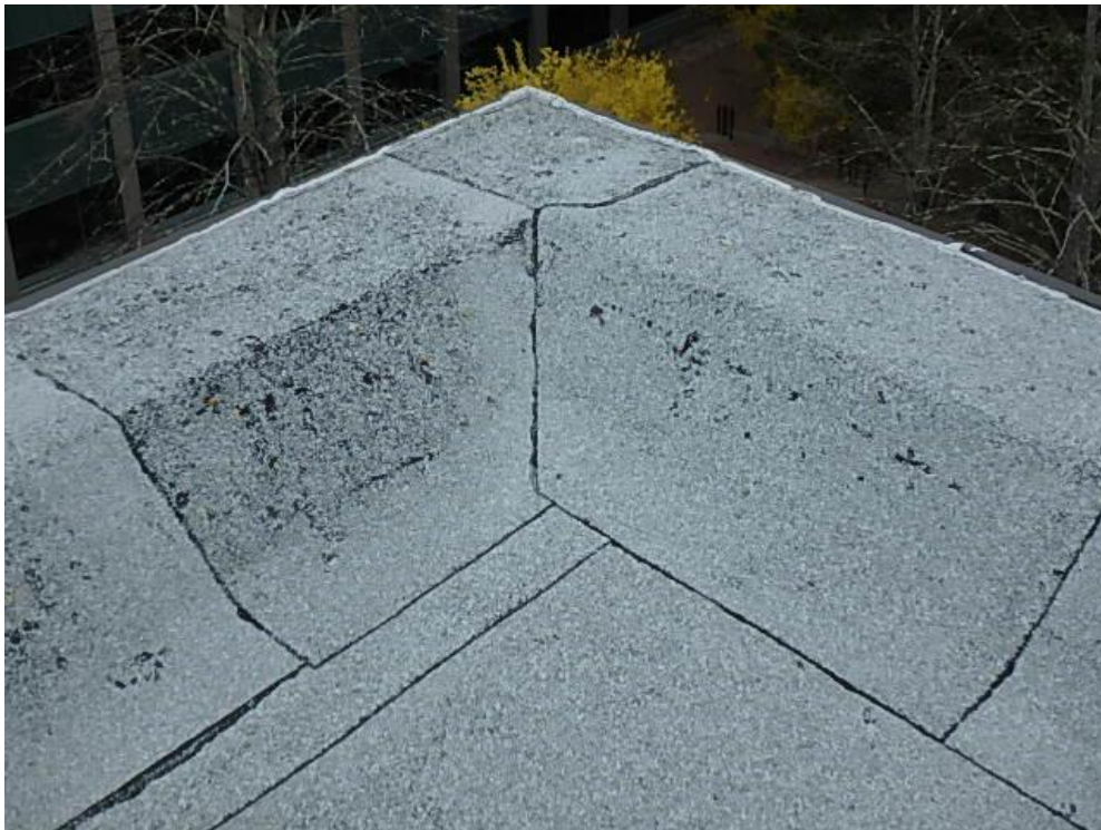
Photograph 58: Roof Area 3.2 – Blistering on membrane around roof edge and improper corner flashing detail.
