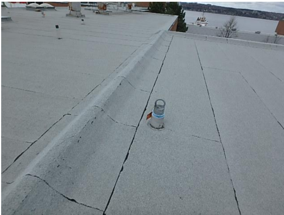
Photograph 52: Roof Area 3.1 – roof divider detail between roof area 3.1 & 3.2
