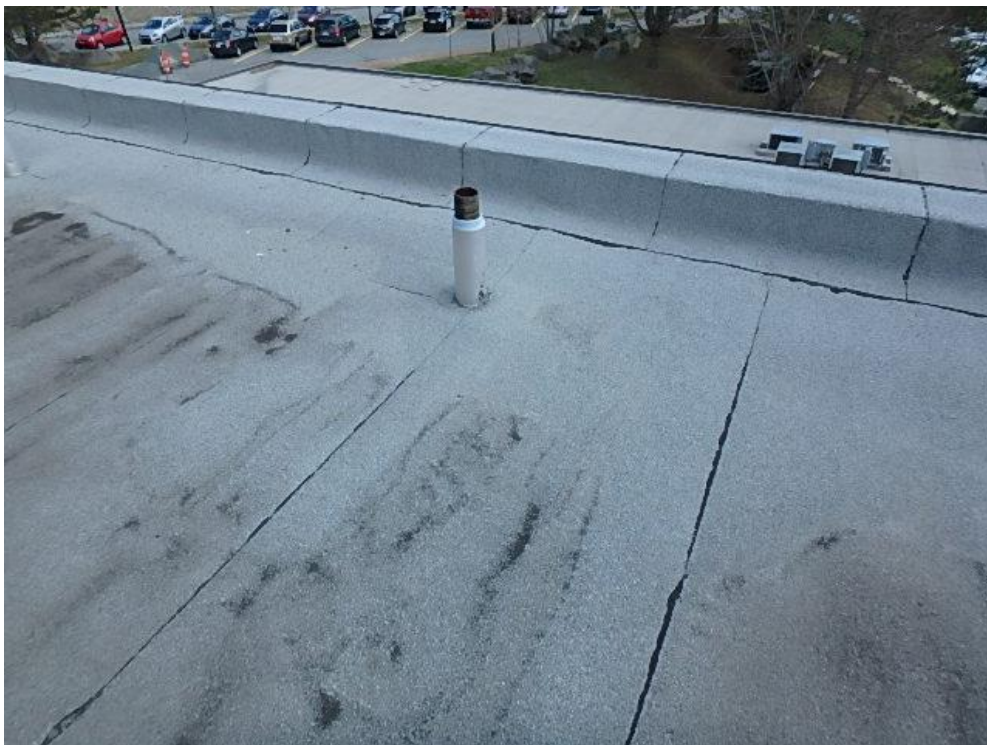
Photograph 22: Roof Area 2.1 – Ridging and blistering of roofing membrane and plumbing stacking penetration
