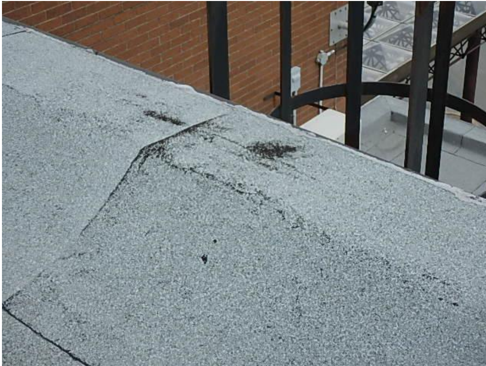
Photograph 53: Roof Area 3.1 – Top of ladder at roof edge without membrane protection.
