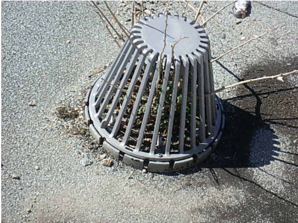
Photograph 39: Roof Area 2.3 – Roof drain blocked by vegetation growth.
