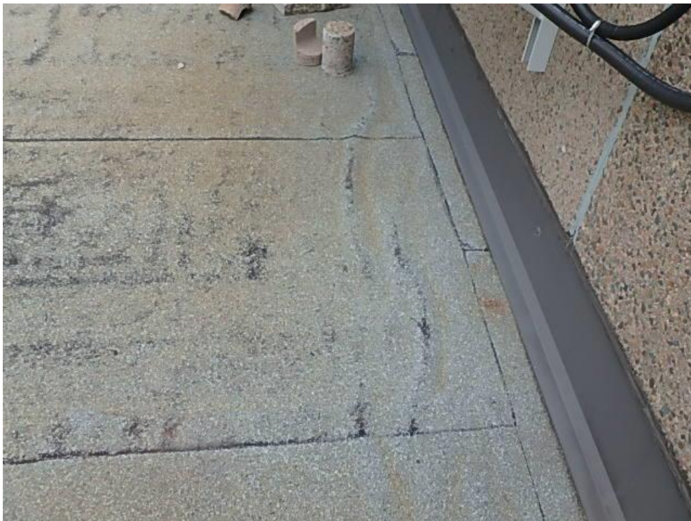
Photograph 10: Roof Area 2.1 – ridging in membrane between roof areas 3.1 and 3.2.
