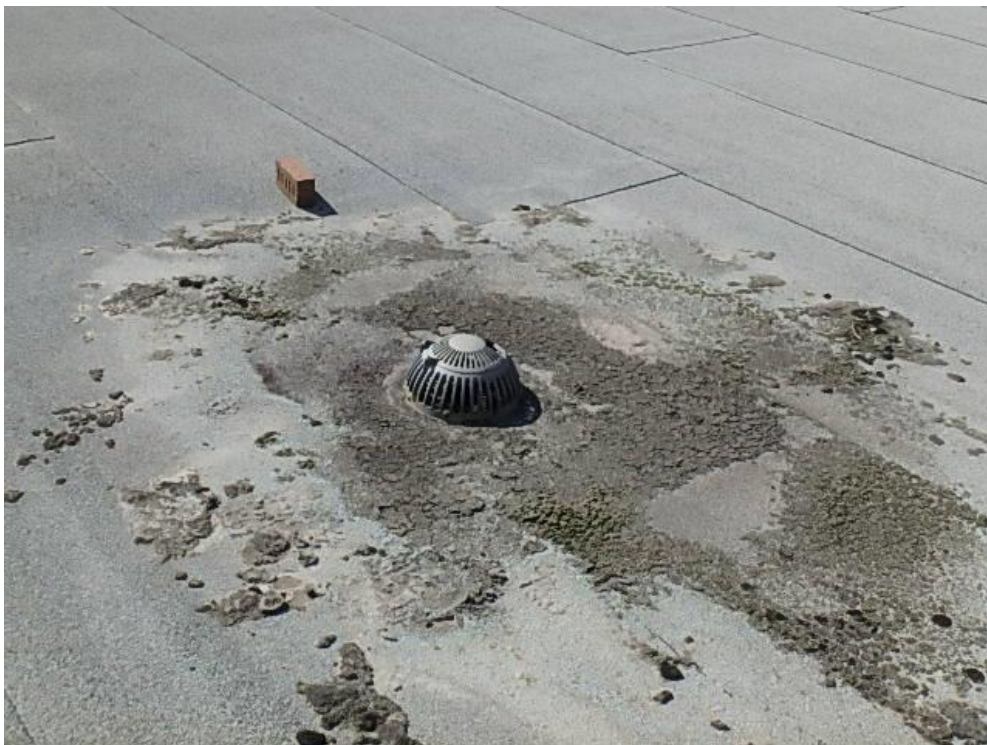
Photograph 4: Roof Area 1.1 – Roof drain with debris and severe blistering.
