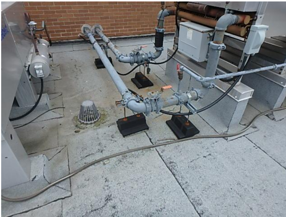
Photograph 32: Roof Area 2.2 – Membrane blistering, HVAC units on sleepers, roof drain with improper cap sheet detail and vegetation growth, and piping from HVAC unit through wall.
