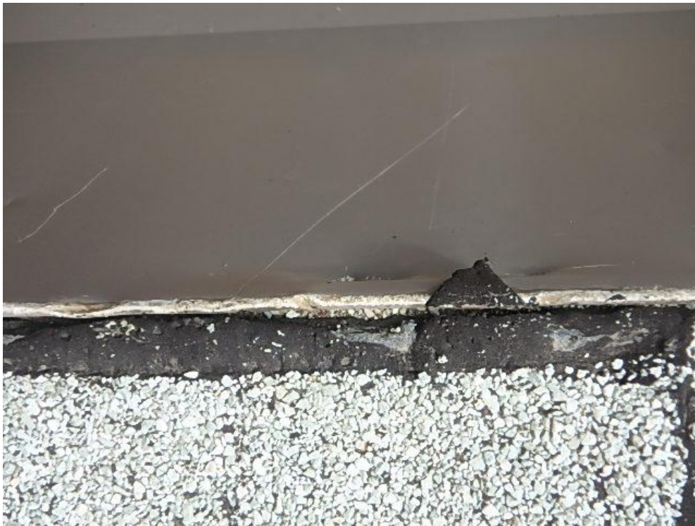
Photograph 20: Roof Area 2.1 – improper and poorly sealed roof edge detail at fascia.
