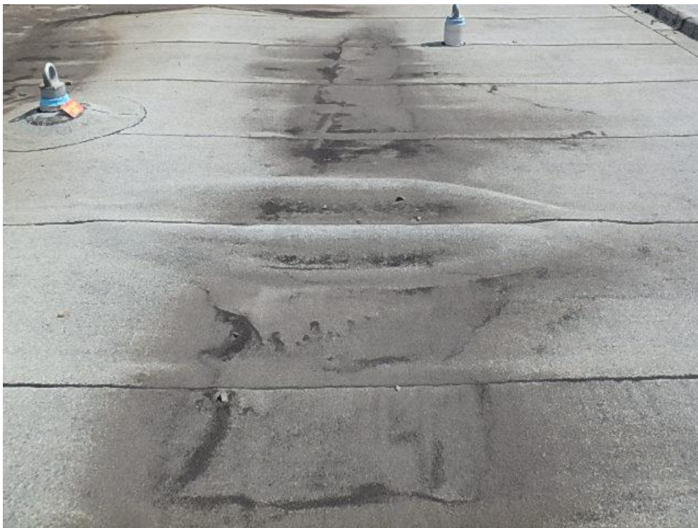
Photograph 26: Roof Area 3.1 – ridging, tenting and evidence of water ponding on membrane. Also shows unused roof anchor to be removed.
