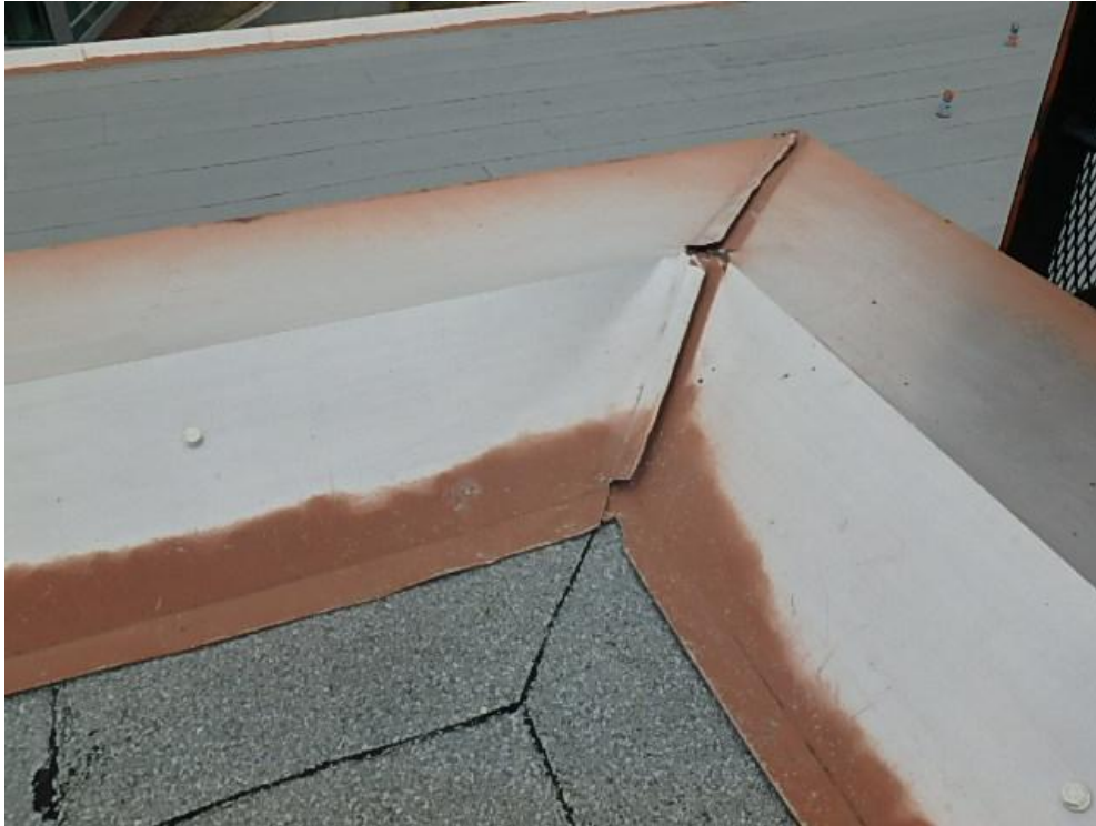
Photograph 29: Roof Area 3.3 – Corner of parapet flashing in poor condition and sealant is missing.
