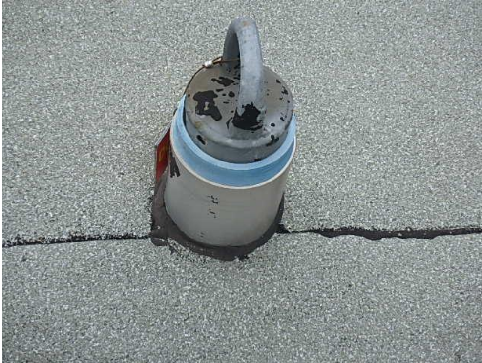
Photograph 7: Roof Area 2.1 – flashing problem at roof anchor that is not being used and should be removed.
