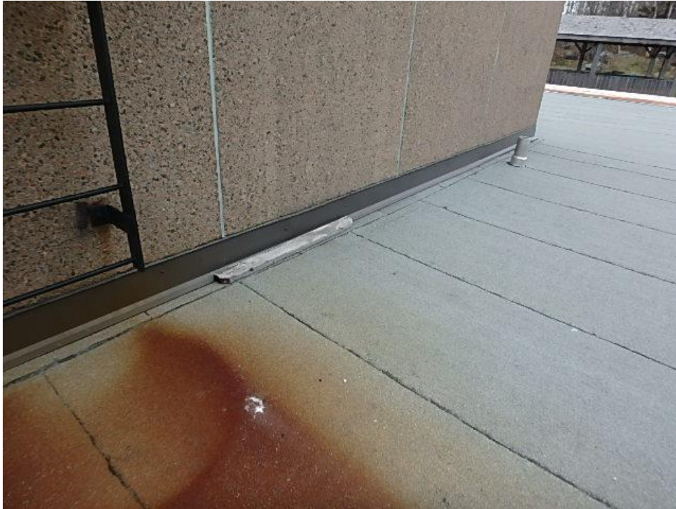
Photograph 11: Roof Area 2.1 – Rust staining of membrane from ladder and membrane protection missing under ladder.
