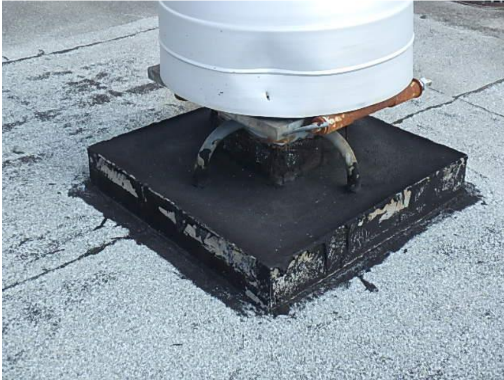
Photograph 13: Roof Area 1.1 – Exhaust fan penetration with improperly sealed conduit and fan penetrations and worn out sealant around base pan.
