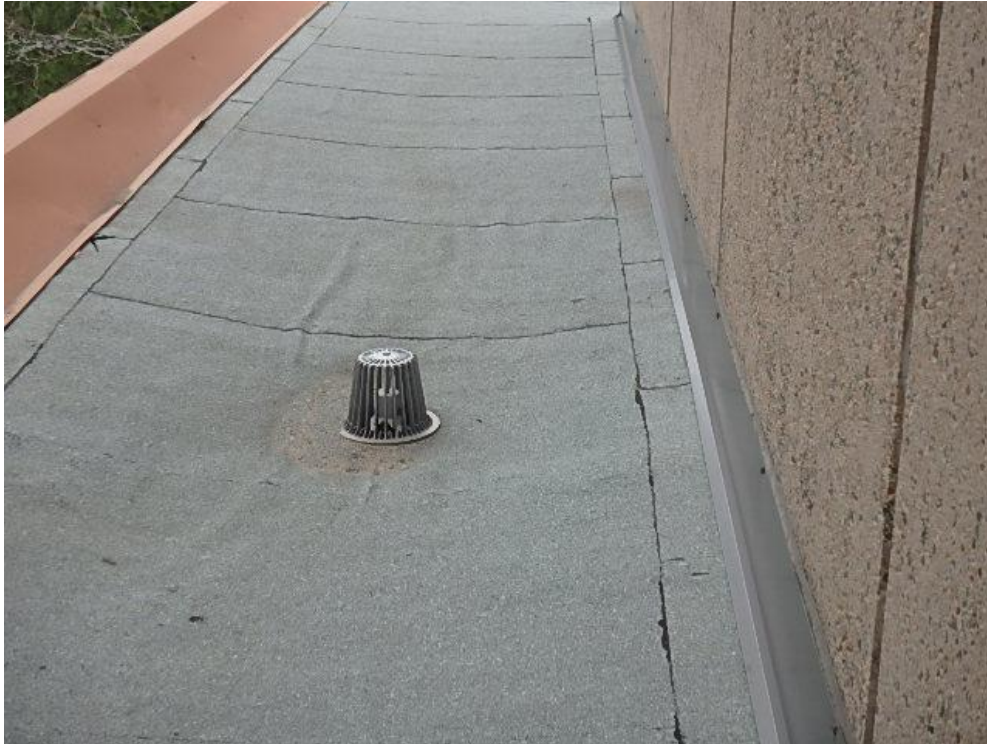
Photograph 5: Roof Area 1.2 – substantial ridging in membrane and typical roof drain
