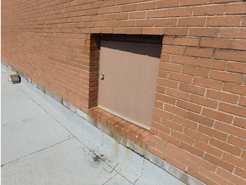
Photograph 43 - Roof Area 2.3 – Staining of membrane and flashing under sill of access door.
