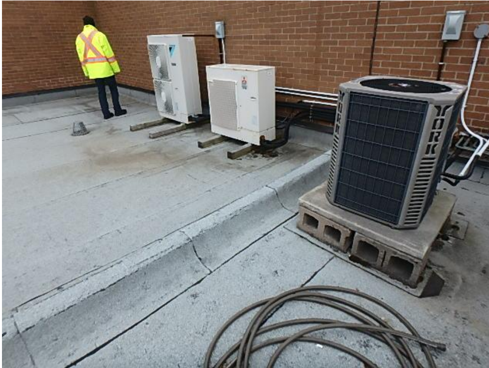
Photograph 33: Roof Area 2.2—HVAC units on sleepers with no membrane protection and AC units on paver/concrete blocks also without membrane protection.
