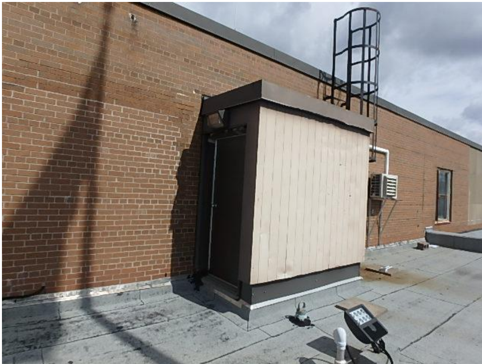
Photograph 14: Roof Area 2.1 – Door to roof area 1.1 with worn membrane due to lack of membrane protection outside of doorway.
