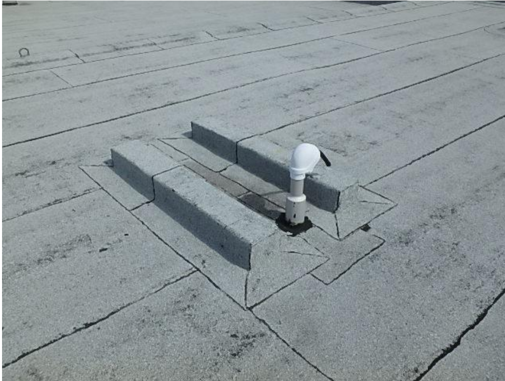
Photograph 7: Roof Area 1.1 – unused sleepers and unused conduit gooseneck with worn out sealant around its base.
