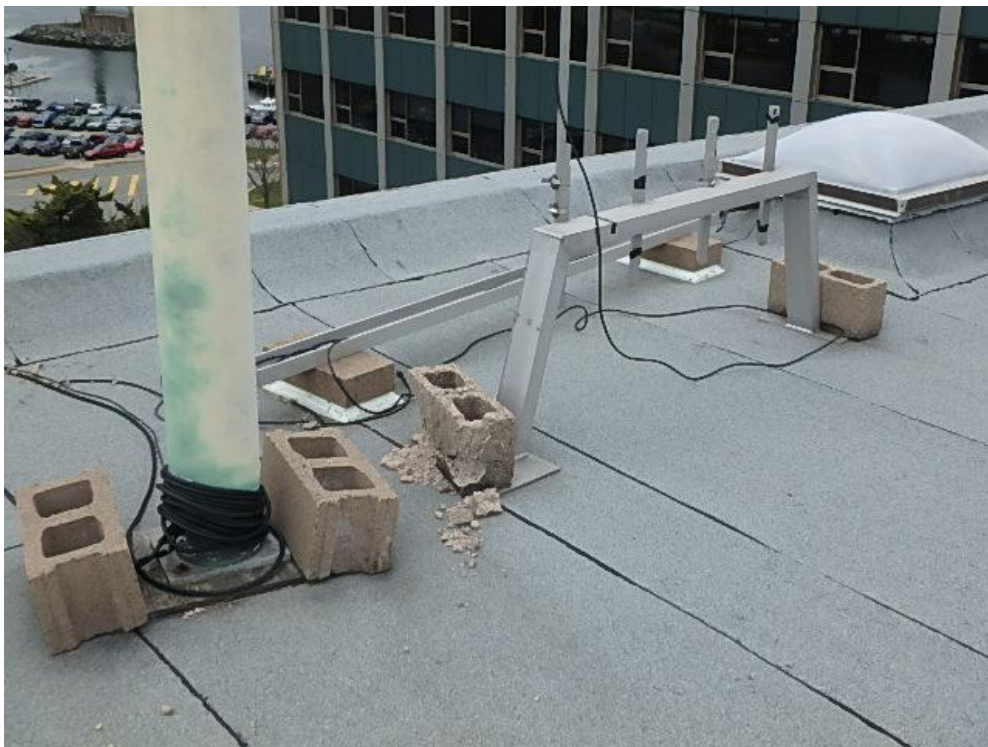
Photograph 62: Roof Area 3.3 –Debris and lack of membrane protection under metal supports and concrete blocks. Improper column support used.
