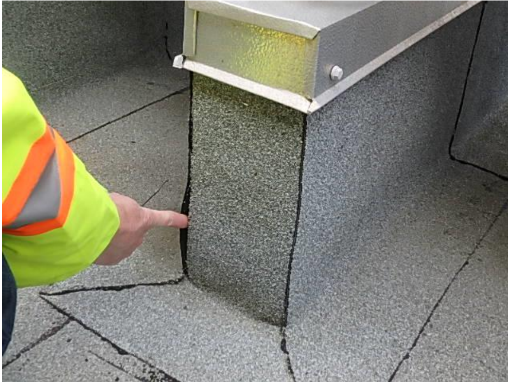
Photograph 31: Roof Area 2.2– Typical membrane delamination around HVAC sleeper.
