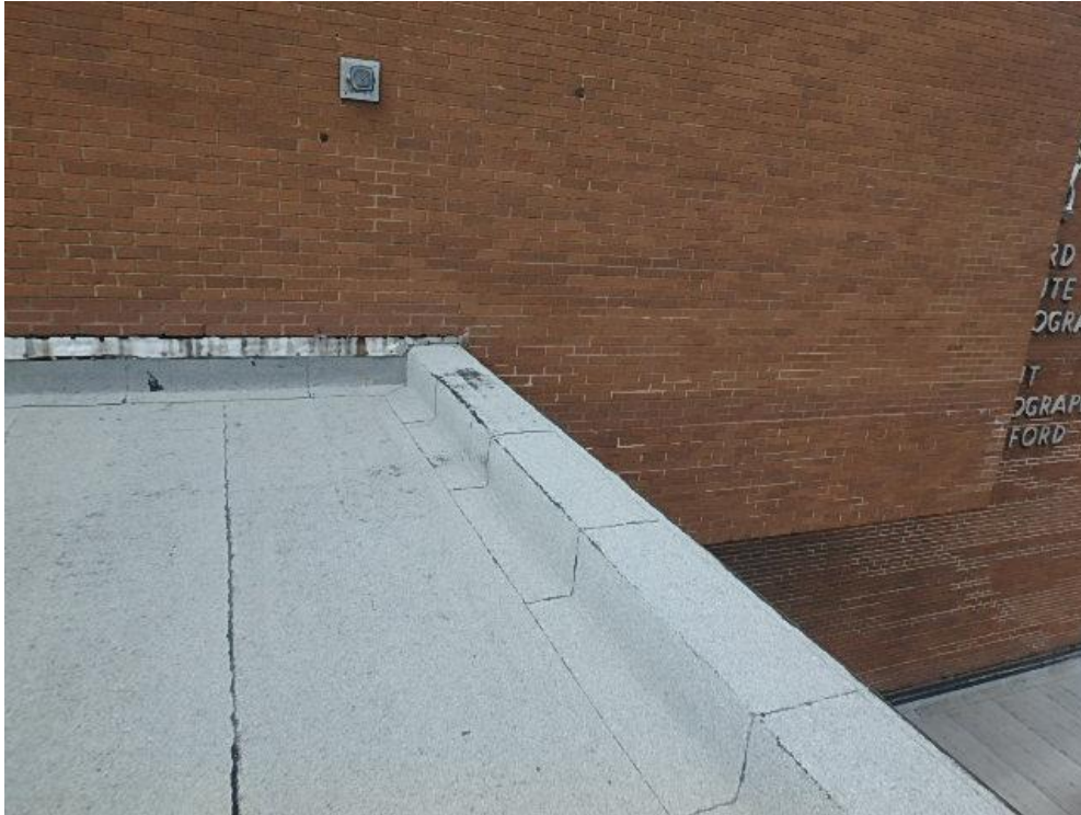
Photograph 23: Roof Area 2.1 – Typical unprotected parapet with worn edges.
