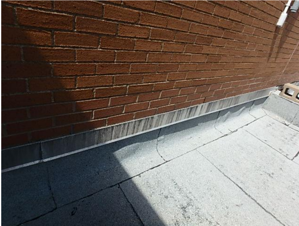
Photograph 21: Roof Area 2.1 – Membrane tenting at reglet detail along wall.
