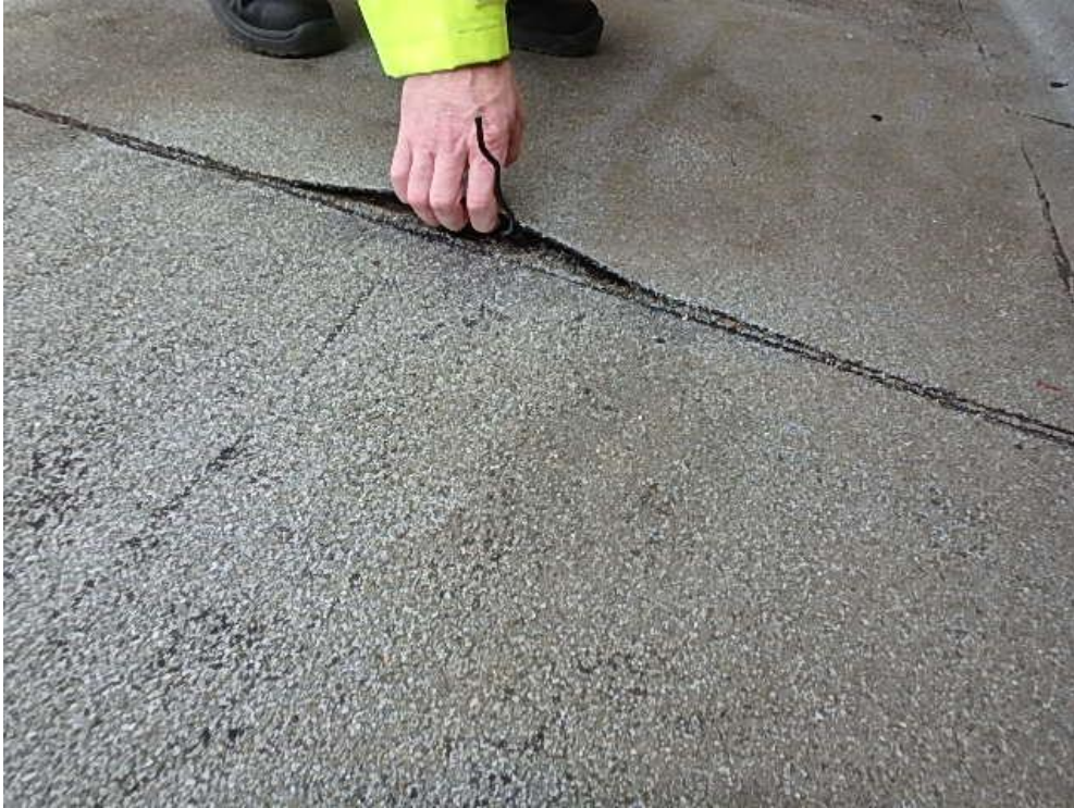
Photograph 35: Roof Area 2.2 – Membrane delamination along seam.
