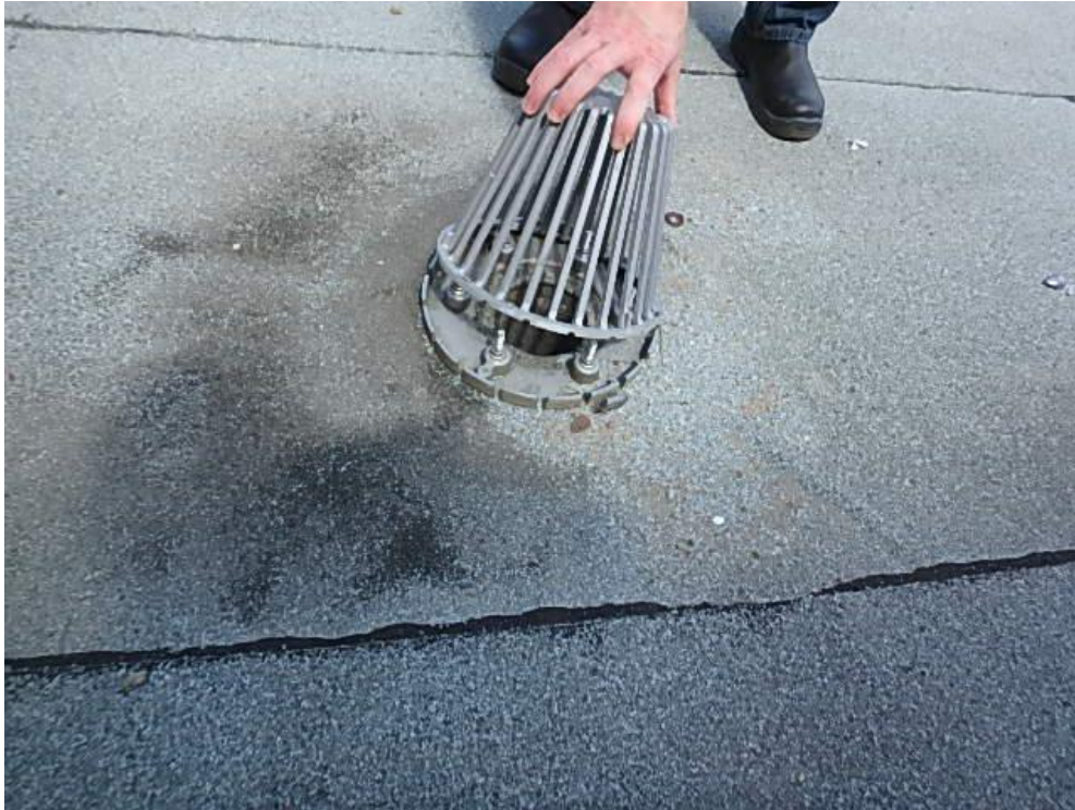
Photograph 19: Roof Area 2.1 – Roof drain with surrounding blisters and improper cap sheet detail around drain.
