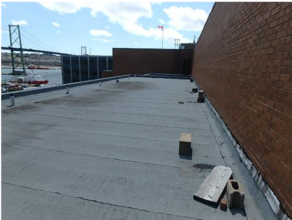
Photograph 26: Roof Area 2.1 – Overall view facing south west showing debris along wall, poorly sealed reglet detail, and ridging and blistering on roofing membrane.
