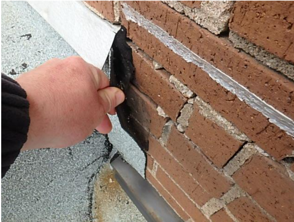
Photograph 65: Roof Area 3.3 – Separation of membrane flashing from wall. Poor flashing detail at intersection of reglet at parapet.
