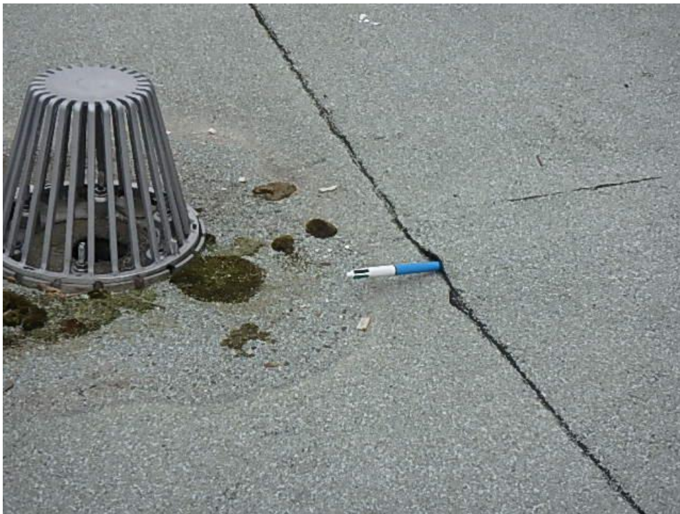
Photograph 8: Roof Area 2.1 – Roof drain without proper membrane cap flashing (typical throughout roof area) and vegetation growth. Also shows debonding of cap sheet membrane.
