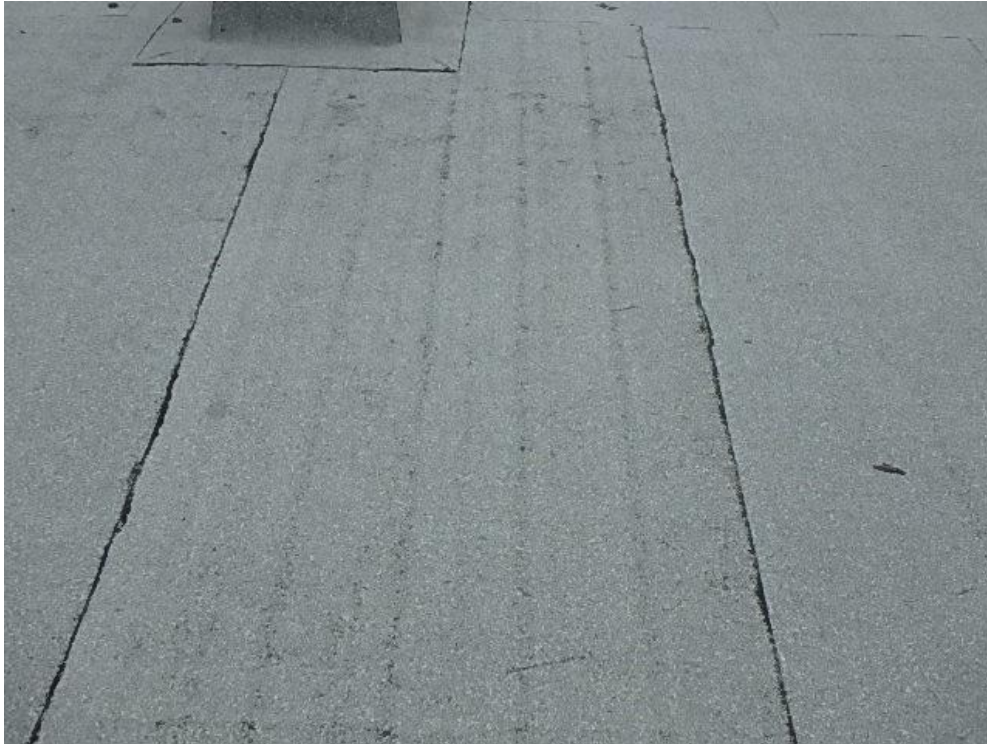
Photograph 9: Roof Area 2.1 – Ridging in membrane
