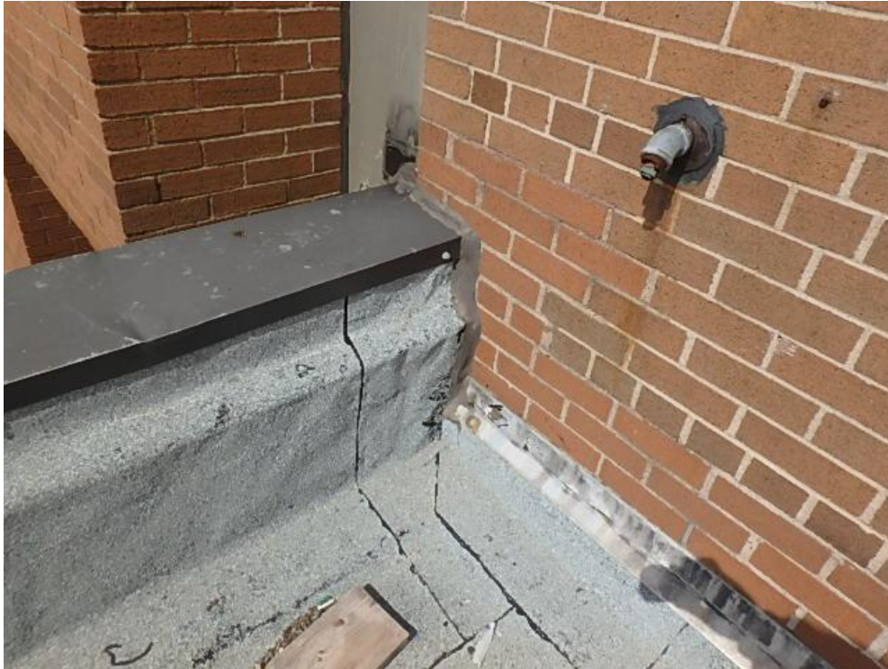
Photograph 15: Roof Area 1.1. Corner of roof area at adjacent wall showing worn, and tented flashing, sealant between parapet and wall, and reglet detail at wall. Both wall transitions are poorly sealed.
