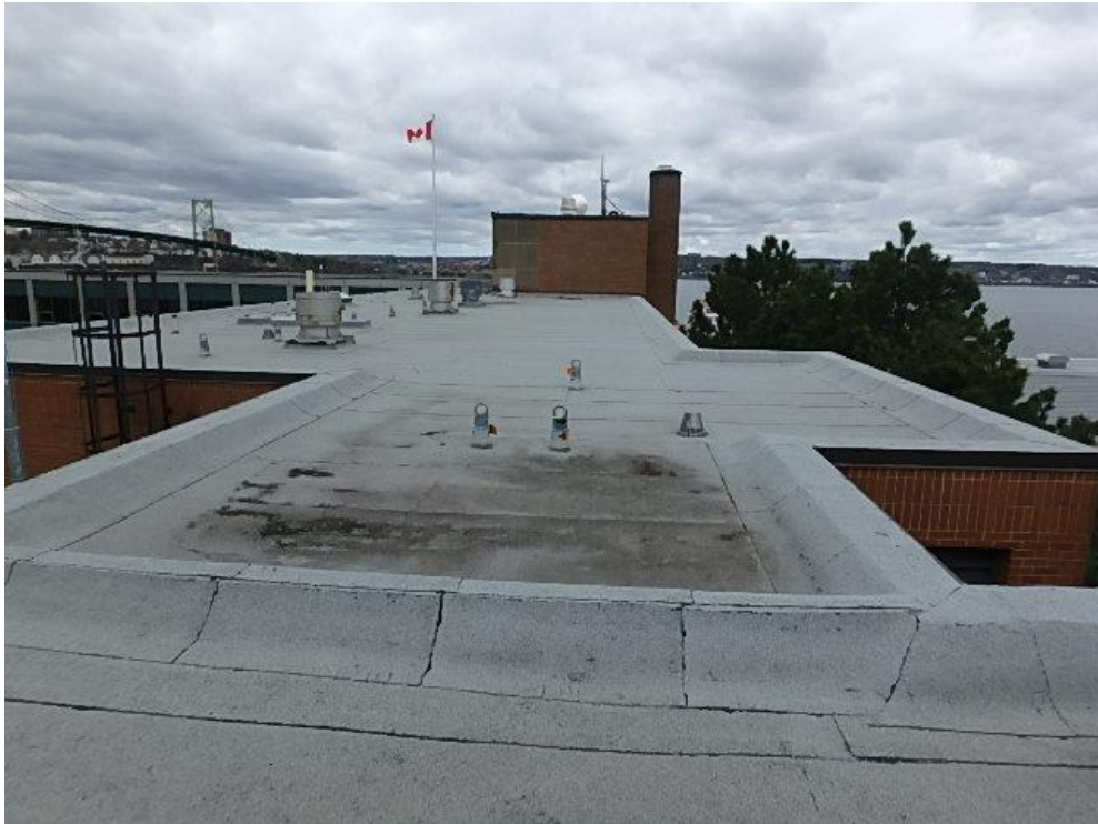
Photograph 59: Roof Area 3.3 – Overall view of roof area 3.3 with evidence of ponding along with ridging and blistering of membrane.
