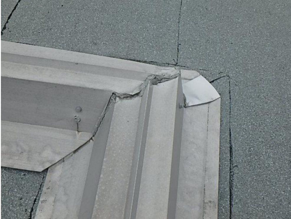
Photograph 17: Roof Area 2.1 – poor sealant adhesion at intersection in expansion joint
