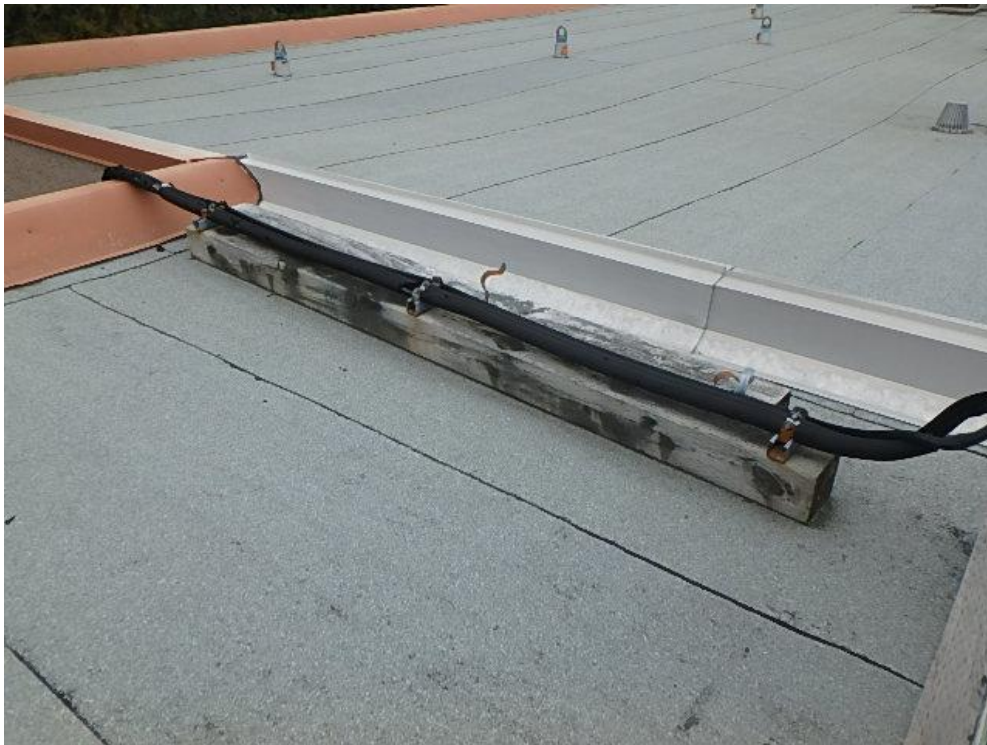
Photograph 14: Roof Area 2.1 – Conduit over parapet and wood sleeper without proper membrane protection.
