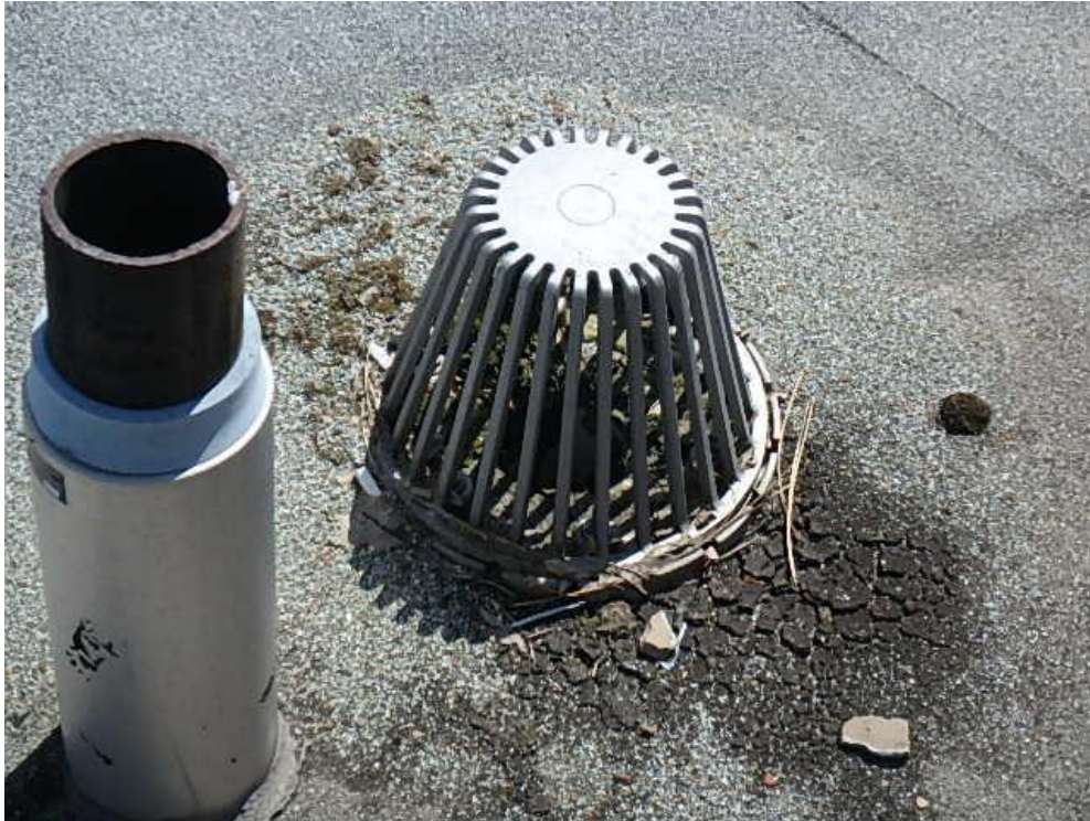
Photograph 27: Roof Area 2.1 – drain and plumbing stack detail with improper cap sheet membrane detail around drain, poorly sealed plumbing stack, cracking in membrane and vegetation growth.
