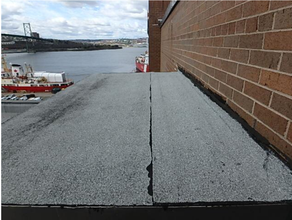
Photograph 19: Roof Area 2.1 – Overall view of roof area 2.1 over doorway to roof area 2.1 with improper drip edge, and reglet detail with poor seal to adjacent wall.
