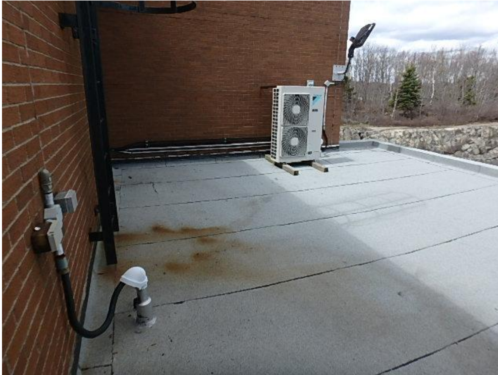
Photograph 29: Roof Area 2.2– Rust staining of unprotected membrane under ladder, HVAC on sleepers without membrane protection, and conduit gooseneck penetration.
