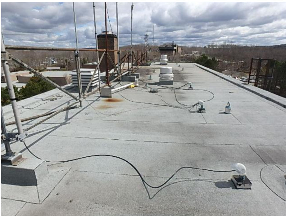
Photograph 24: Roof Area 3.1 – Overall view of roof area facing north east. Also showing metal truss supporting antennae, sleeper truss supports, and conduit goosenecks along with exhaust fans, drains, and roof anchors.
