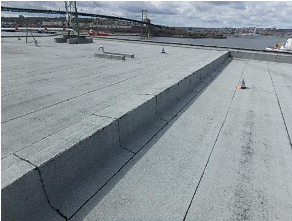
Photograph 4: Roof Area 1.1 – roof divider between two parts of 1.1 that is not protected by metal flashing. Also shows roof anchors that are not in use and should be removed.
