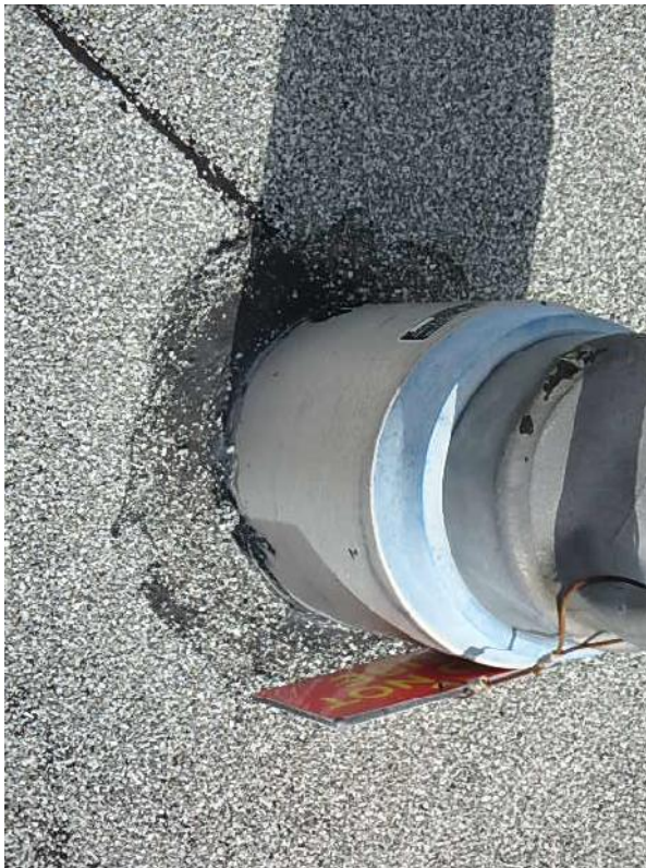
Photograph 48: Roof Area 3.1 – Typical roof anchor to be removed due to load testing failure. Poor flashing around anchor base is also typical.
