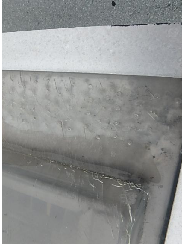
Photograph 27: Roof Area 3.2 –Damaged skylight.
