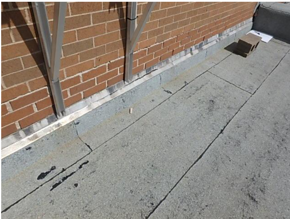
Photograph 16: Roof Area 1.1 – Ladder to roof area 3.1 showing no membrane protection at bottom, bleed out at seams, and wearing of membrane.
