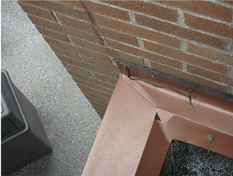
Photograph 3: Roof Area 1.2 – Damaged flashing at reglet.
