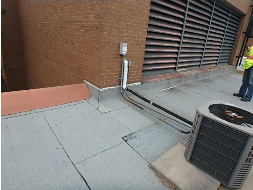
Photograph 21: Roof Area 2.2 – Showing conduit penetration into wall, wall louvre with water staining on membrane and air conditioner on pavers with cap sheet as membrane protection.
