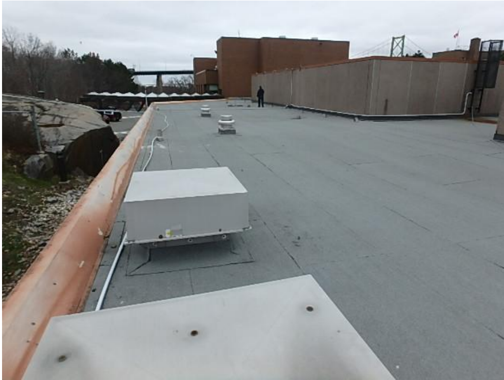
Photograph 19: Roof Area 2.1 – Overall view of roof area 2.1 on north side facing east showing unused roof curbs, conduit, exhaust fans and typical parapet flashing.
