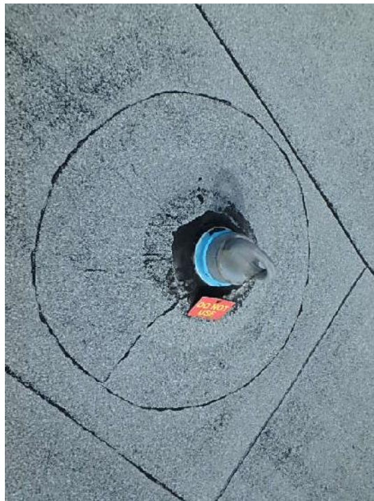
Photograph 8: Roof Area 1.1 – Existing roof anchor that is not in use and should be removed.
