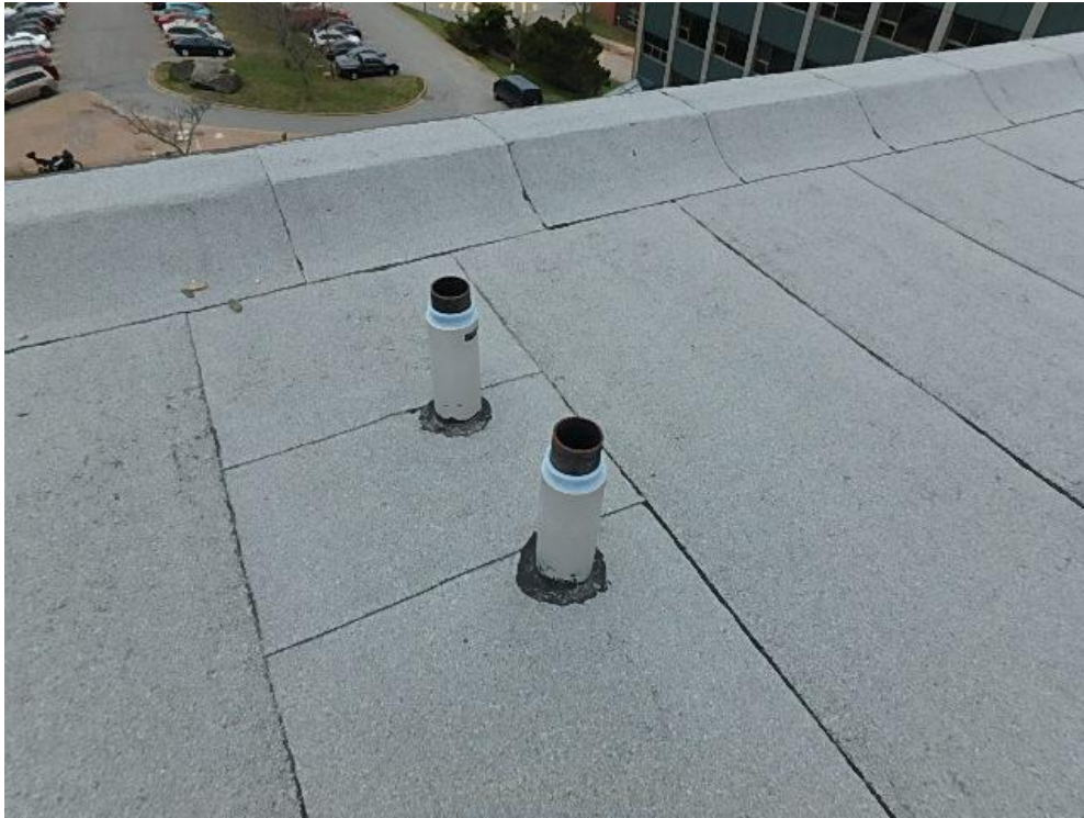
Photograph 61: Roof Area 3.3 – Flashing problem around plumbing stacks.
