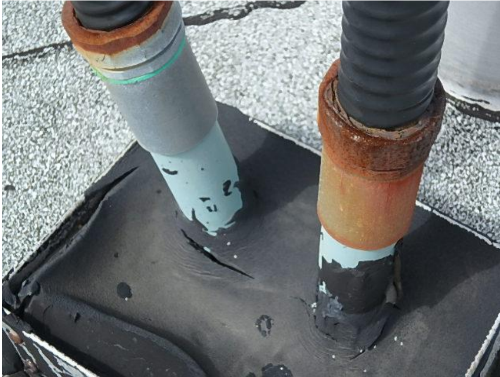
Photograph 5: Roof Area 1.1 – Improperly sealed and cracked pitch pan with improperly sealed conduit penetrations.
