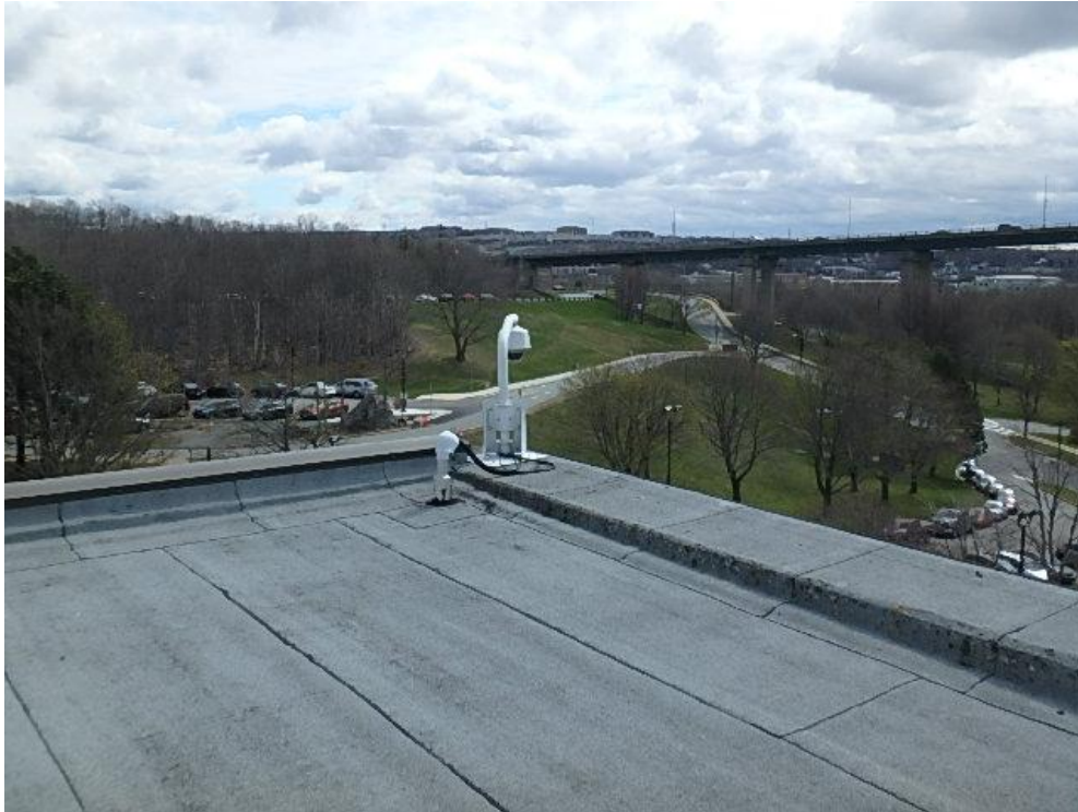
Photograph 9: Roof Area 1.1 – View of the east corner showing two different parapet conditions along with security camera and conduit gooseneck penetration with worn sealant.
