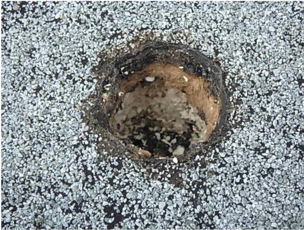
Photograph 77: Murray Building roof area 3.3 Core cut
