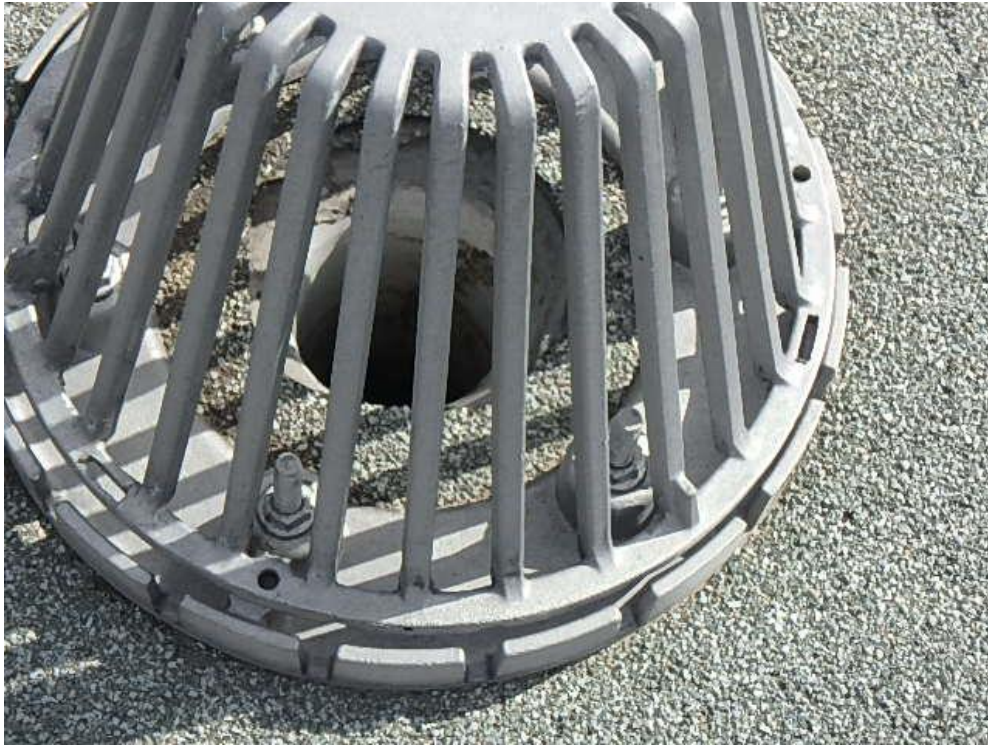
Photograph 49: Roof Area 3.1 – Typical roof drain installation with improper cap flashing detail.
