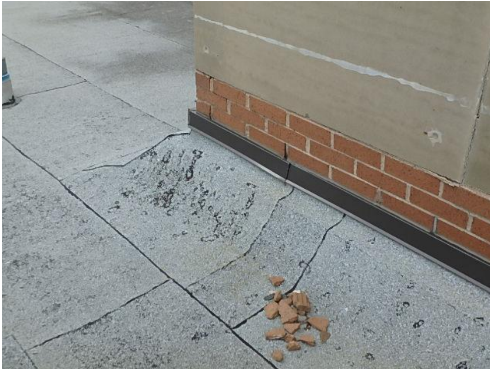
Photograph 63: Roof Area 3.3 – Blistering on membrane along with minor debris.
