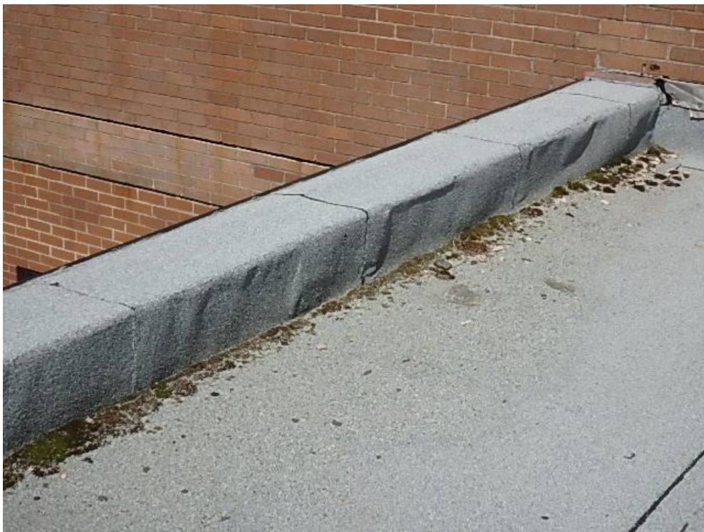
Photograph 40: Roof Area 2.3 – Parapet with membrane tenting and vegetation growth.
