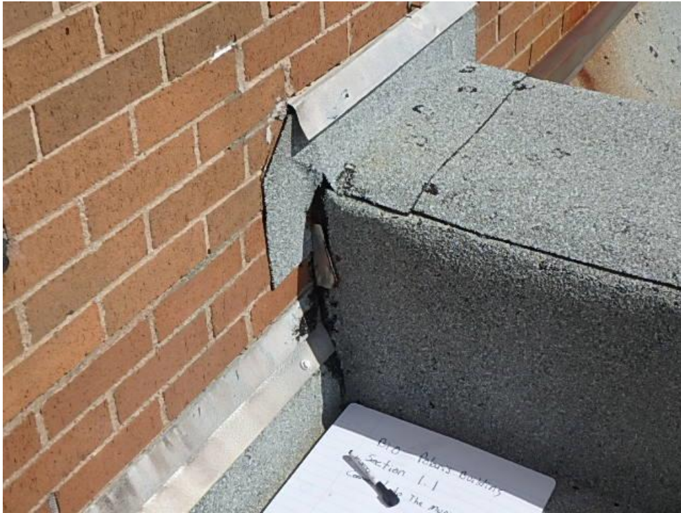
Photograph 17: Roof Area 1.1 – roof divider between Polaris and Murray building with improper reglet detail at intersection of divider and wall.
