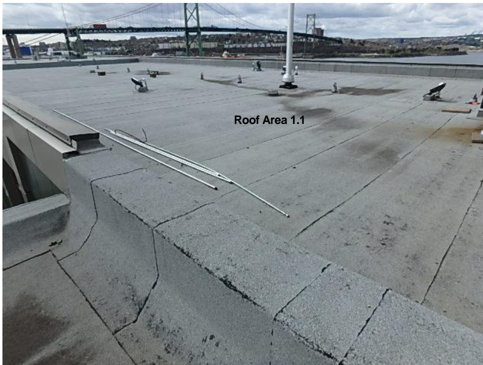
Photograph 2: Overall view of Polaris building Roof Area 1.1 looking south towards Halifax. This is a 2 ply modified bitumen roof that is approximately 12 years old
