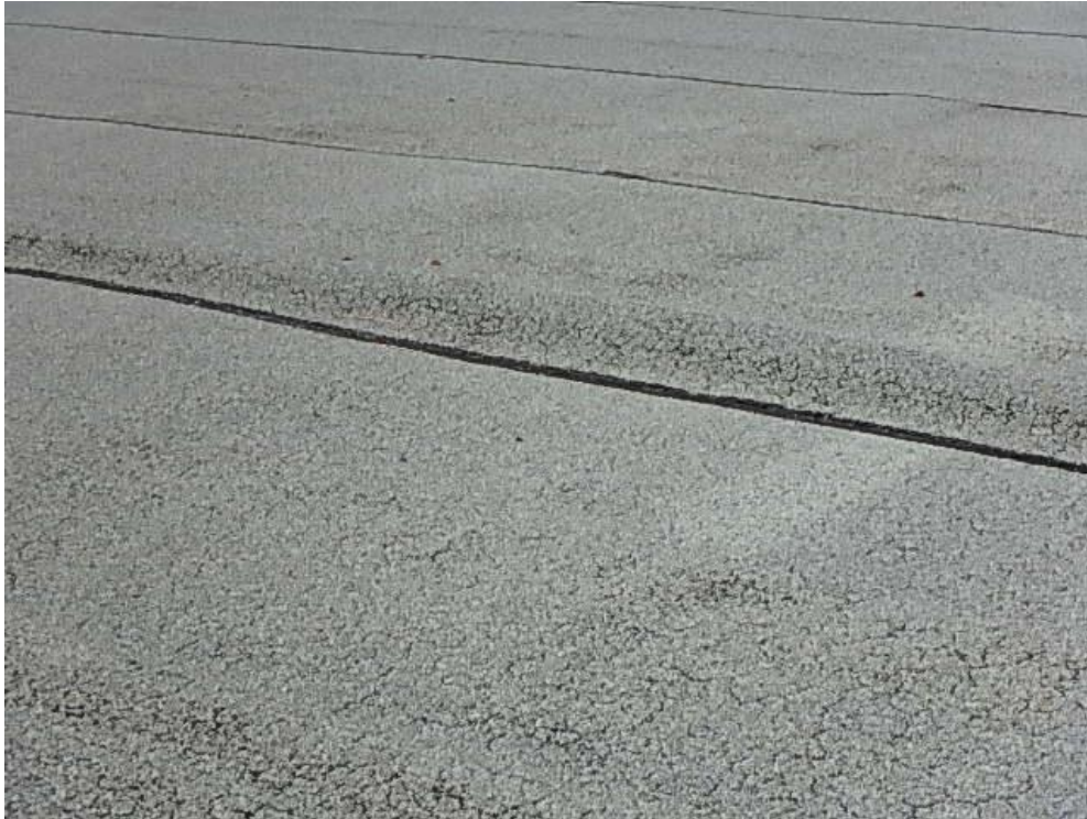
Photograph 5: Roof Area 1.1 – Ridging of membrane at seam.
