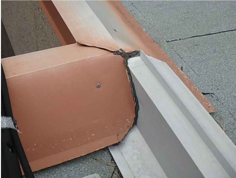
Photograph 13: Roof Area 2.1 – poor adhesion of flashings at intersection of parapet and expansion joint.
