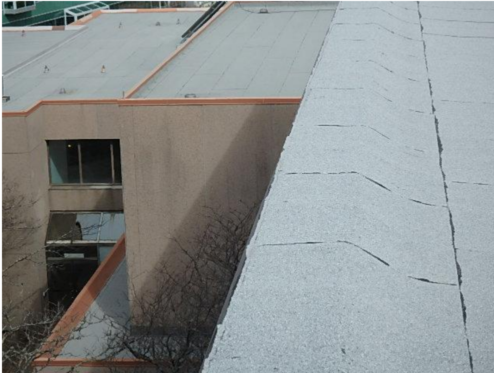
Photograph 47: Roof Area 3.1 – Typical gravel stop along roof edge.
