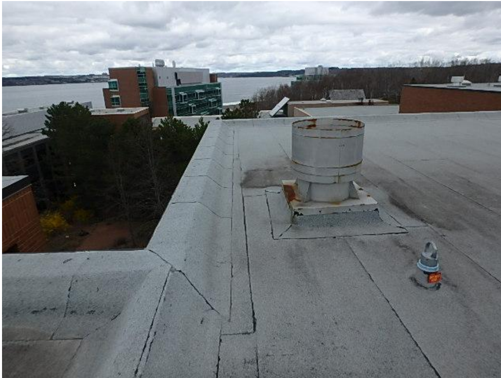
Photograph 57: Roof Area 3.2 – Evidence of ponding around exhaust fan curb. Membrane flashing problems also evident around curb.
