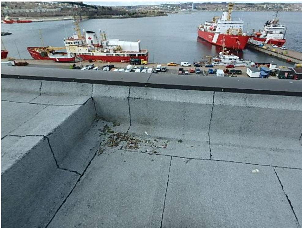
Photograph 10: Roof Area 1.1 – Roof divider condition at perimeter showing minor debris build up. Majority of perimeters are not protected by metal flashing.
