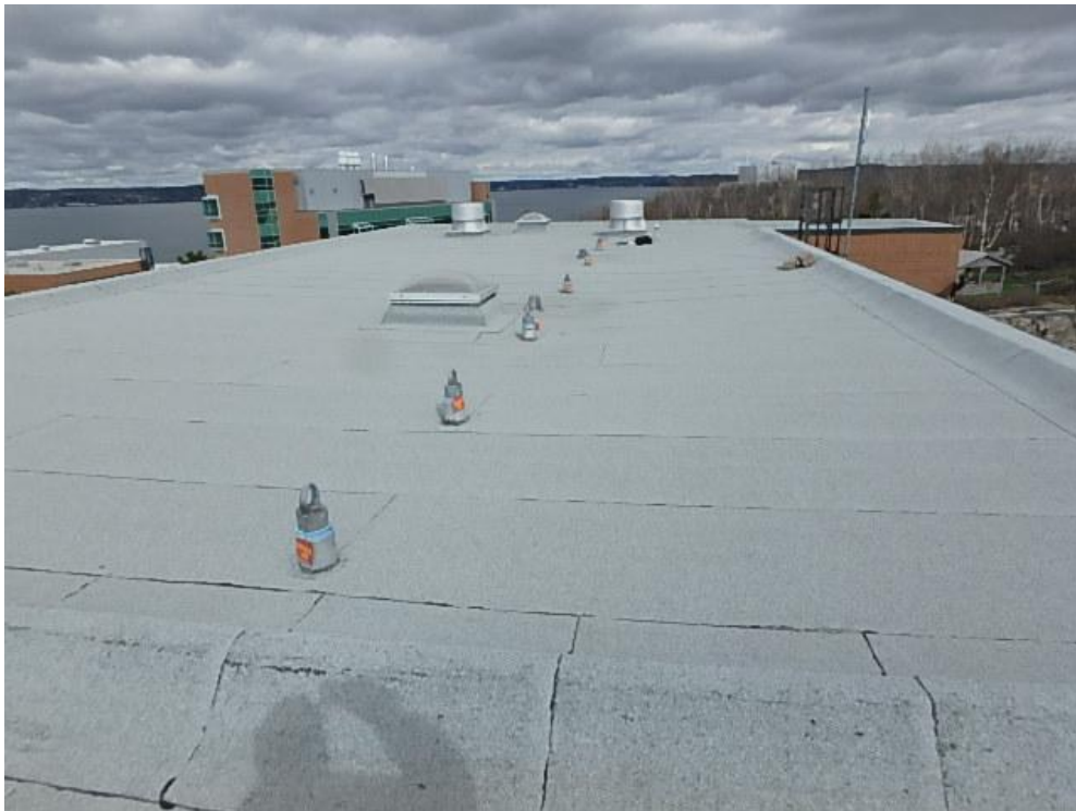
Photograph 46: Roof Area 3.1 – Overall view of roof area facing north west. The modified bitumen roof is approximately 12 years old.
