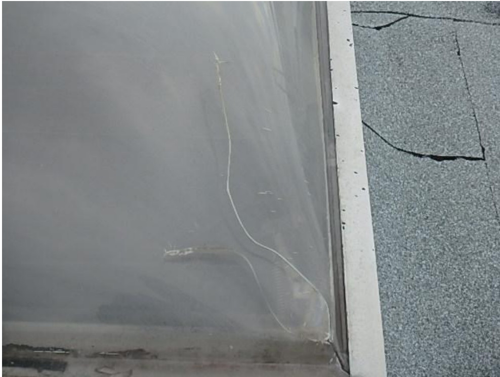
Photograph 55: Roof Area 3.1 – Damaged skylight.
