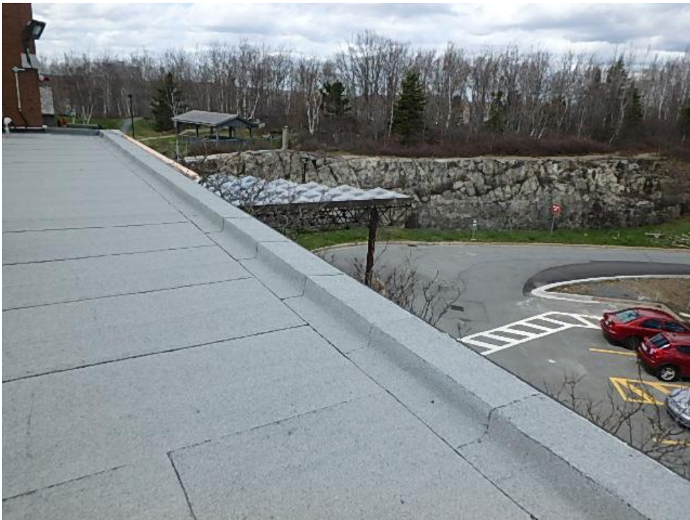
Photograph 36: Roof Area 2.2 – Typical parapet detail around roof edge.
