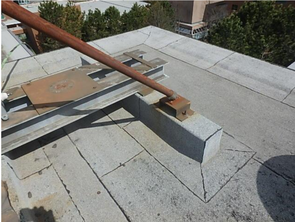
Photograph 27: Roof Area 3.1 –Truss support sleeper with connector screwed directly through membrane (improperly sealed), and typical roof edge detail.
