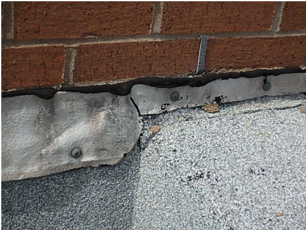
Photograph 24: Roof Area 2.1 – Damaged and poorly sealed flashing along wall at reglet and parapet intersection.
