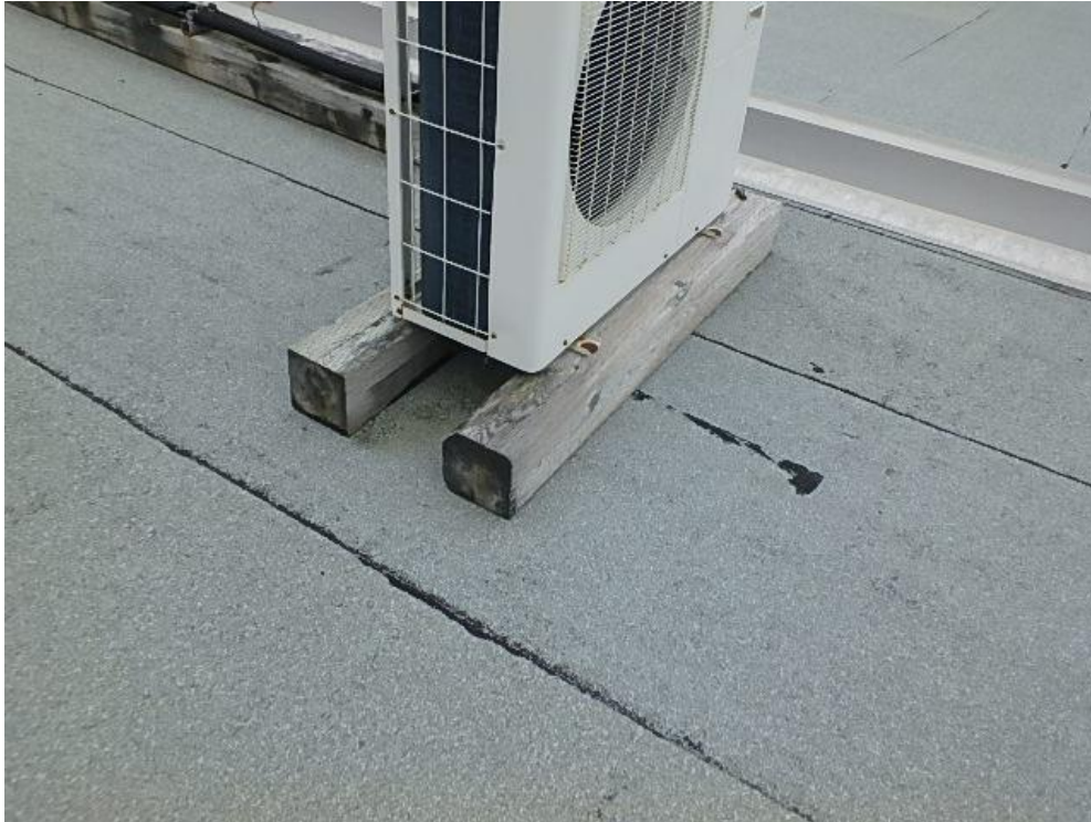
Photograph 15: Roof Area 2.1. Small HVAC unit on wood sleepers without proper membrane protection.
