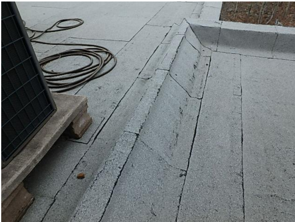
Photograph 34: Roof Area 2.2 – Membrane blistering and ridging, and unprotected membrane over roof divider.
