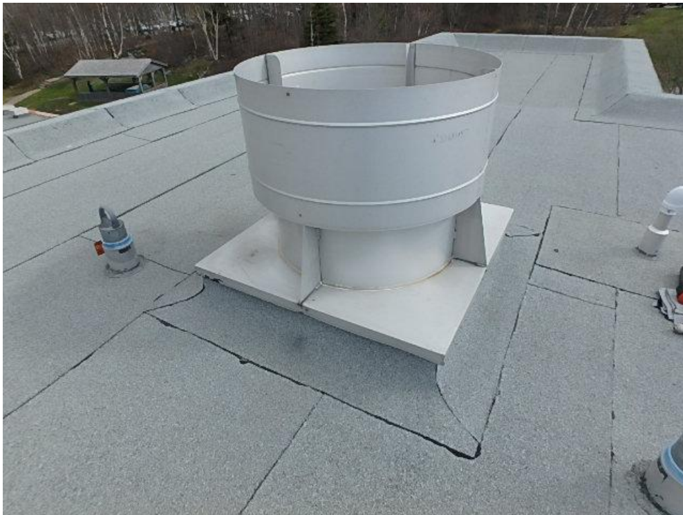
Photograph 50: Roof Area 3.1 – Exhaust fan and conduit gooseneck penetrations.
