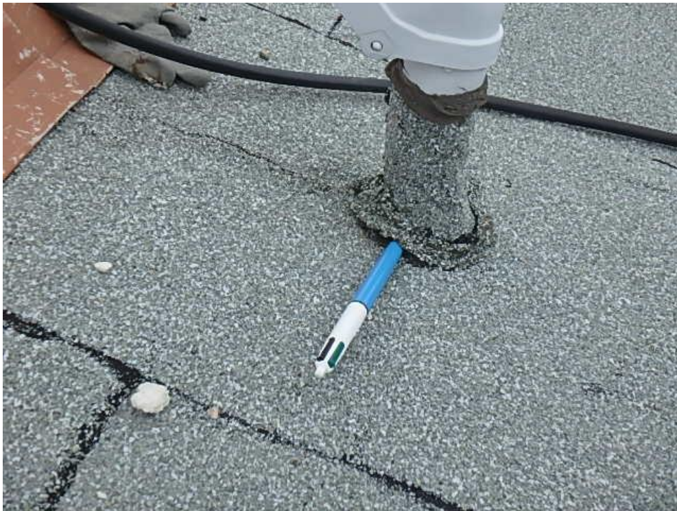
Photograph 6: Roof Area 2.1 – flashing poorly sealed and debonded at conduit gooseneck.
