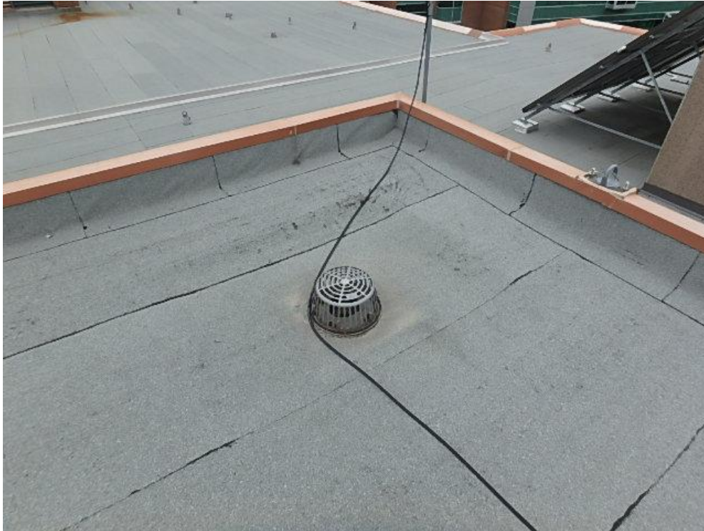
Photograph 25: Roof Area 3.1 – Membrane tenting around parapet, ridging in cap sheet membrane, conduit across roof area and improper cap sheet at roof drain.
