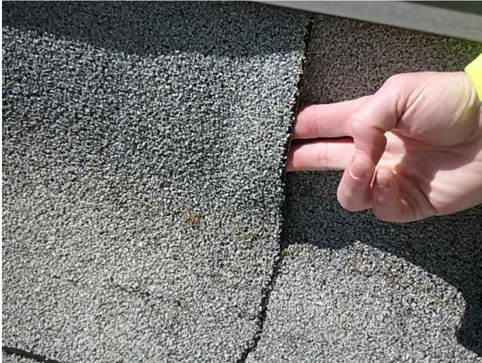
Photograph 7: Roof Area 1.1 – delamination of membrane cap sheet flashing that occurs in multiple locations along parapet.
