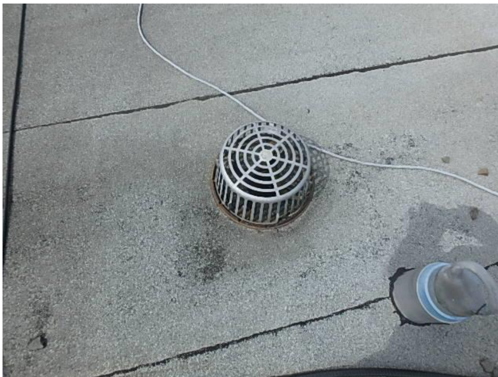
Photograph 30: Roof Area 3.1 – Typical roof drain installation with improper cap sheet detail.
