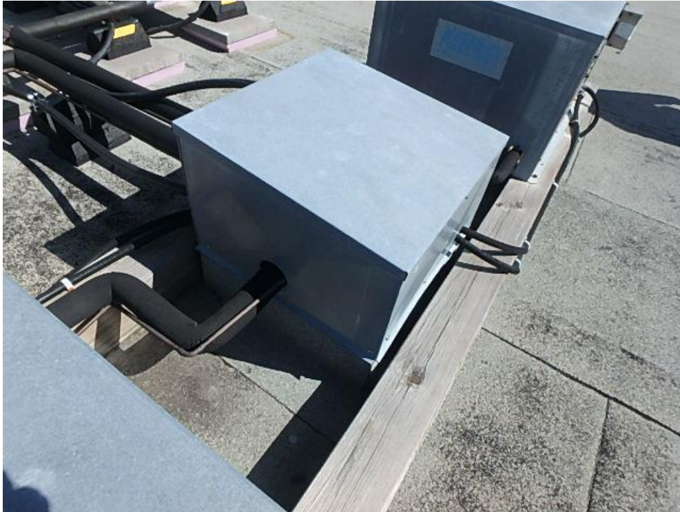
Photograph 11: Roof Area 1.1 – Doghouse penetration detail and HVAC units on sleepers that do not have membrane protection underneath.
