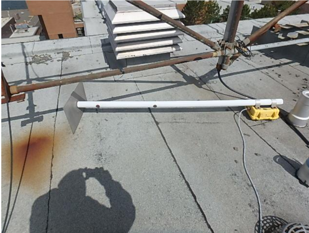
Photograph 25: Roof Area 3.1 – unprotected conduit support and minor debris and membrane rust staining.
