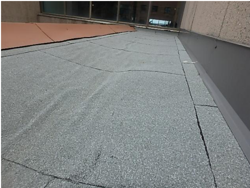
Photograph 4: Holland Building Roof Area 1.2 substantial ridging in membrane throughout roof area.
