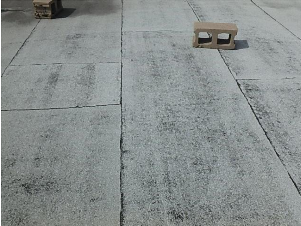
Photograph 3: Roof Area 1.1 – showing debris and membrane wear
