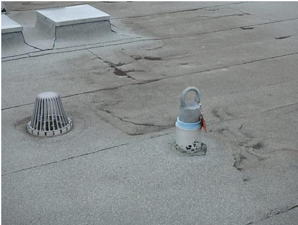
Photograph 56: Roof Area 3.1 – Blistering and ridging in membrane and flashing problems around unused roof anchor. Unused curbs also shown.
