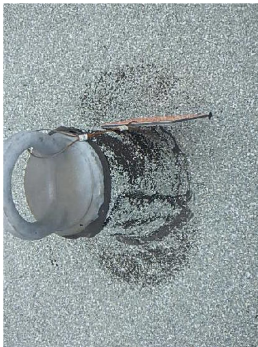
Photograph 31: Roof Area 3.3 – Full view of membrane flashing that is in poor condition around roof anchor.
