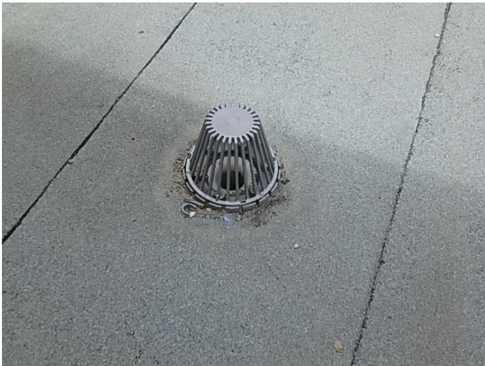
Photograph 30: Roof Area 2.2 – Typical roof drain installation with improper cap sheet detail.
