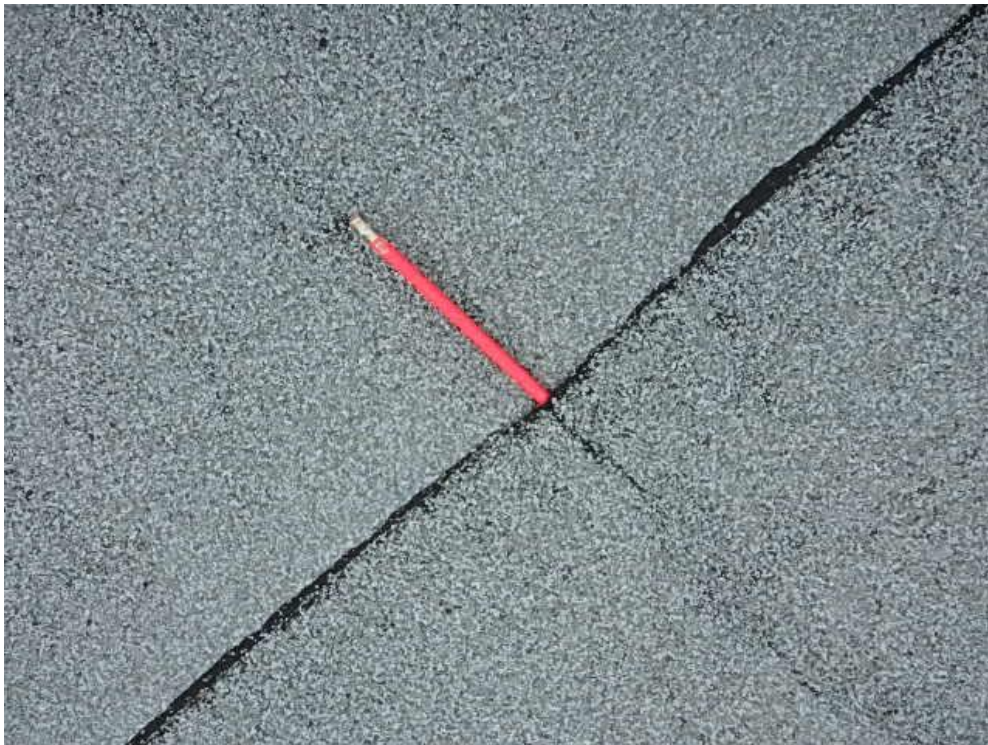
Photograph 66: Roof Area 3.3 – Debonding of membrane flashing is evident in multiple locations.
