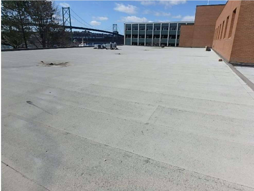
Photograph 1: Overall view of Murray building Roof Area 1.1 looking south towards Halifax. This is a 2 ply modified bitumen roof that is approximately 15 years old
