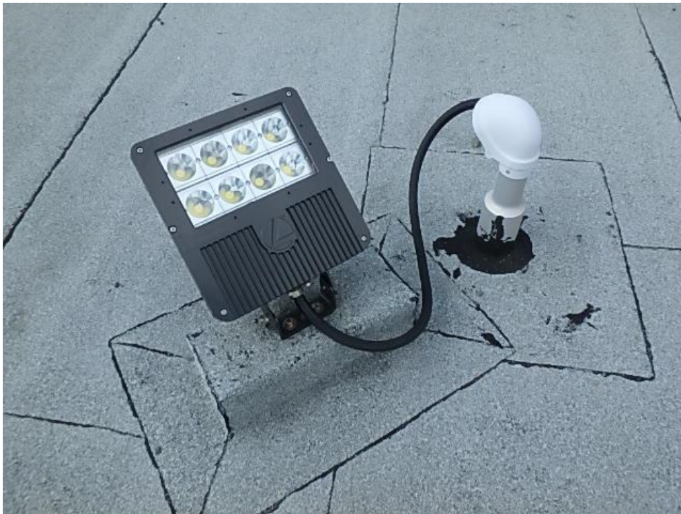
Photograph 12: Roof Area 1.1 – Typical light and conduit gooseneck detail.
