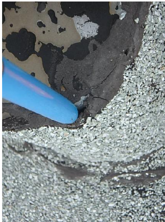
Photograph 30: Roof Area 3.3 – Blistered and poorly sealed membrane flashing around base of roof anchor.
