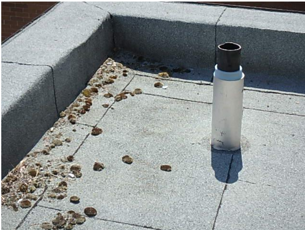
Photograph 28: Roof Area 2.1 – Debris and vegetation growth in corner along with stack penetration.
