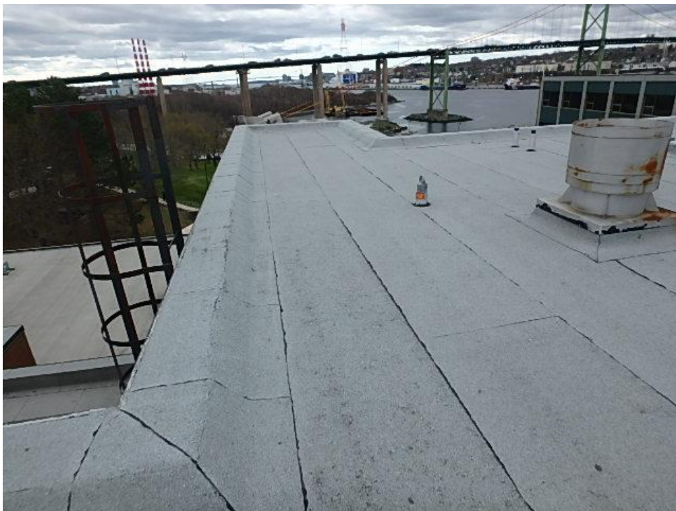
Photograph 60: Roof Area 3.3 – Membrane protection missing at top of ladder.
