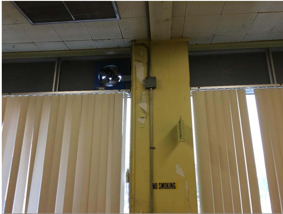
Photo 3: View of the damaged lead-containing paint observed in Location 45 in the Environment Canada Office of the second floor.
