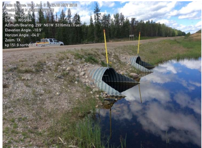
Figure D-2: View of the upstream culvert inlet (left) and the downstream culvert outlet (right) of the Klewi River at Highway 5 km 151.9.
