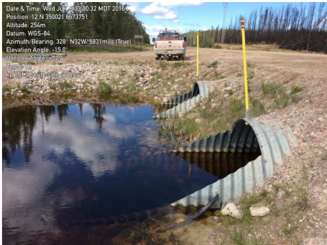
Figure D-2: View of the upstream culvert inlet (left) and the downstream culvert outlet (right) of the Klewi River at Highway 5 km 151.9.
