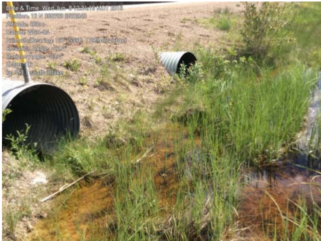
Figure D-4: View of the upstream culvert inlet (left) and the downstream culvert outlet (right) of the unnamed tributary of the Klewi River at Highway 5 km 152.9. Typo for km marker in the embedded note descriptions (kp 153.1 is actually km 152.9).
