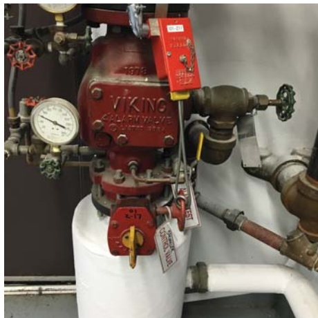
EXISTING PLUG TYPE TAMPER SWITCH IN WORKSHOPS BLDG
