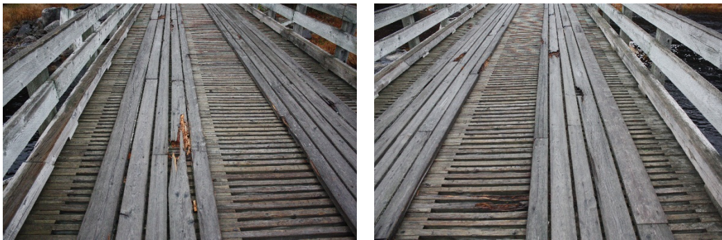
Fig. 2-3. The Mersey River Bridge. Details of the damaged structure. View towards the West.
