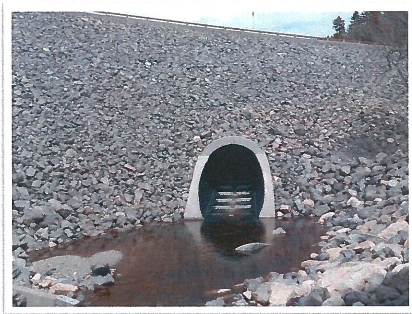
Figure 2. Illustration of proposed new culvert with baffle inserts (not to scale)
