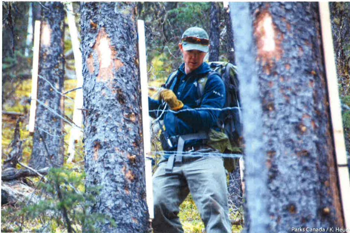
Figure 2: Lumber protecting trees being used as posts (Panther River test fence).
