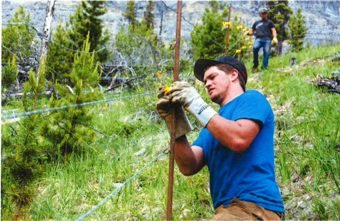
Figure 7: Metal sucker rod posts with two strands insulated for electrification (Red Deer River test fence).
