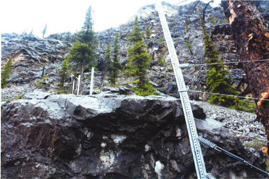
Figure 5: Metal U-channel posts pounded into scree (Panther River test fence).
