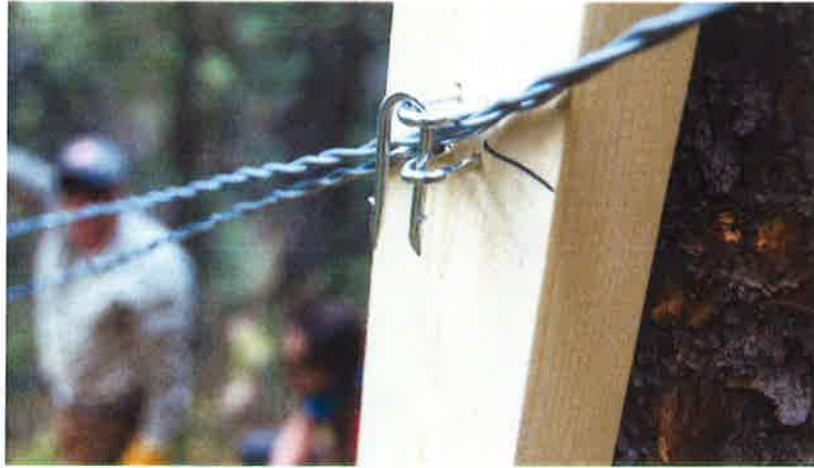
Figure 3: Double-staple-cotter-pin system used for adjusting wire heights (Panther River test fence).
