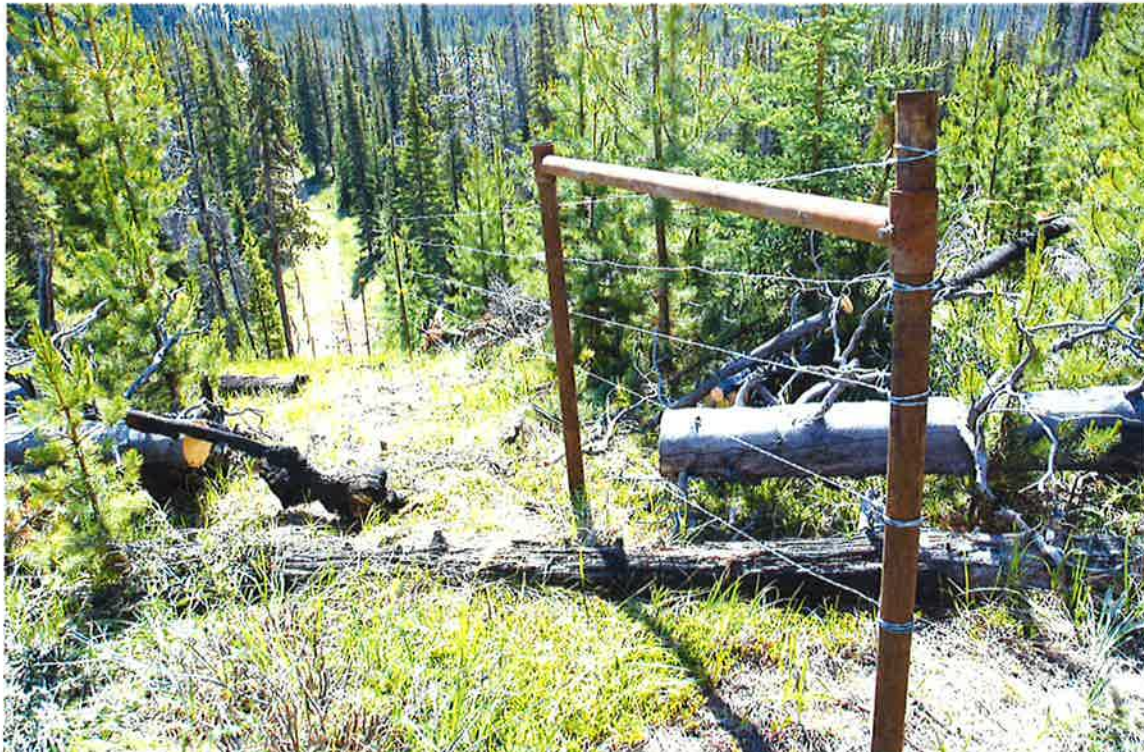
Figure 8: Brace constructed from drill stem.
