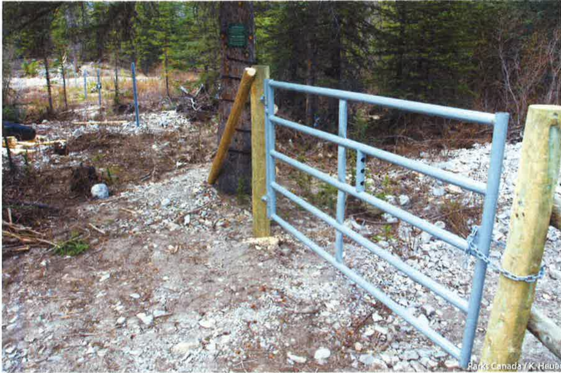
Figure 9: Metal swing gate for horse/hiker access (Panther River test fence – does not include spring mechanism).
