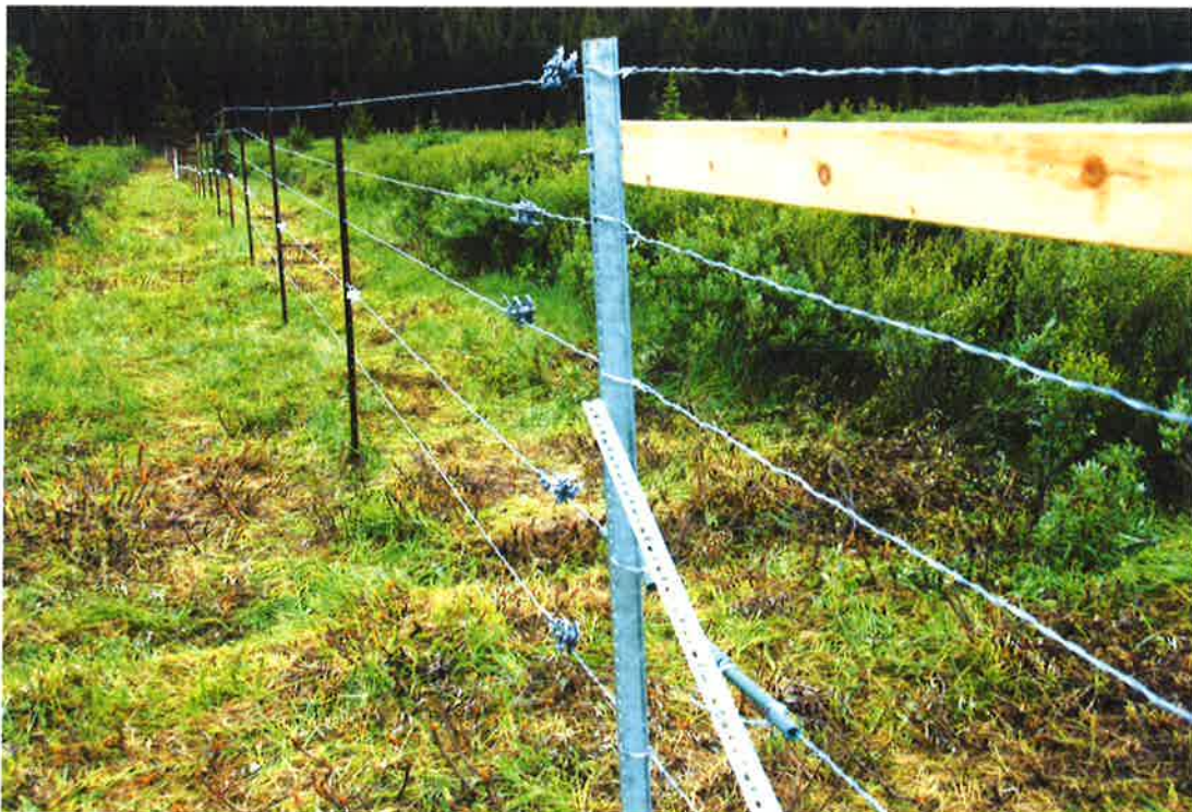
Figure 4: Metal U-channel brace in foreground with metal T-posts in background (with one wire insulated for electrification) (Windy soft release pasture X-fence).
