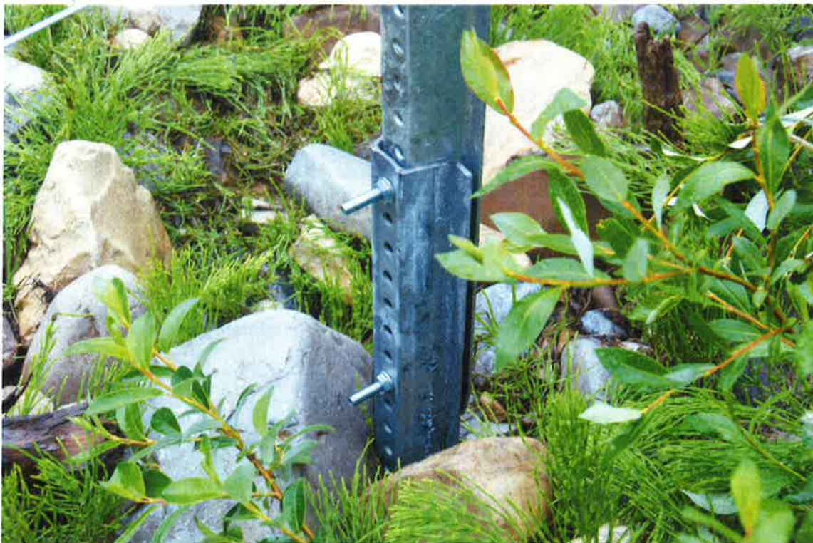
Figure 6: Metal U-channel ground rod (3') driven into the ground and bolted onto 5'-long post (Panther River test fence).
