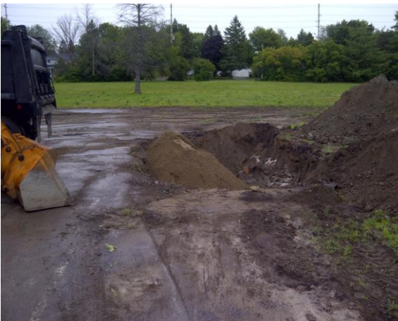
Photograph No. 5: View of clean fill sand being backfilled into the excavation, looking east.
