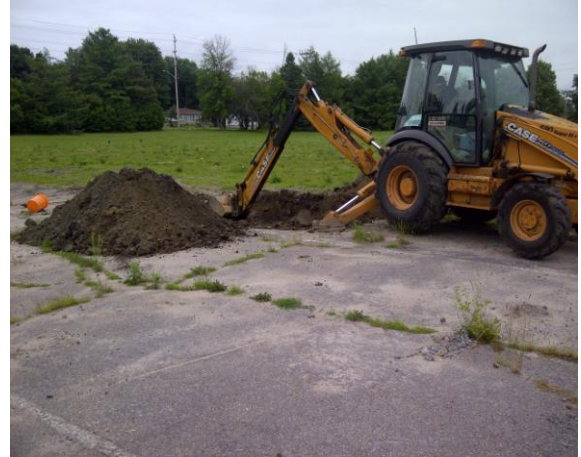
Photograph No. 2: Excavating contaminated soil in the vicinity of the former buried pipeline.
