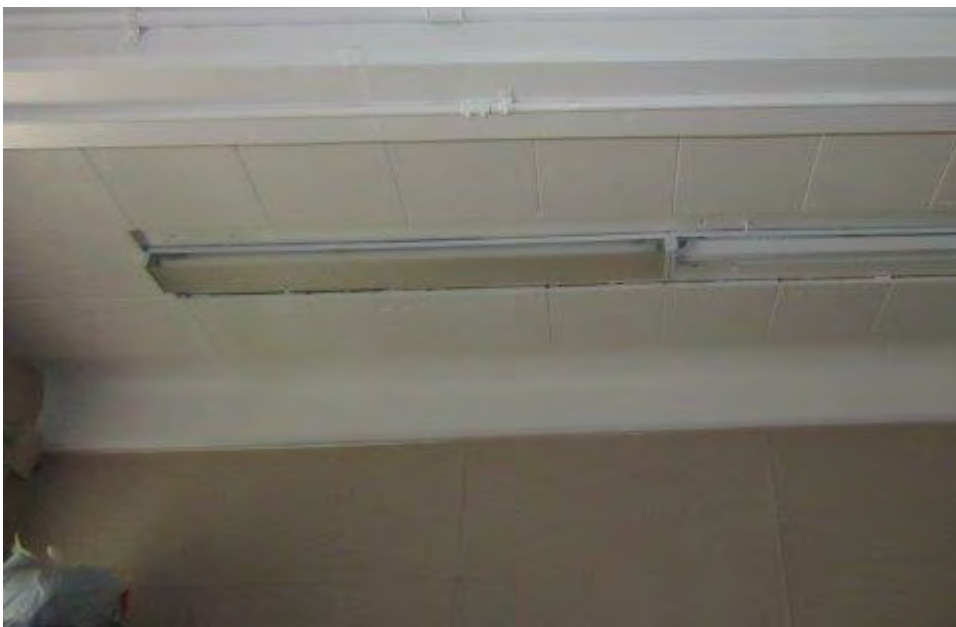
Photograph 6: Typical 12" fiberglass ceiling tiles present in most offices.
