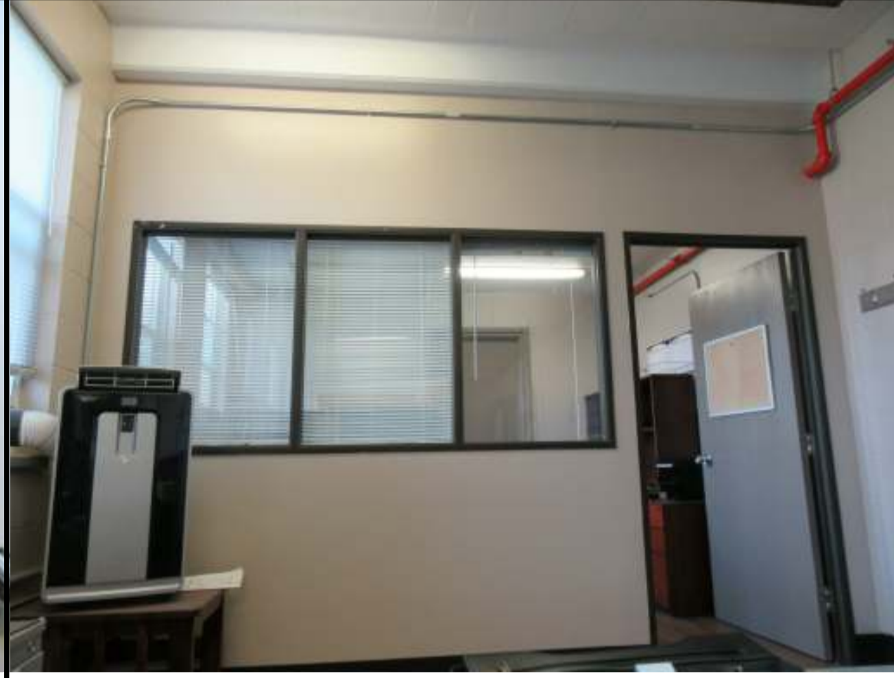
PHOTO 112 F ROOM 108 & ROOM 112
