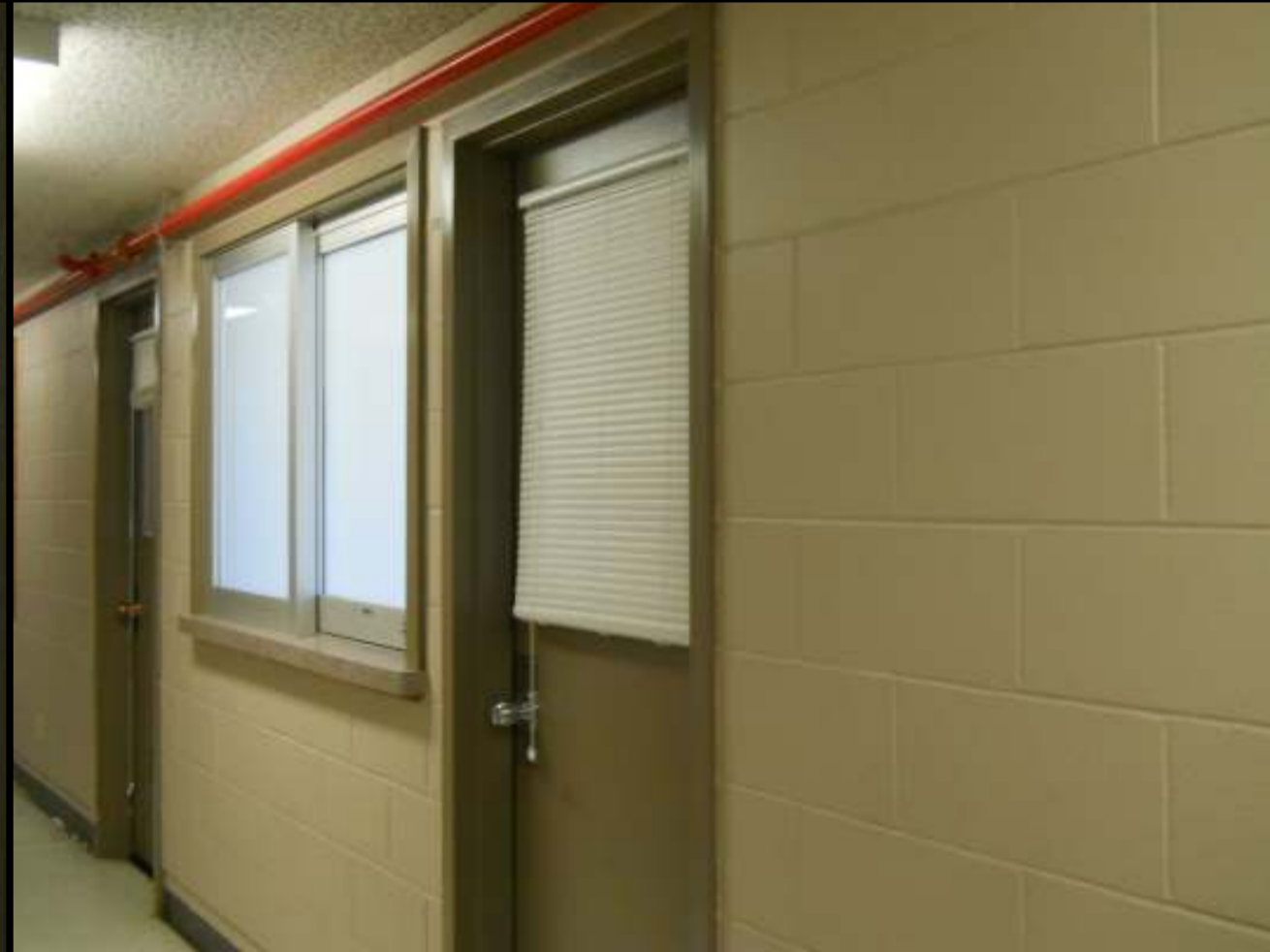
PHOTO 108 J ROOM 108 & ROOM 135
