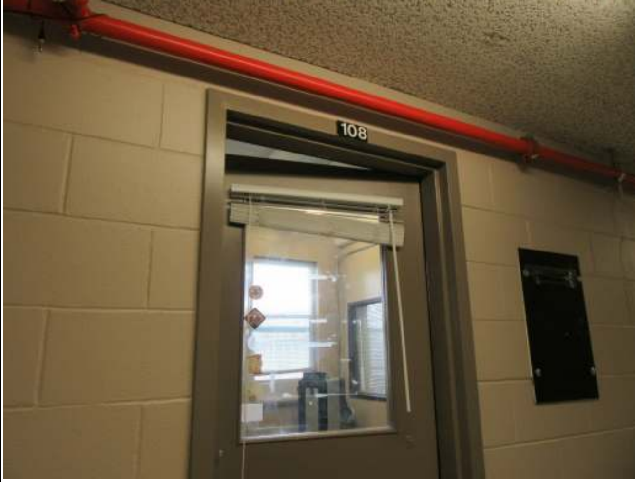
PHOTO 108 A ROOM 108 & ROOM 135
