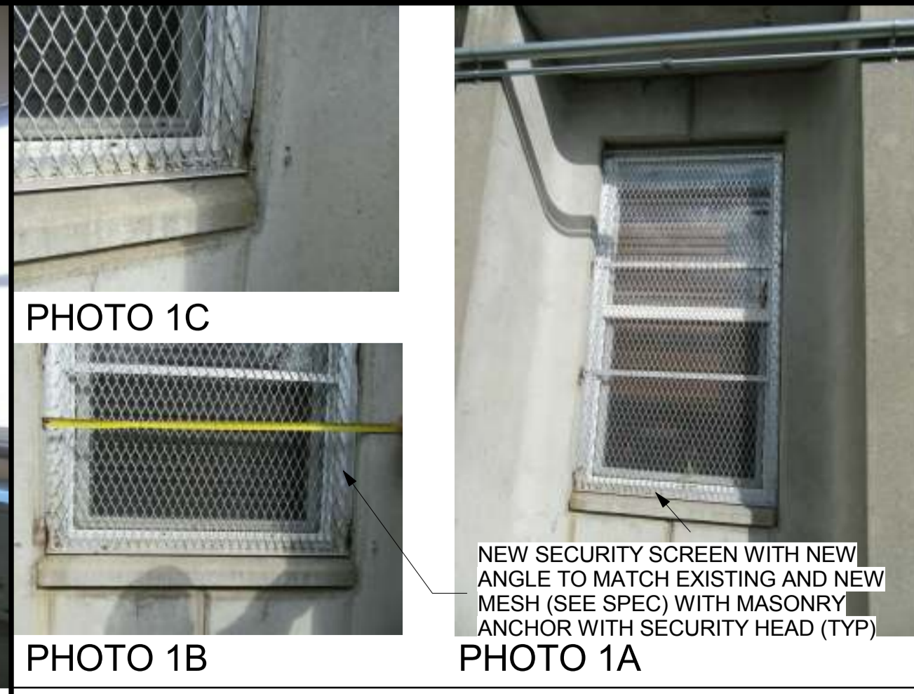
PHOTO 1B PHOTO 1A TYPICAL EXTERIOR WINDOW SECURITY SCREEN
