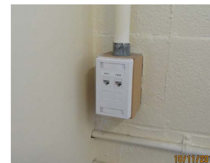
(PHOTO 4) TYPICAL STANDARD DATA OUTLET SCALE NTS
