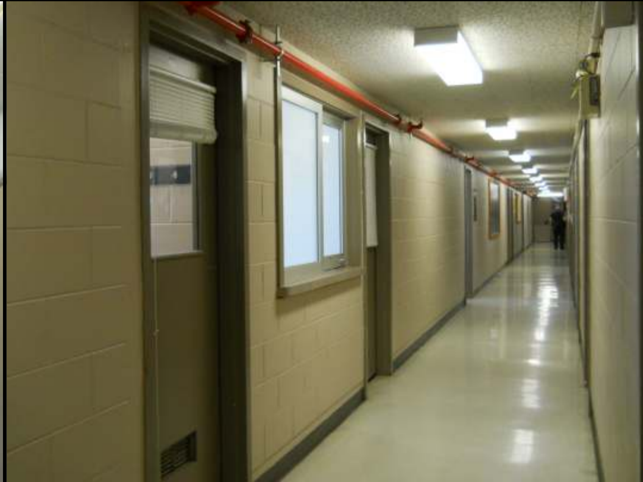
PHOTO 108 K ROOM 108 & ROOM 135
