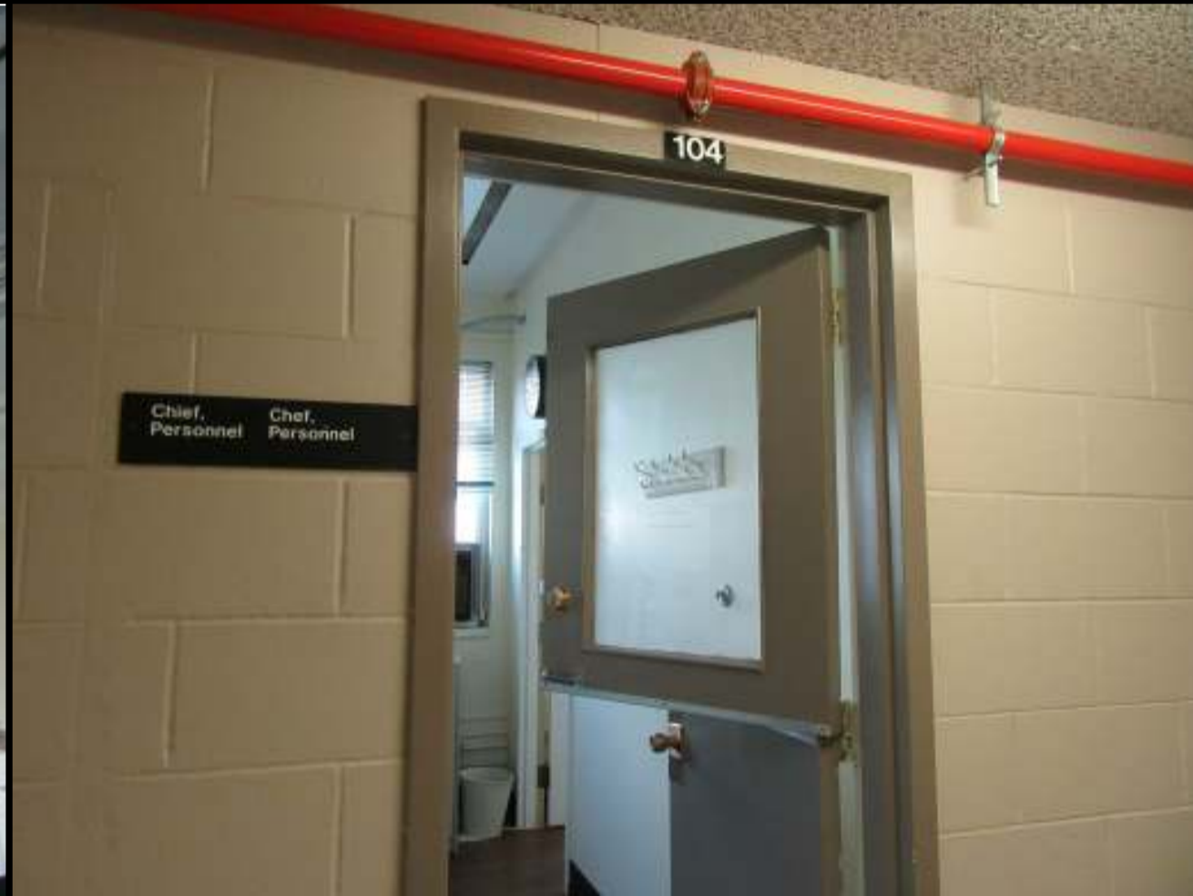
PHOTO 104 A ROOM 104 & ROOM 135
