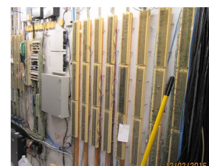
(PHOTO 6) TELEPHONE DEMARCATION SCALE NTS
