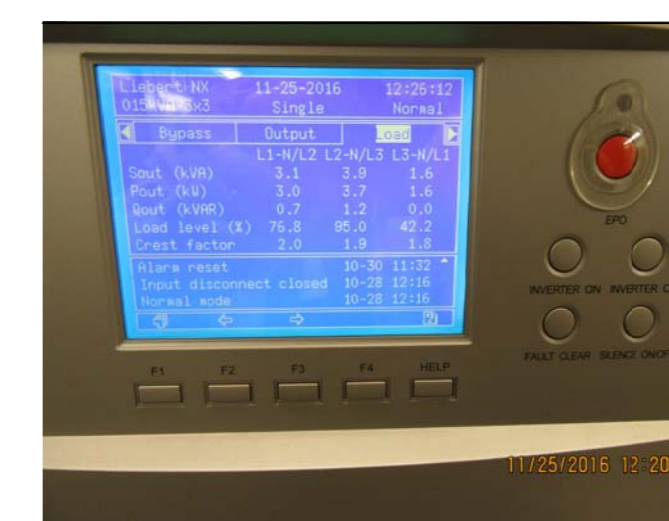
(PHOTO 7) UPS MONITOR DISPLAY SCALE NTS
