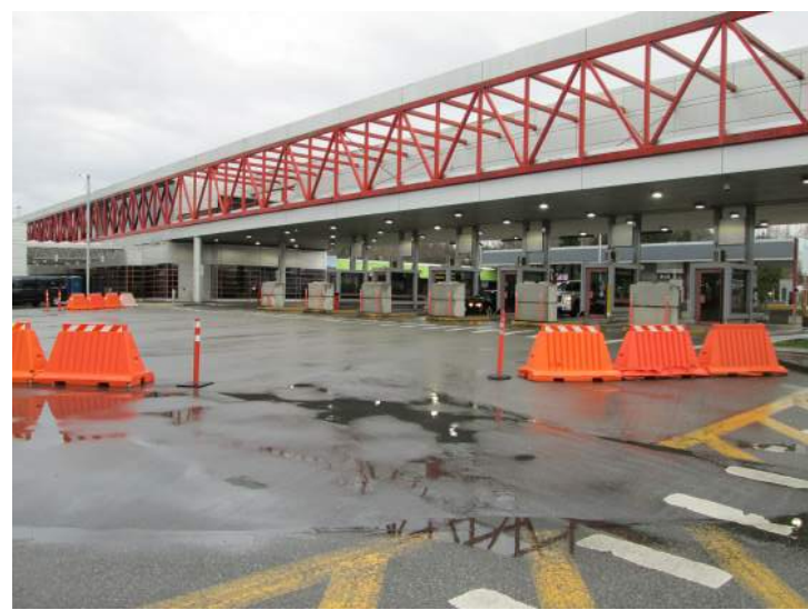
V0 - VIEW OF PROJECT SITE
