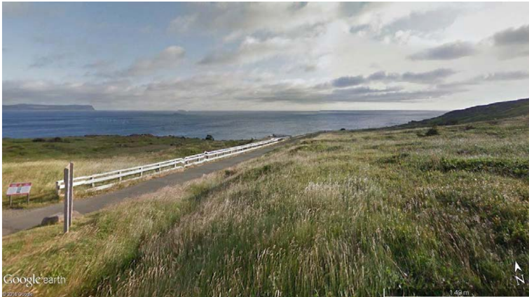
Fig. 4. The paved roadway linking the current parking lot to the WWII battery (Image credit: Anne Desgagné).
