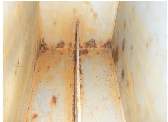
2. Typical tank bottom condition..
