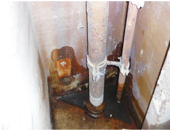
3. Example of standing water in tank..
