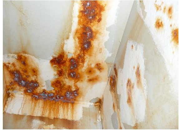
2. Typical tank top paint deterioration..
