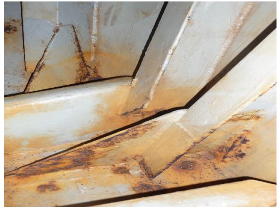
18. Bottom brackets corrosion (typical).
