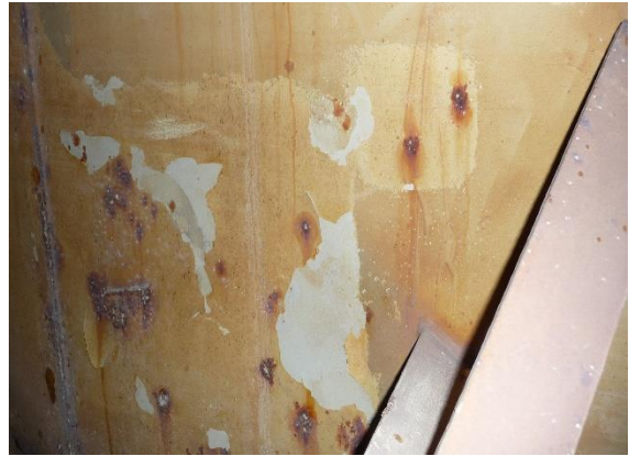
8. Example of spalling of paint.
