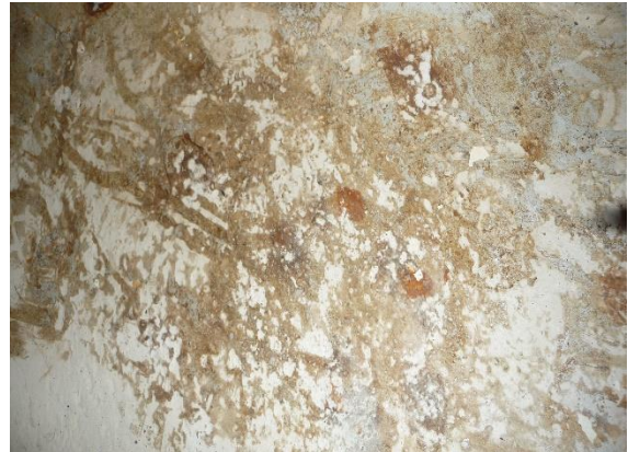
6. Typical bottom shell condition showing minor pitting.
