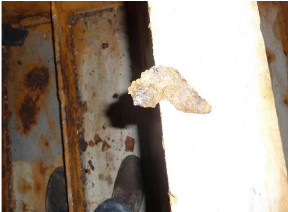
9. Typical scaling on webs and face flats.
