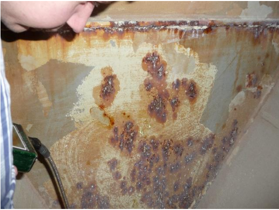
9. Example of web and face flat corrosion
