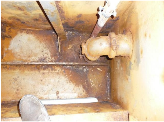
3. Bottom shell corrosion (typical)
