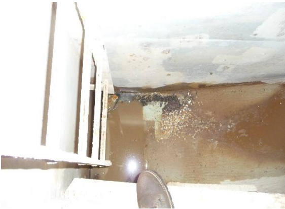
13 Example of standing water in the tank.
