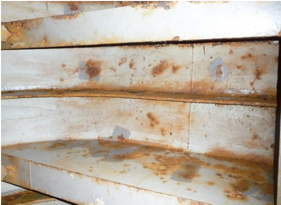
5. Typical Bottom Shell corrosion
