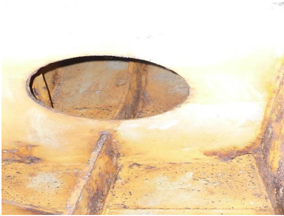
19 Corrosion under crane pedestal.
