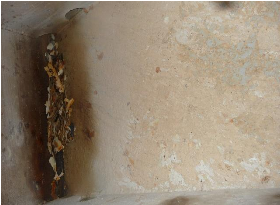
5. Paint flakes trapped in way of drainage point.
