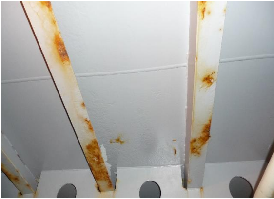
3. Deck head corrosion (typical)
