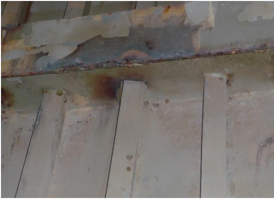
3. Framing corrosion (typical)
