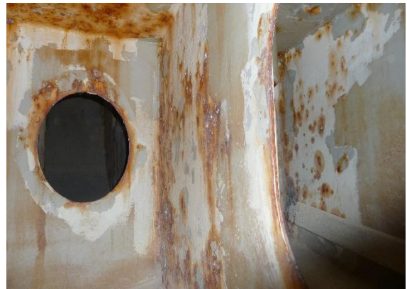
4. Typical Girder- Floor corrosion.
