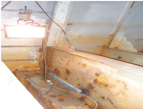
5. Typical Floor corrosion and new anode.
