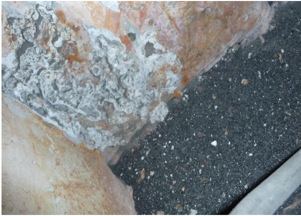
7. Typical paint deterioration in way of pitting.
