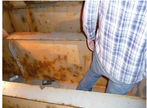
20. Webs of Floor corrosion (typical).
