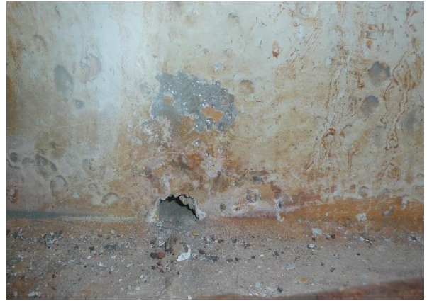
8. Example of pitting and poor quality water way.
