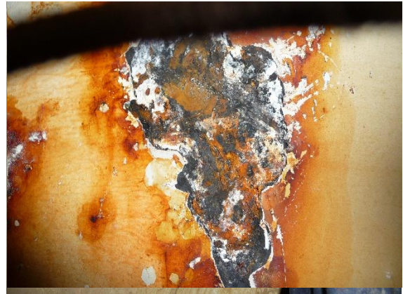
8. Blister removed showing typical corrosion on web of Floor.
