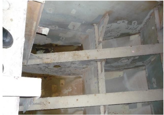
12. Typical tank bottom corrosion.
