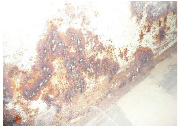
6. Corrosion at bottom half of Web of floors
