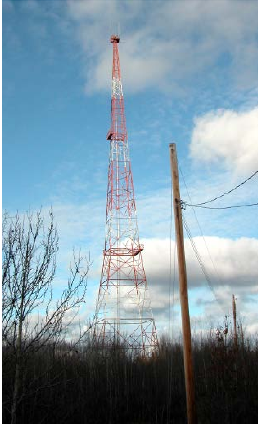
Existing tower to remove
