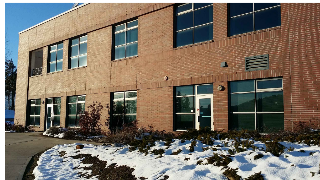
PHOTO 5: VIEW OF EXTERIOR WALL AT GRIDS 1/A-K
