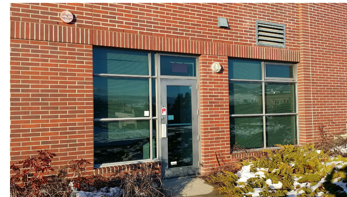
PHOTO 7: VIEW OF EXTERIOR WALL AND GRILLS AT GRIDS 1/J-K
