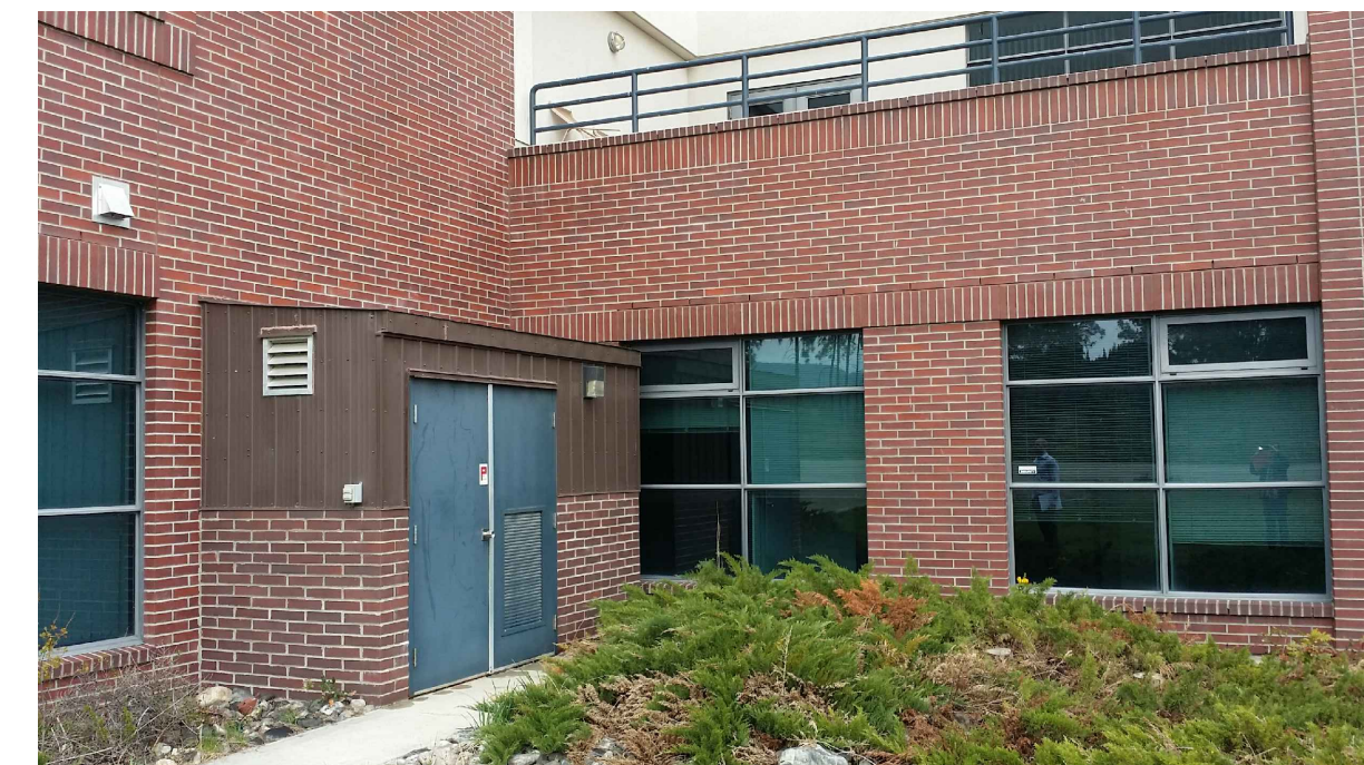
PHOTO 6: VIEW OF EXTERIOR WALL AND GRILLS AT GRIDS C/1-2
