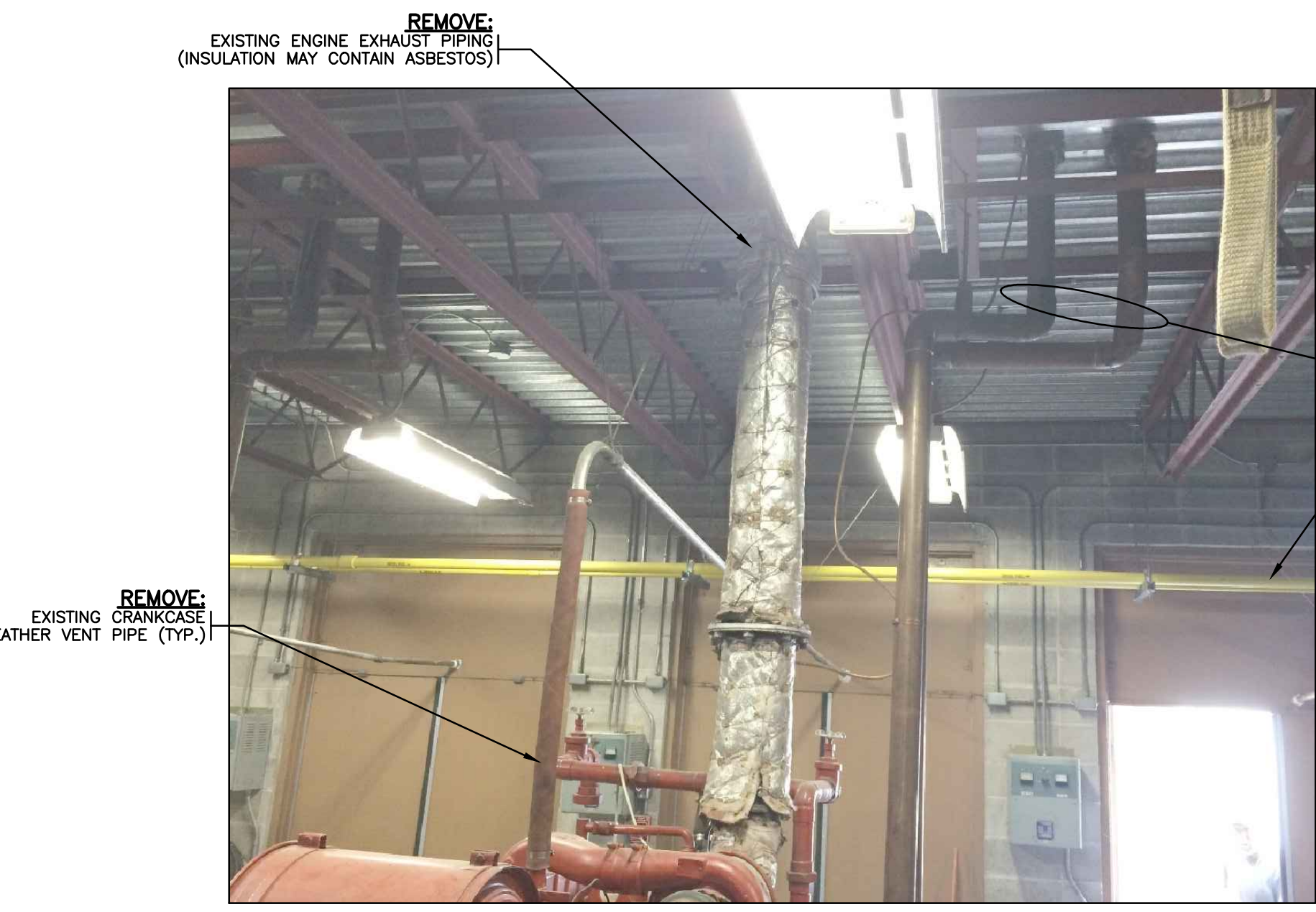
PHOTO 1 ROOF EQUIPMENT DEMOLITION N.T.S.
