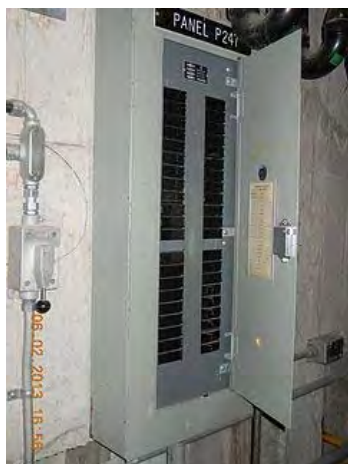
Typical access restriction of panel. Typical of 3 panels in service space.
