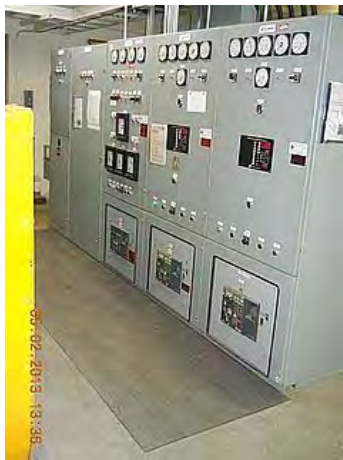
Synchronizing control panel.
