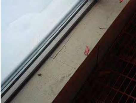
Deteriorated wood sill at windows.
