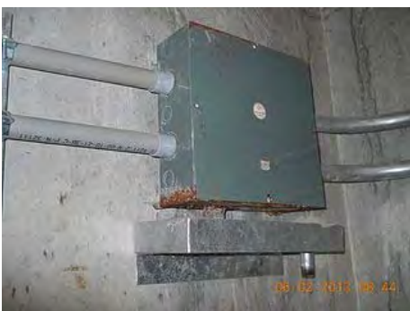
Rusting pull boxes. Typical for two.
