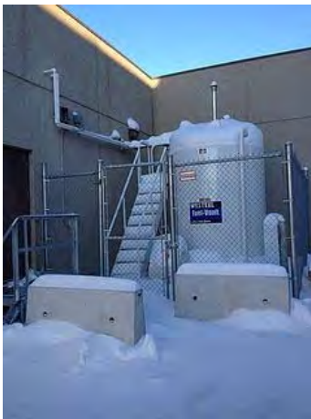
Outdoor fuel storage tank for Gensets
