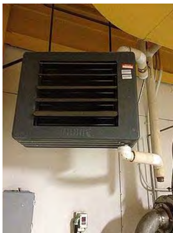
Unit Heater - Mezzanine level
