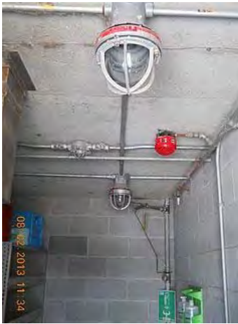
Explosion proof wiring in hazardous storage rooms.
