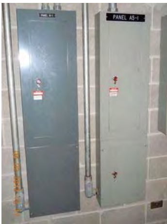
Panel A5-1 c/w lighting control contactor in lower section.
