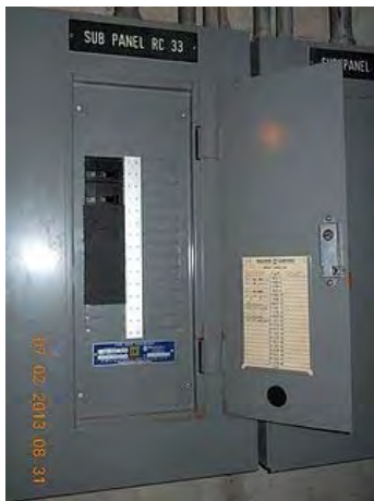
Typical Square D panel installed for refrigeration upgrade.
