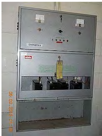
Emergency lighting panel in Service Building.
