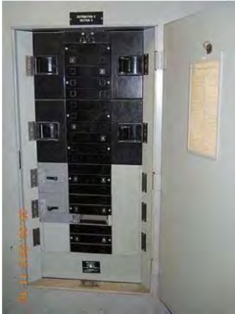
Westinghouse CDP in distribution enclosure.
