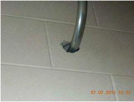
Fire stop missing on wall penetration.
