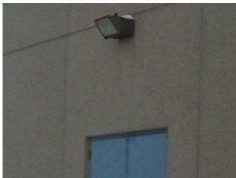
HPS light fixture over west loading doors.
