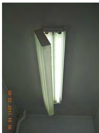
T12 wrap around fixture.
