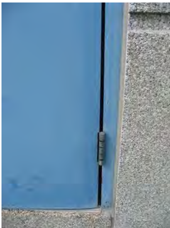
Damaged hinge at east door.
