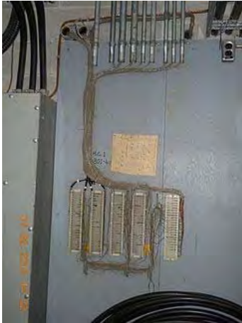
Telecom service cable from main building.
