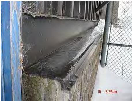
Lack of drainage at sill flashing causing water / ice buildup.
