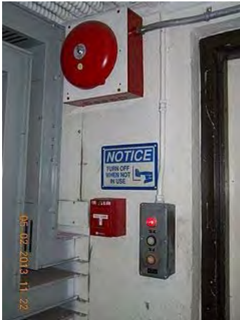
Typical 2 stage pull station and alarm bell. (no visual devices)
