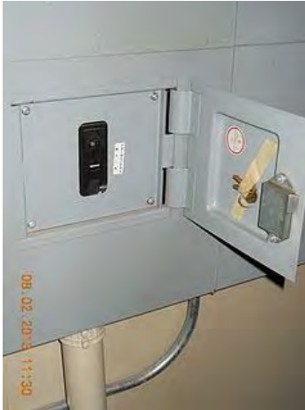
Main breaker in distribution panel.
