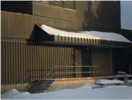
Sloped metal clad Canopy above loading dock.
