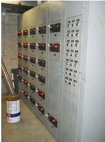
Backside of Motor Control Centre.
