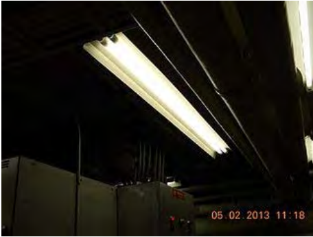
T12 lamp fluorescent fixture.
