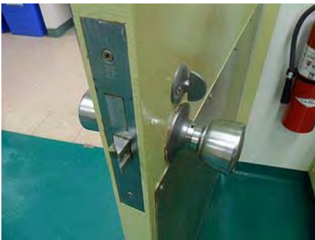
Typical lab metal door with thumb-turn deadbolt and knob handset.
