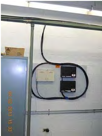
Fibre optics carrier cable.
