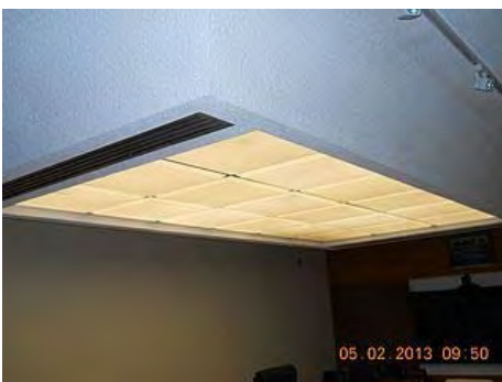
Luminous ceiling installation.
