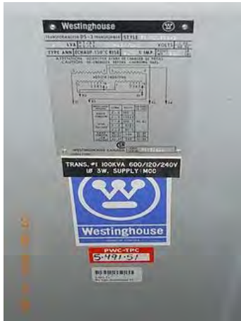
Westinghouse transformer identification plate.
