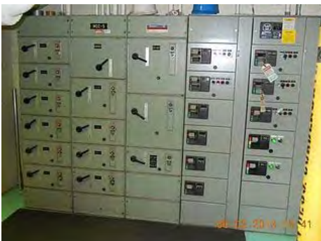
Typical Westinghouse 1972 MCC. Two new sections added.
