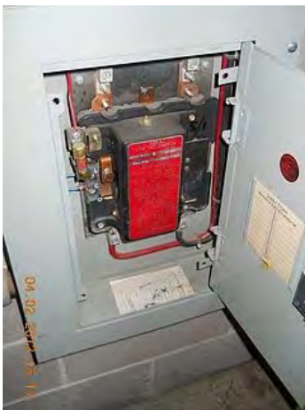
Typical panel contactor for lighting control.
