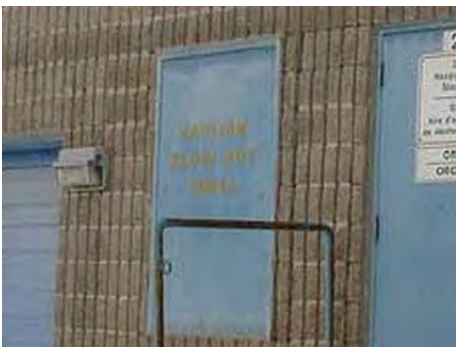
Blowout panel, east elevation, at hazardous materials area and loading dock.
