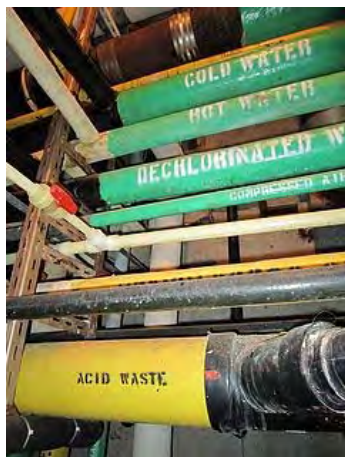
Natural gas line (top yellow pipe) in service corridor for laboratory use only
