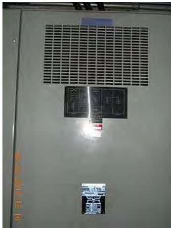
Typical enclosed free standing distribution with integral transformer.
