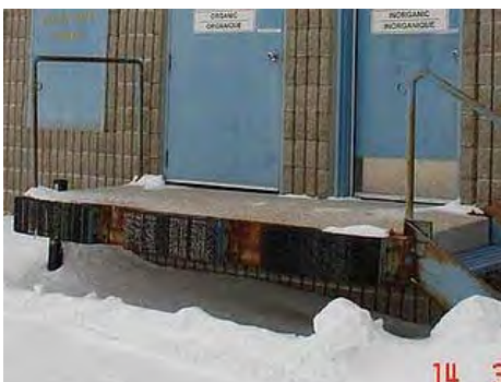
Exterior concrete loading dock with rusted steel framing and worn rubber bumpers.
