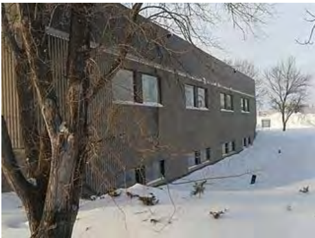
Fixed aluminum windows (north exposure).
