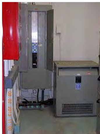
Transformer at service entry.
