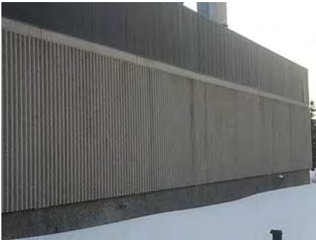
Ribbed precast concrete panels.
