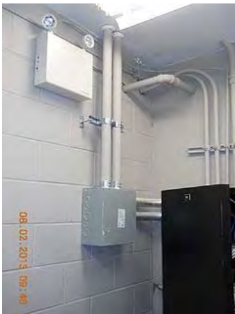
EMT conduit and wiring.
