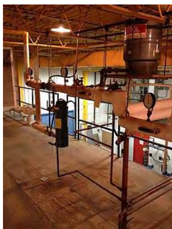
Boiler hot water loop pot feeder
