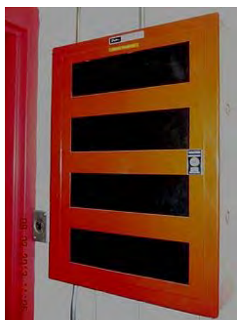
Fire alarm panel in electrical room.
