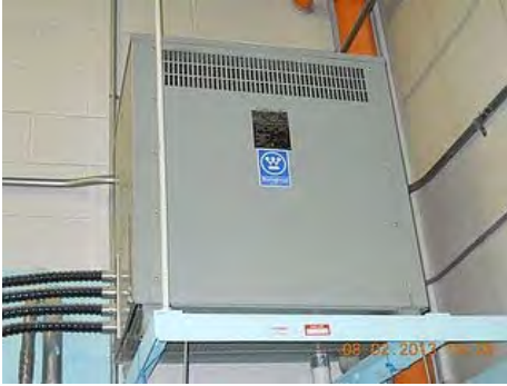
Transformer above CDP in warehouse.
