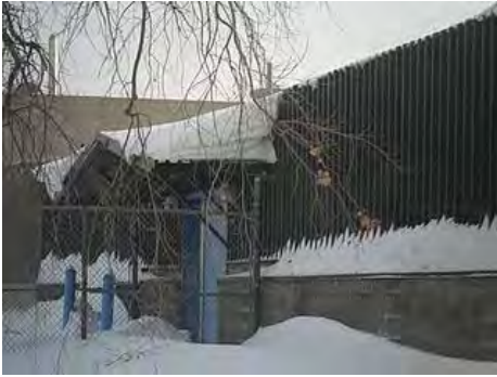
Metal Cladding at North wall and canopy constructed at overhead door.
