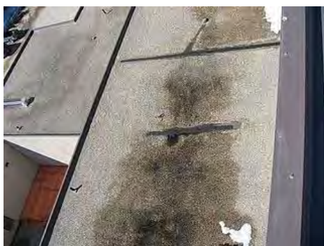
Built-up roofing (at Service Block) showing roof repairs and residual water pooling.
