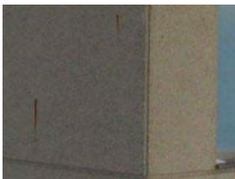
Iron spotting on west wall near southwest corner.
