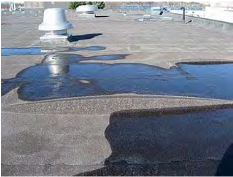
Roof area with deteriorated SBS roof membrane.
