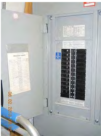
Panelboard for scanning.
