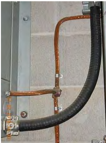
Bare copper ground conductors.
