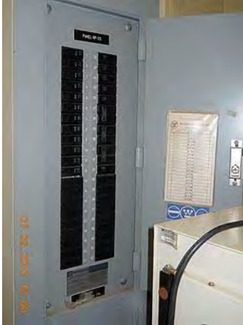
Panel access restricted by lab equipment.
