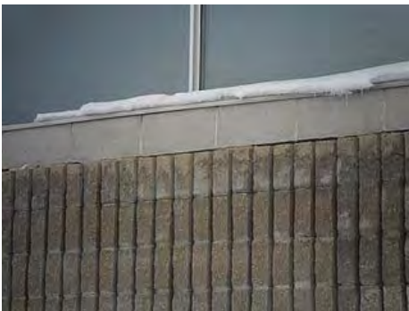
Single wythe of block beneath windows. Mortar joint deteriorated.
