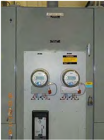
Utility Meters in 2002 switchboard.
