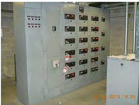
Main Service breakers for Annex in MCC.
