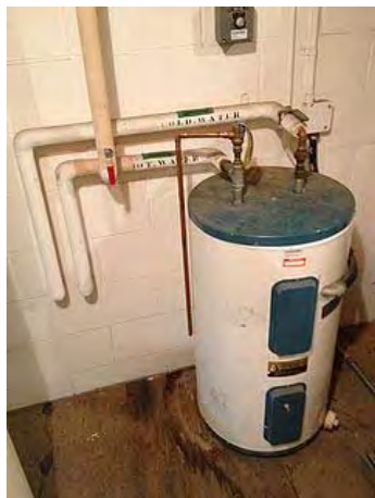
190 litre hot water tank on mezzanine level
