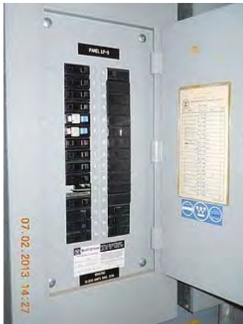
Filler plate missing.
