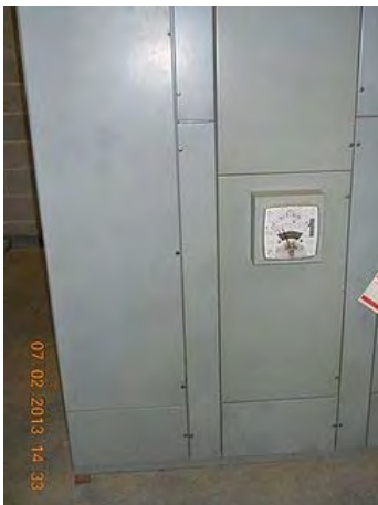
Customer meter in first section of MCC.
