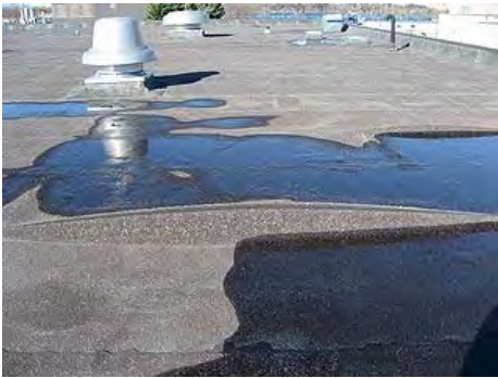
Blister of Modified bitumen roofing. Repaired in 2012.
