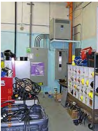
Main service with two CDPs and transformer.
