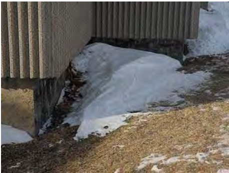
Settlement of Grade at Exterior wall.
