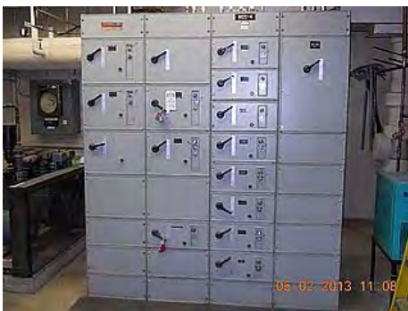
MCC #4 - one of 7 units, total of 41 sections.
