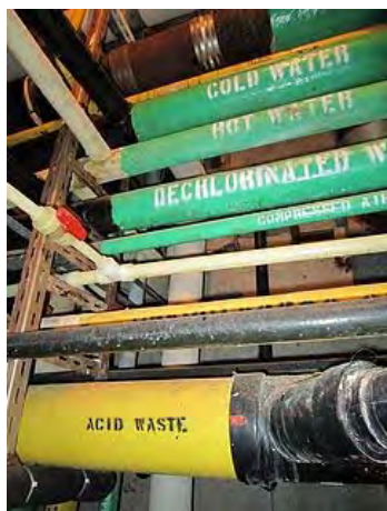
Rack of various plumbing piping in service corridor
