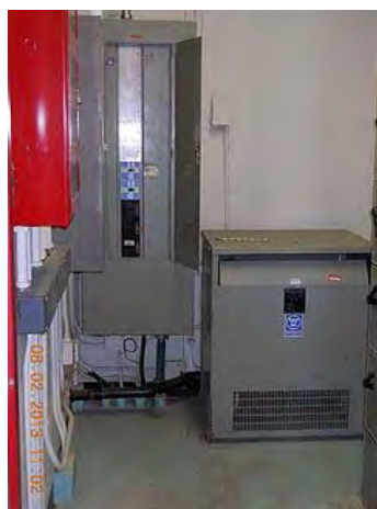
Grounding at service entry, below panel.
