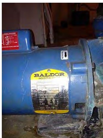
Hot water circulating pump
