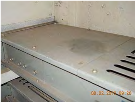
Horizontal bus duct needing cleaning.
