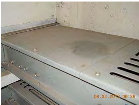
Typical bus duct.
