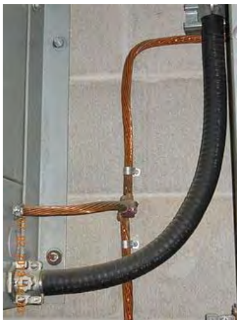
Grounding of transformer.
