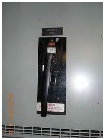
Air Circuit breaker not labeled.
