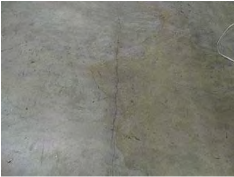
Hairline cracking in concrete slab (storage room).
