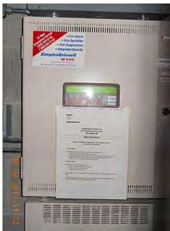
Expansion panel for local Fire Alarm system.
