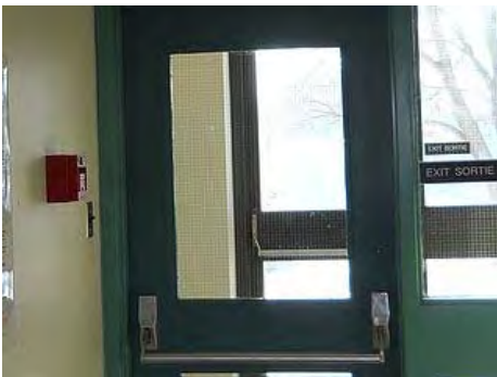
Two stage pull station at front entry.
