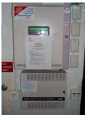
Sub panel for gas suppression system.
