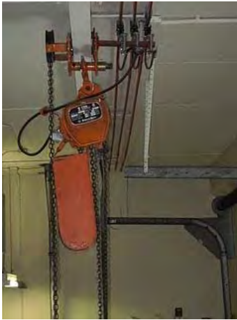
Chain Hoist by loading dock in Water Treatment room
