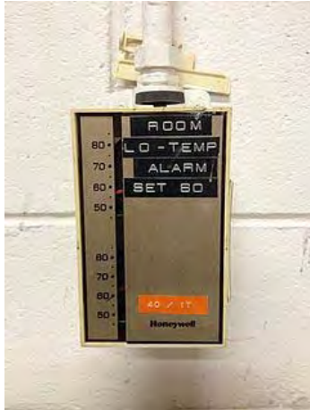
Thermostat control for heating valve on AHU
