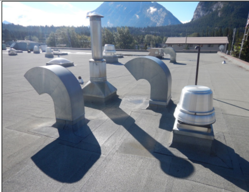
Photo 20 – Existing roof penetration curbs included : B vents, goose neck vents, turbine exhaust fans. Detail drawings should be provided for these penetrations.
