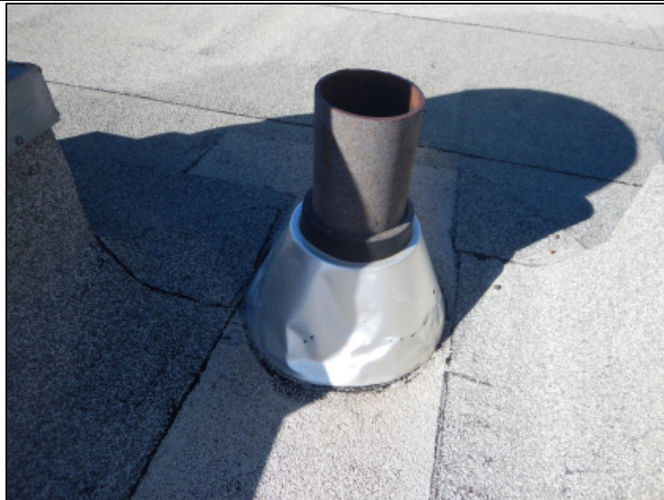
Photo 18 – Existing plumbing vent pipe penetrations are waterproofed via aluminum roof jacks complete with neoprene collars. The existing field membrane terminates on the horizontal at the base of the roof jack. WEC recommends all roof penetrations are curbed up to a minimum of 200mm in height above the finished level of the new primary roof membrane.
