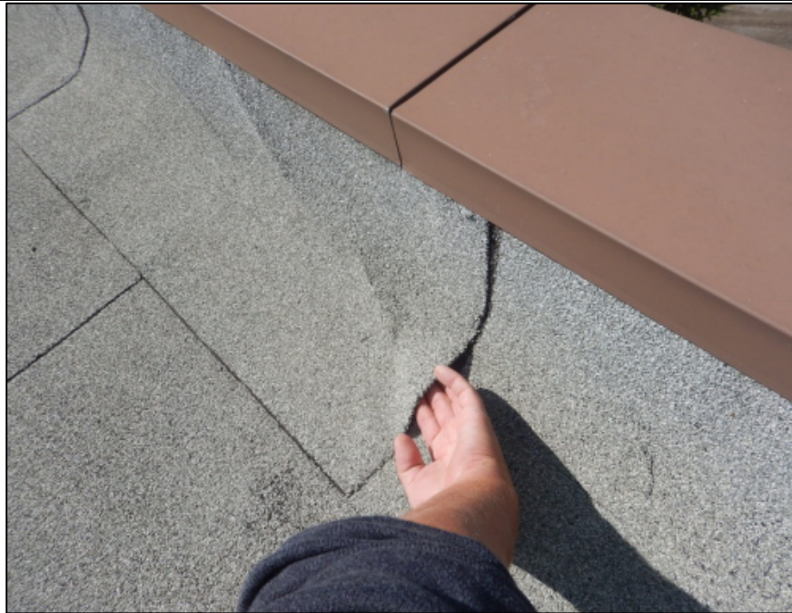
Photo 27 – Open and unsealed parapet wall cap stripping laps were observed on the inside face of the Garage's upper roof section.
