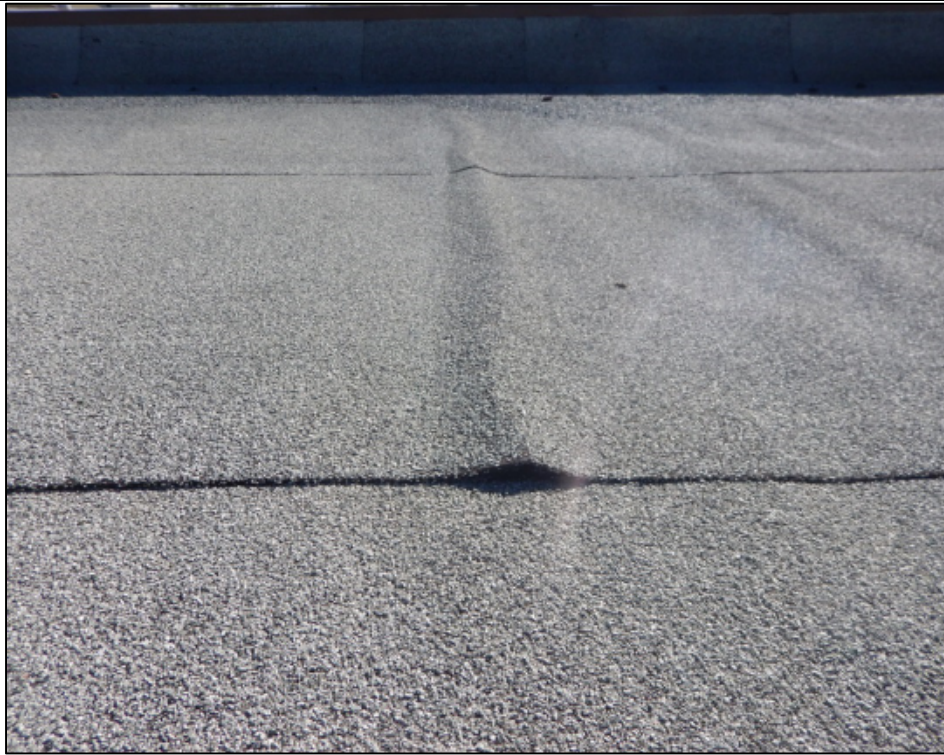
Photo 5 – Open and unsealed side laps in the cap sheet were observed where cross sheet membrane ridges are present on Building 1's roof.
