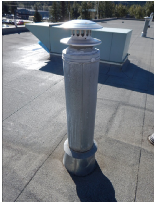
Photo 17 – Existing B vent pipes are waterproofed via galvanized metal roof jacks, storm collars and sealant. The existing field membrane terminates on the horizontal at the base of the roof jack. WEC recommends all roof penetrations are curbed up to a minimum of 200mm in height above the finished level of the new primary roof membrane.
