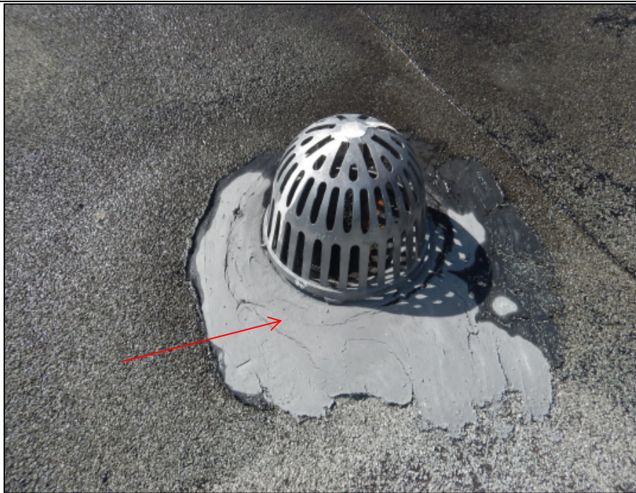
Photo 29 – Past repairs were observed to have been made at the Garage roofs' internal roof drains.
