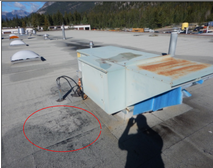
Photo 11 – Degranulation of the existing cap sheet was observed immediately below the RTU service doors on Building 1.
