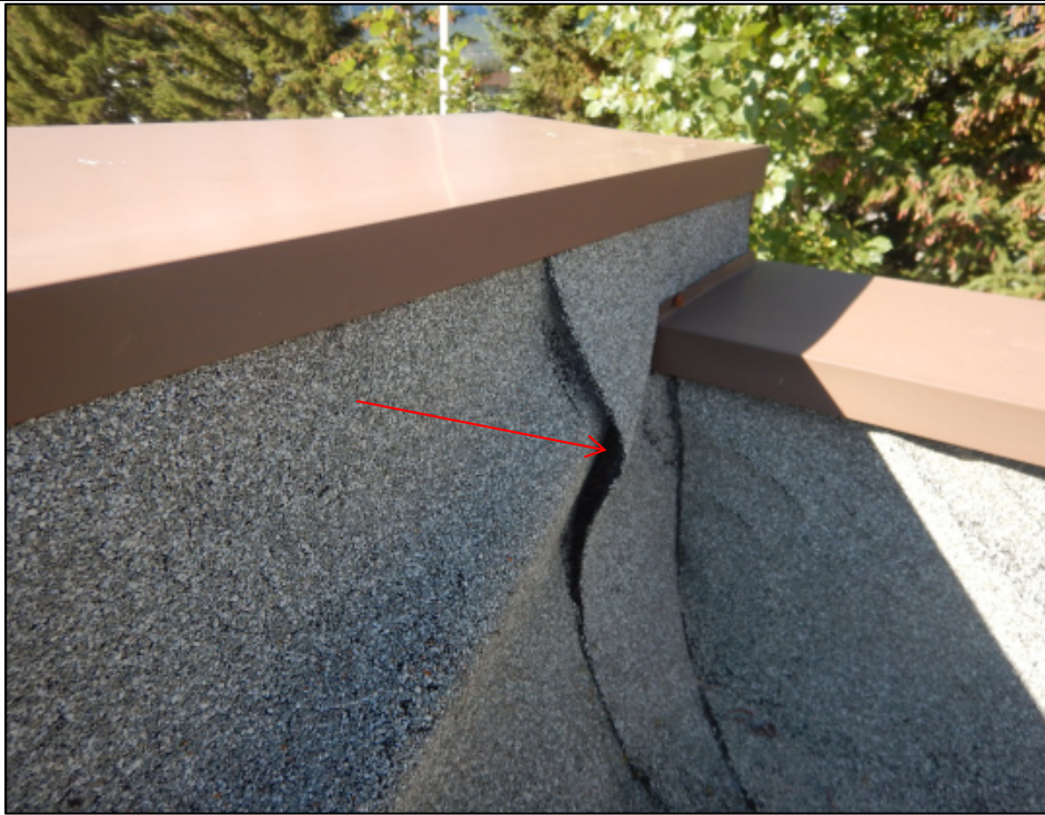
Photo 3 – Membrane stripping laps were observed to be open and unsealed on the inside face of Building 1's parapet walls.
