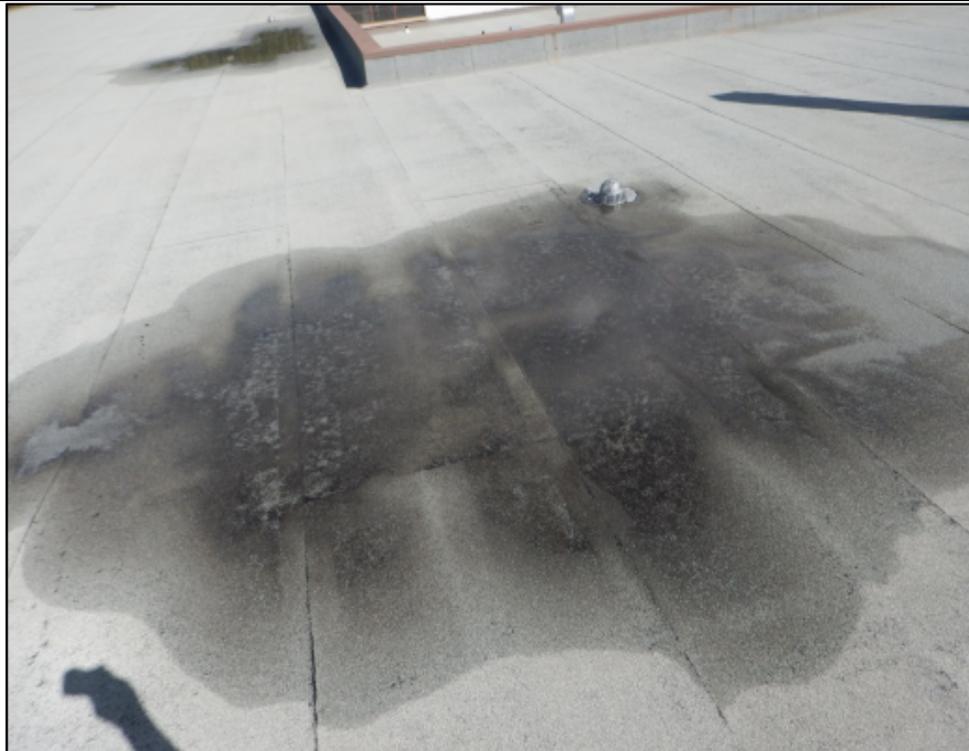
Photo 25 – Ponding was observed adjacent to the existing roof drains on the Garage's upper roof section.
