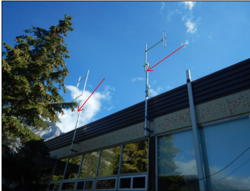
Photo 14– Existing communications equipment will need to be removed from the fascia cladding and parapet wall caps of Building 1 and the Garage to allow for the removal of the existing roof components and installation of new roof assembly components.
