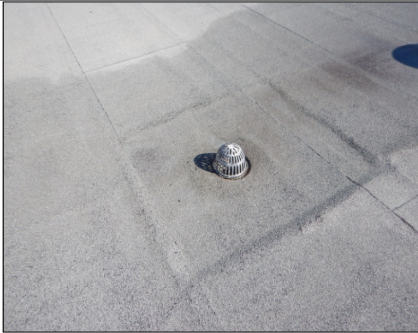
Photo 19 – Existing internal drains have recessed sumps to aid in collecting rain and melt water from the field of the roof. Consideration should be given to installing new tapered insulation drain sumps around new cast metal internal roof drains.
