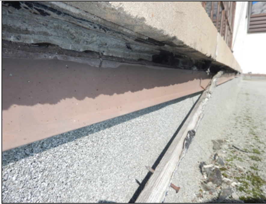
Photo 23 – The leading edges of the existing roof membrane stripping plies is open and unsealed at the base of the high walls on the Garage's lower roof section.
