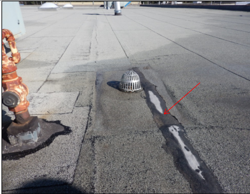
Photo 1 – Previous repairs were observed at cap sheet side laps immediately adjacent to an internal roof drain on the roof of Building 1.
