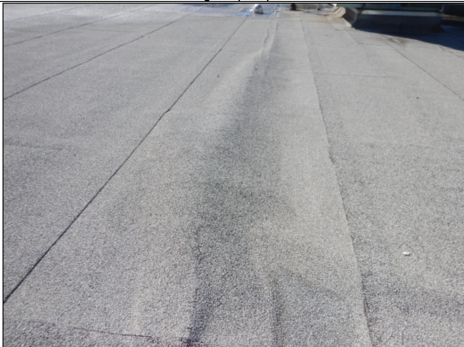
Photo 4 – Numerous cap sheet blisters were observed throughout the field of Building 1's roof membrane.
