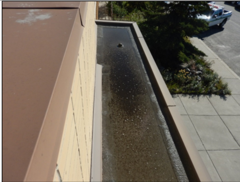
Photo 13 – Ponding was observed on the entrance canopy roof and is a result of inadequate positive slope to the internal roof drain and possible a blocked drain. There is no existing emergency overflow scupper on this roof.
