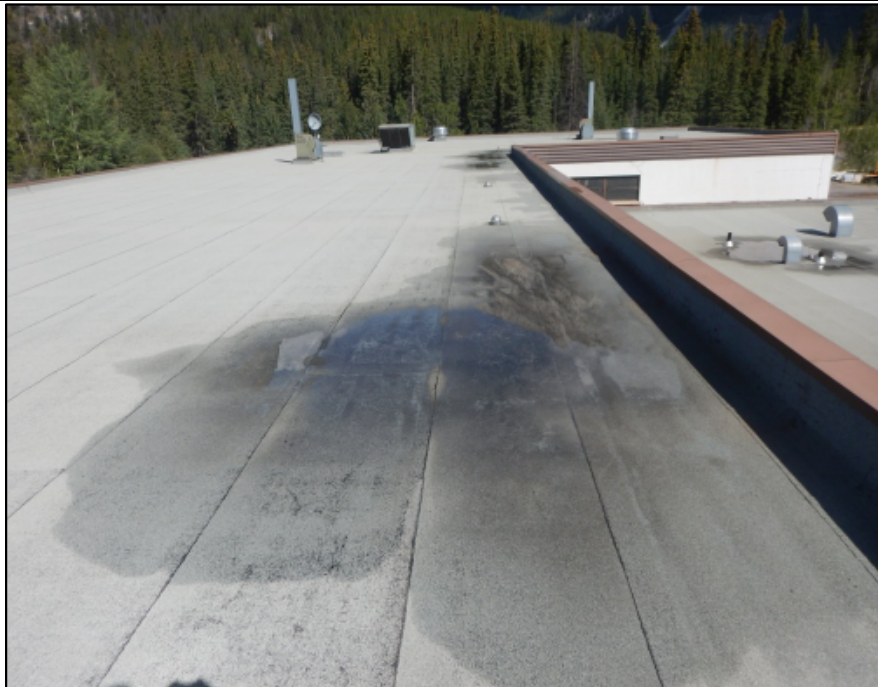
Photo 26 - Ponding was observed adjacent to the existing roof drains on the Garage's upper roof section.
