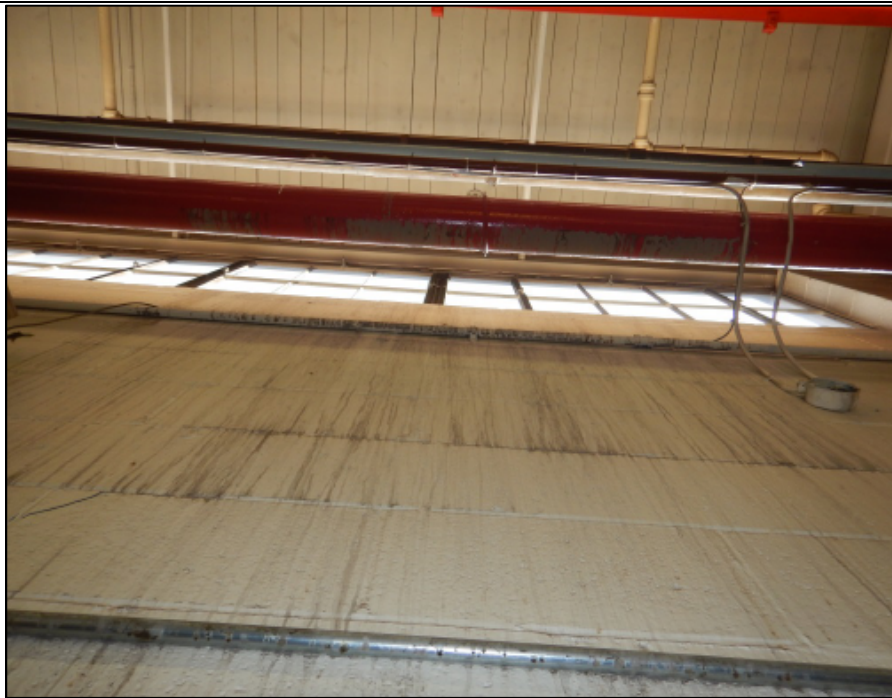
Photo 21 – Onsite personnel reported active leaks occur in the Garage immediately below the clerestory windows. Stains were observed on the inside face of the concrete block wall.
