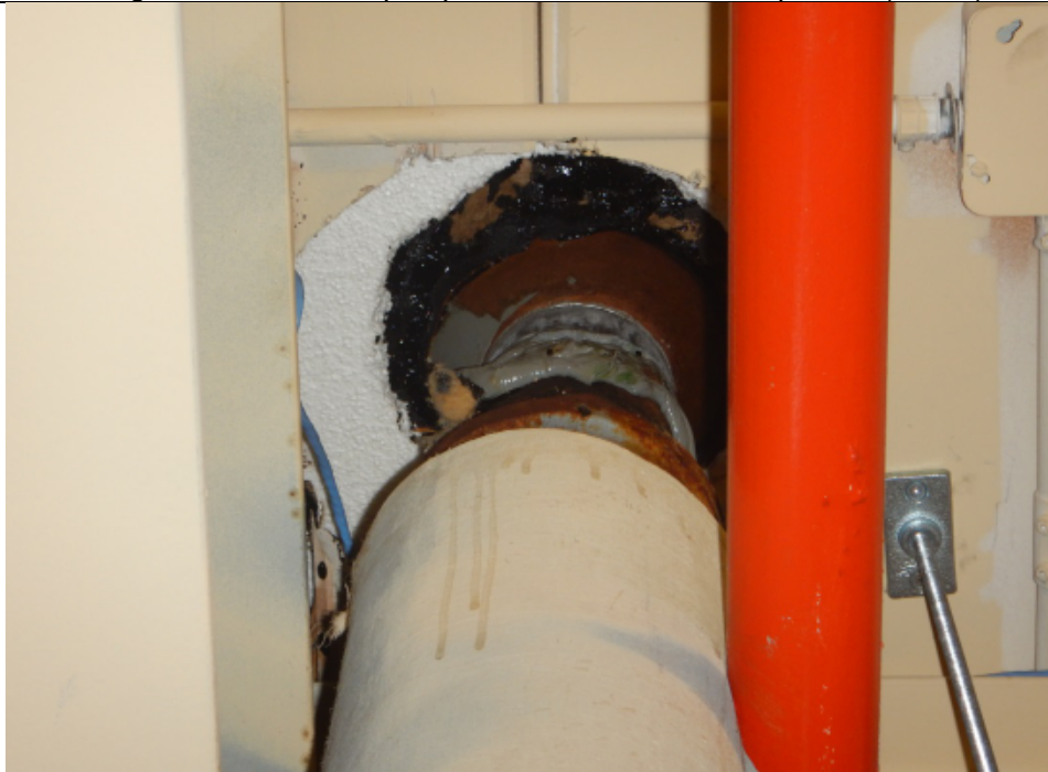
Photo 8 – The following existing roof assembly components were confirmed at one of the internal drain locations inside the building: wood fibreboard and expanded polystyrene insulation.
