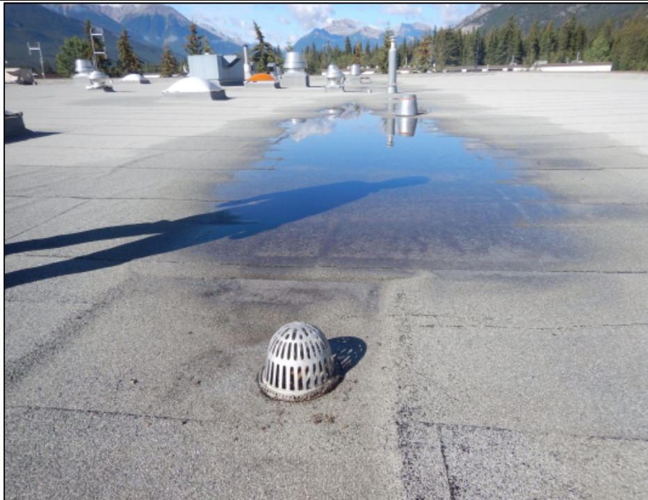
Photo 6 – Ponding was observed between internal roof drains in the central valleys of Building 1's roof.
