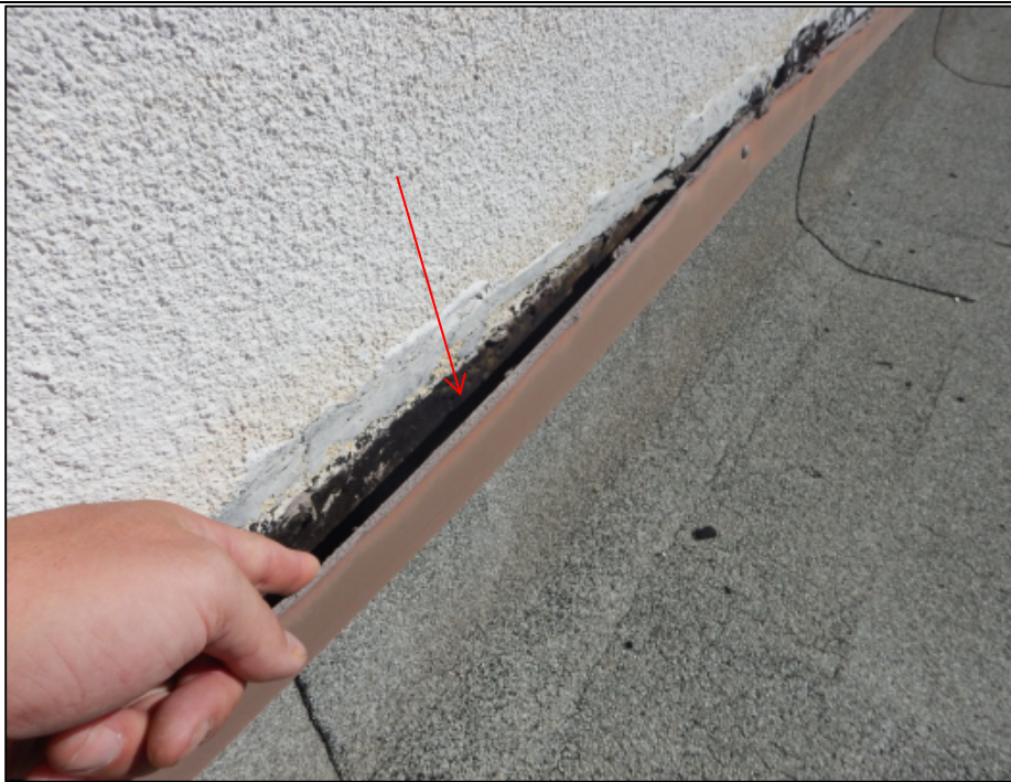
Photo 31 – The existing roof membrane stripping plies on the Garage's lower roof section are open and unsealed at the base of the stucco high walls.
