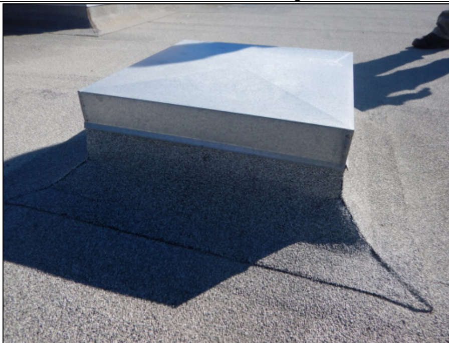
Photo 12 – Several abandoned roof penetration curbs are present on the roof of Building 1. All abandoned openings/curbs should be removed (if possible) and the wood deck in-filled with new matching decking.
