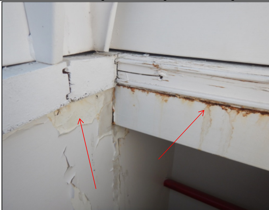
Photo 10 – Evidence of water intrusion was observed inside the roof access hatch on Building 1.
