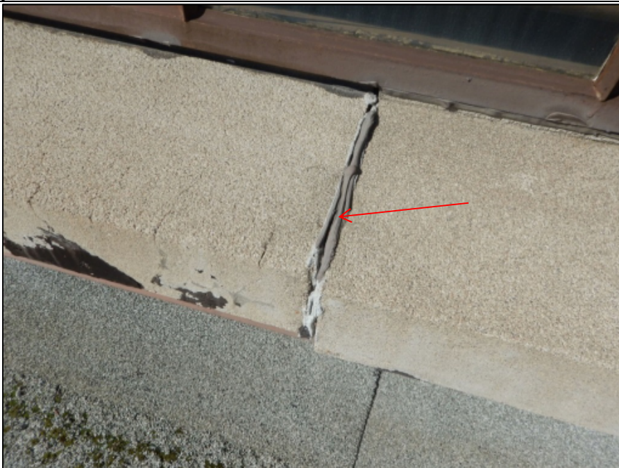
Photo 22 – The existing sealant installed between the joints of the stone window sill lintels immediately above the Garage's lower roof section has failed.
