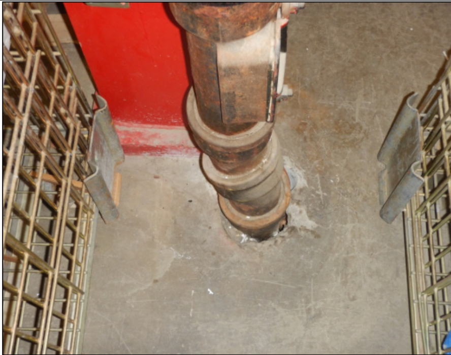
Photo 9 – The internal roof drains connect to interior rain water leaders that remove rain and melt water below grade in Building 1 and the Garage.
