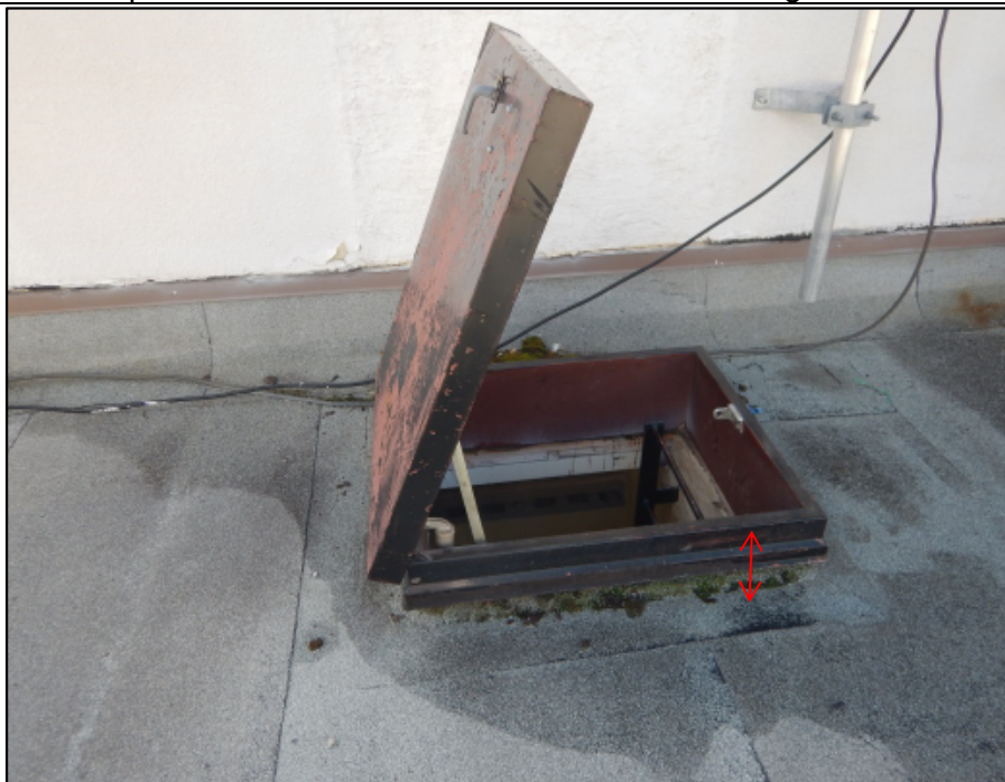
Photo 32 – The existing roof hatch curb is below 200mm in height from the finished surface of the primary roof membrane on the Garage's lower roof.
