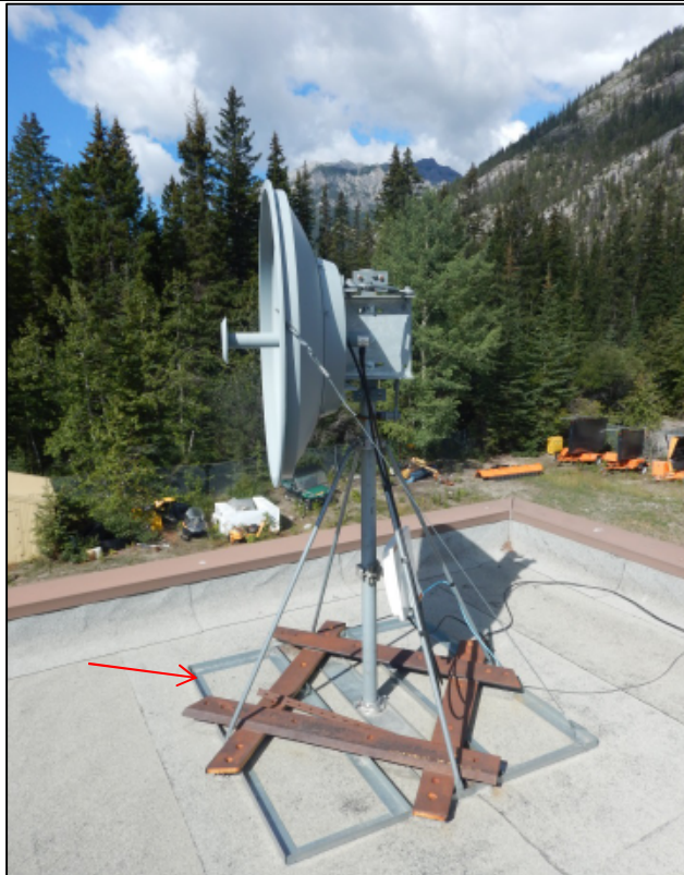
Photo 33 – Communications equipment (and stand) rests directly on the surface of the existing cap sheet.
