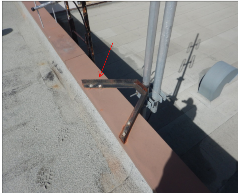
Photo 15 - Existing communications equipment will need to be removed from the fascia cladding and parapet wall caps of Building 1 and the Garage to allow for the removal of the existing roof components and installation of new roof assembly components.
