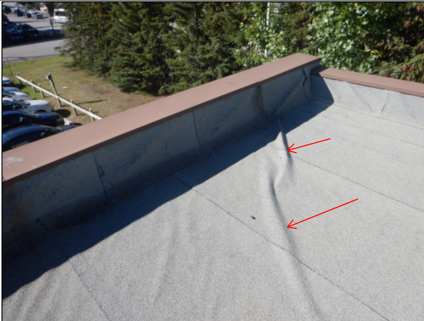
Photo 2 – Diagonal wrinkling of the roof membrane was observed throughout the field of Building1's roof.
