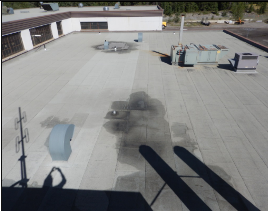
Photo 24 - Ponding was observed adjacent to the existing roof drains on the Garage's lower roof section.
