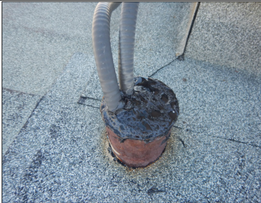
Photo 16 – Onsite personnel reported recent water intrusion into the interior space of the building at waterproofing gum boxes. Several of these gumboxes have been recently topped-up with trowel-applied mastic.
