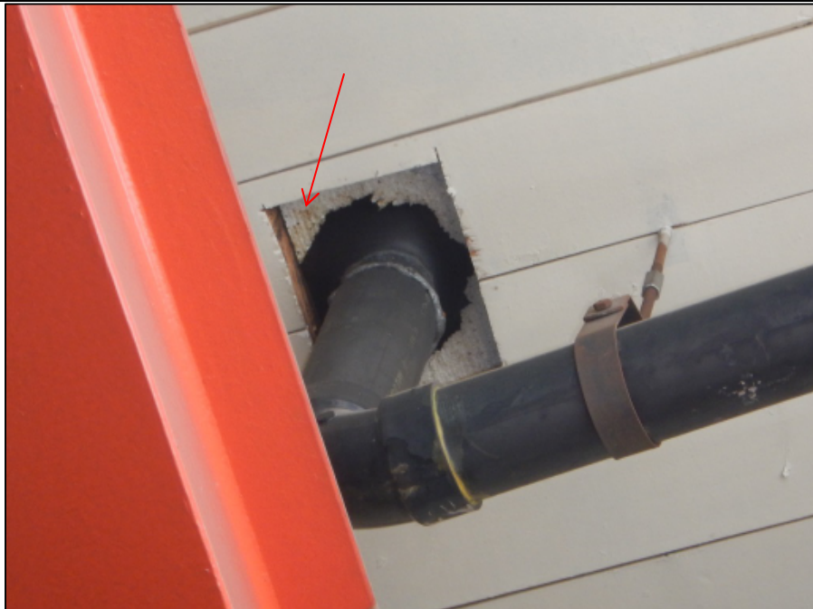
Photo 30 – Expanded polystyrene insulation was observed at an internal roof drain below the on the Garage's upper roof.
