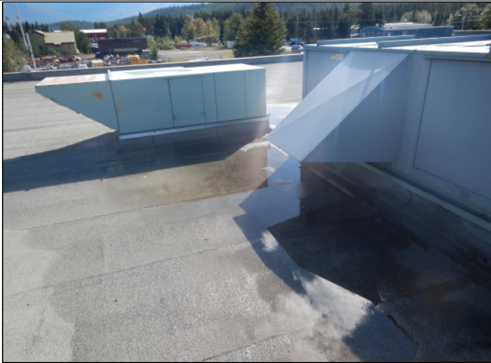
Photo 7 – Ponding was observed upslope of the curbed roof top units (RTUs) in Building 1.
