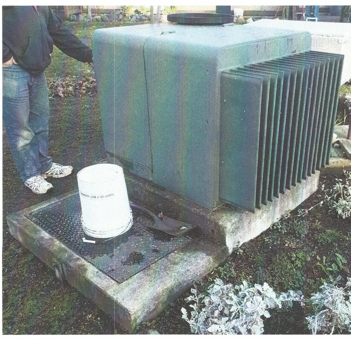
6 EXISTING PADMOUNT TRANSFORMER AND CONCRETE PAD N.T.S.
