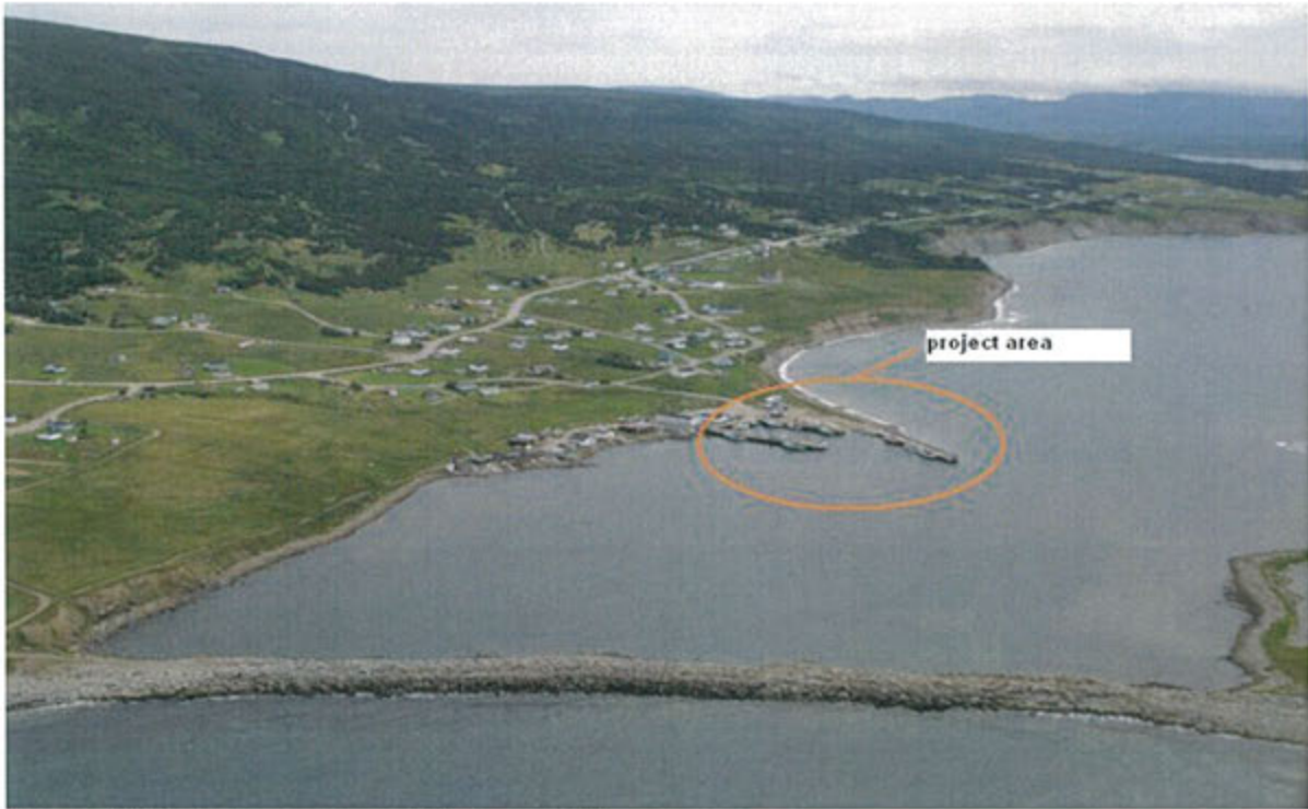
Figure 2: Aerial overview of Codroy SCH.
