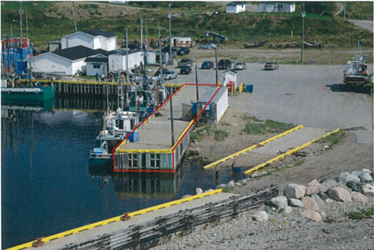
Figure 3. Section of wharf to be reconstructed (red).
