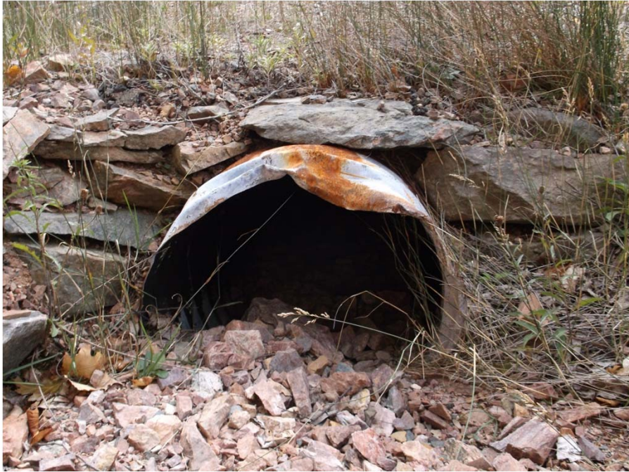
Photograph 11 – 600mm Dia. CSP Inlet @ Station 47+106.7
