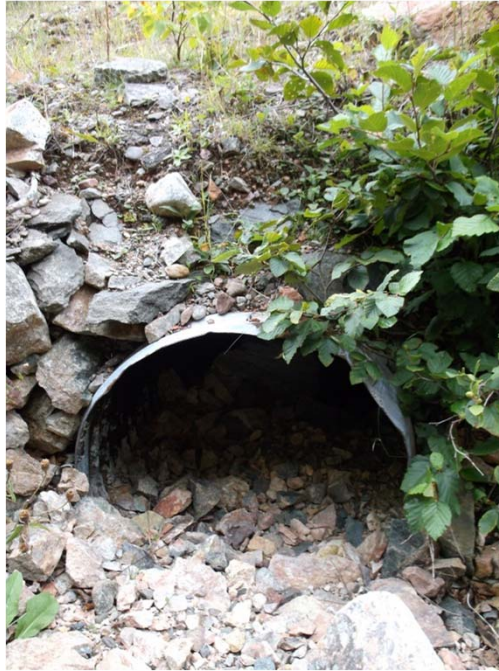
Photograph 9 – 800mm Dia. CSP Inlet @ Station 46+356.9
