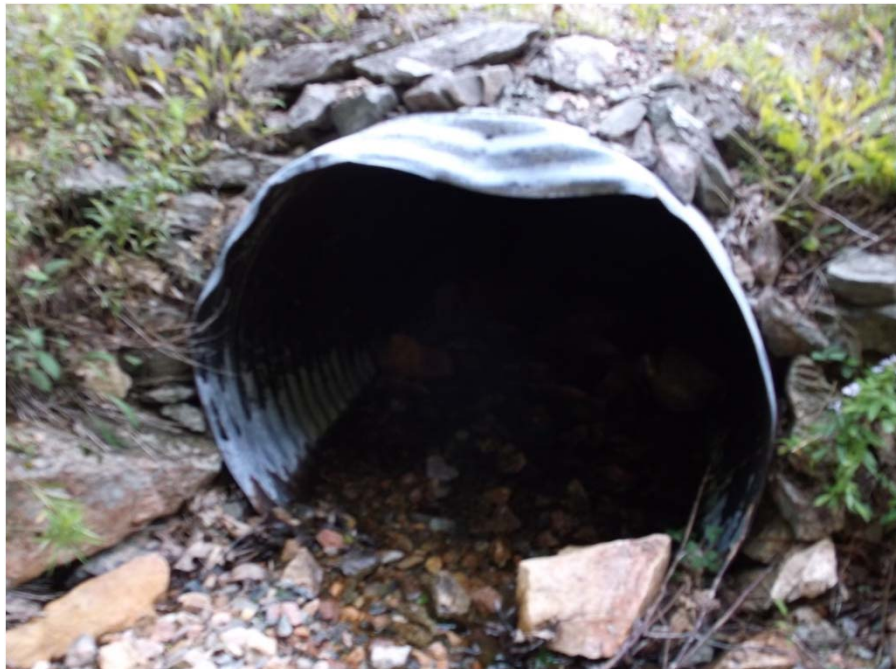
Photograph 10 – 1200mm Dia. CSP Inlet @ Station 46+898.0
