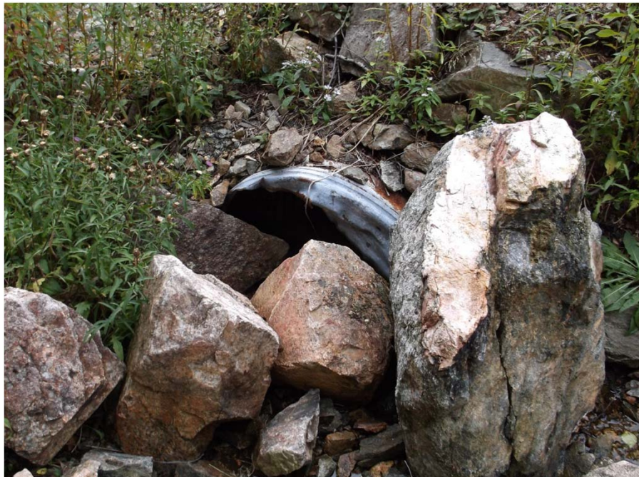
Photograph 8 – 800mm Dia. CSP Inlet @ Station 46+164.9
