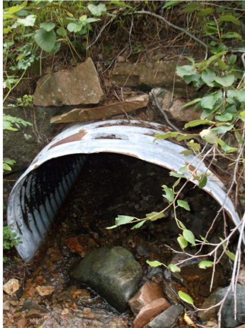
Photograph 5 – 1200mm Dia. CSP Inlet @ Station 45+724.3
