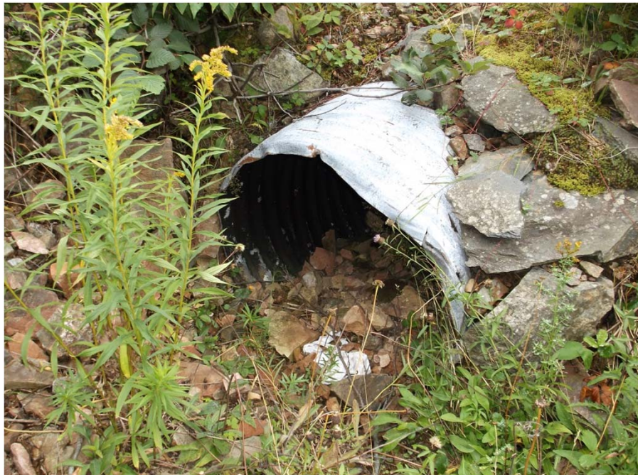
Photograph 4 – 800mm Dia. CSP Inlet @ Station 45+316.1
