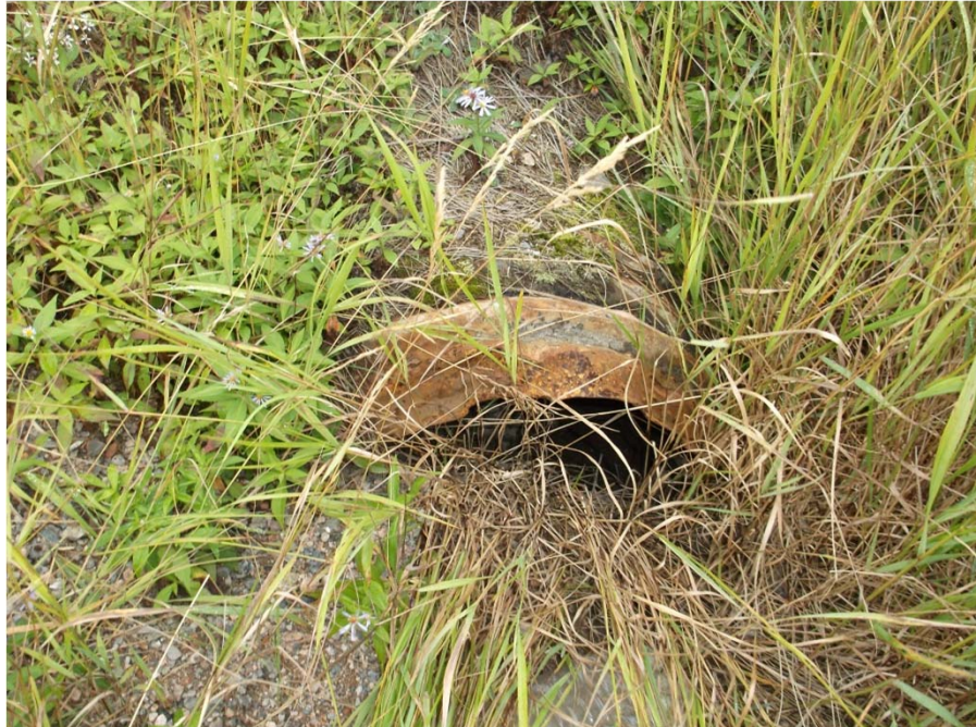
Photograph 3 – 600mm Dia. CSP Outlet @ Station 44+583.2
