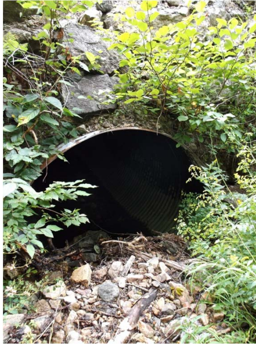
Photograph 7 – 1800mm Dia. CSP Inlet @ Station 46+064.0
