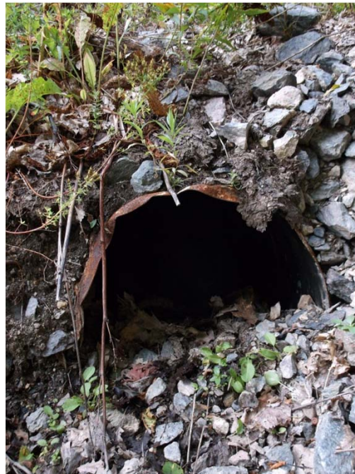
Photograph 2 – 600mm Dia. CSP Inlet @ Station 39+786.6
