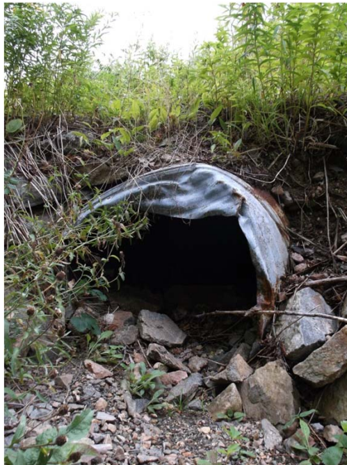
Photograph 6 – 800mm Dia. CSP Inlet @ Station 45+918.6
