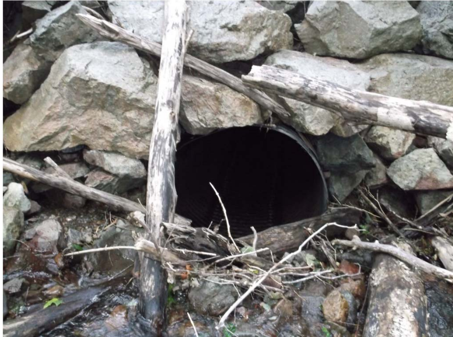
Photograph 1 – 1200mm Dia. CSP Inlet @ Station 38+379.2
