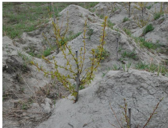
Photograph 5 (left) and 6 (right). Live staking in the rough and loose soils of this tailings pond is easy and allows the cuttings to grow rapidly (right, start of 2 nd year growth for cuttings)
