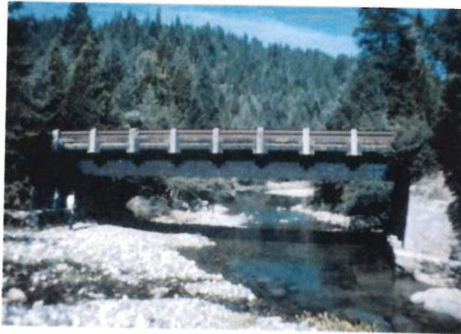
Figure 4.2 Oilborne preservatives are often used for treatment of glulam beams, such as in this bridge (Lebow and Tippie, 2001).
