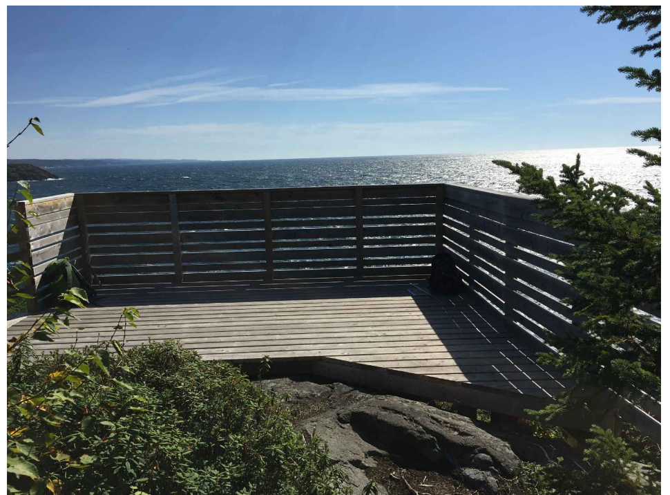
VIEW OF STRUCTURE FACING WEST
