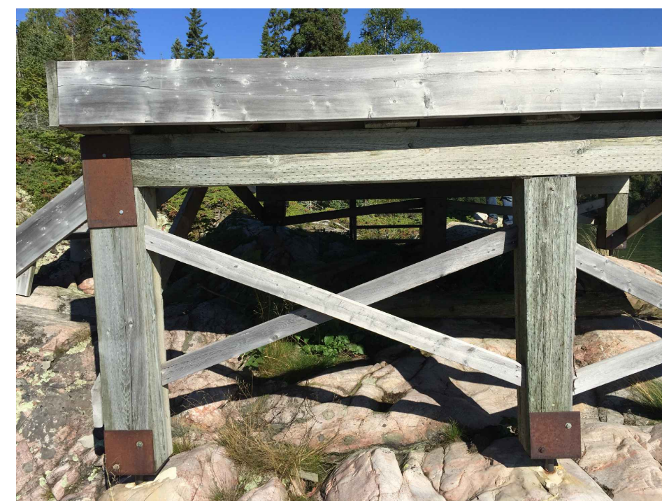
VIEW OF STRUCTURE FACING NORTH
