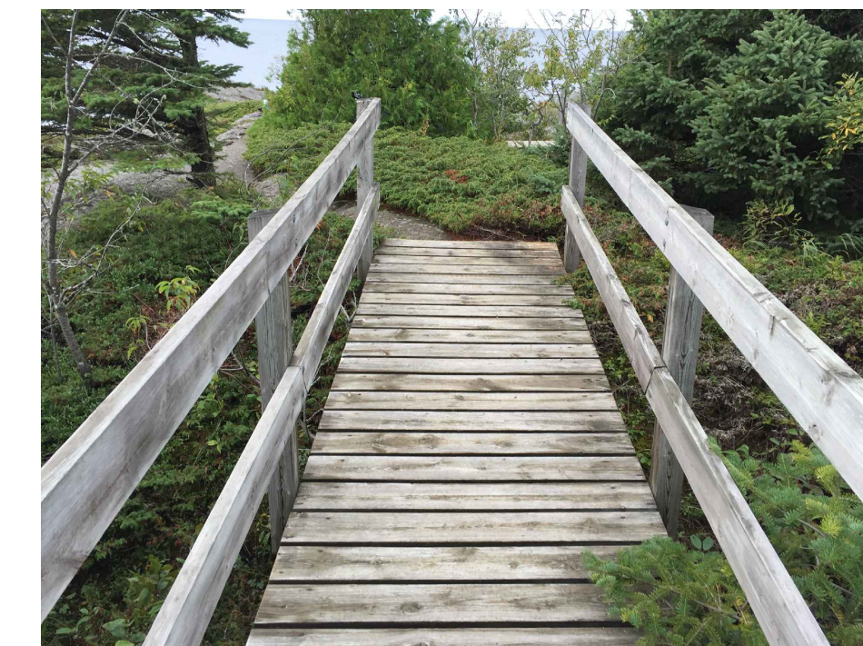
VIEW OF STRUCTURE FACING SOUTH
