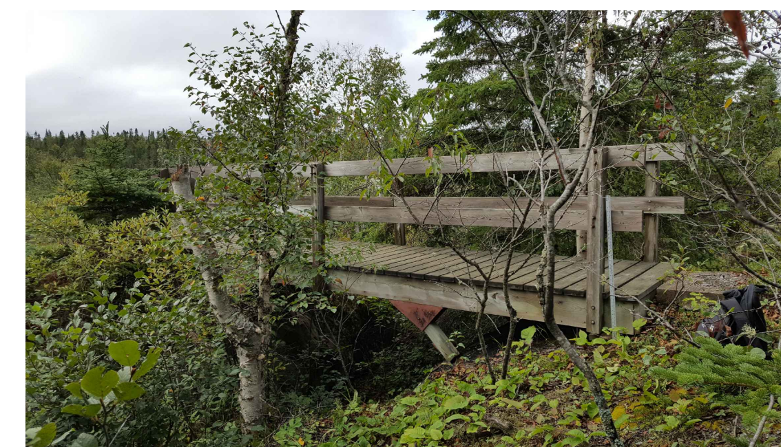
VIEW OF STRUCTURE FACING NORTHEAST
