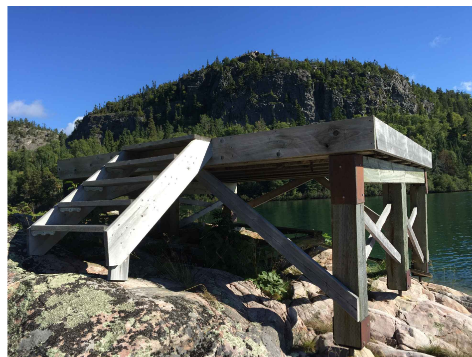
VIEW OF STRUCTURE FACING EAST
