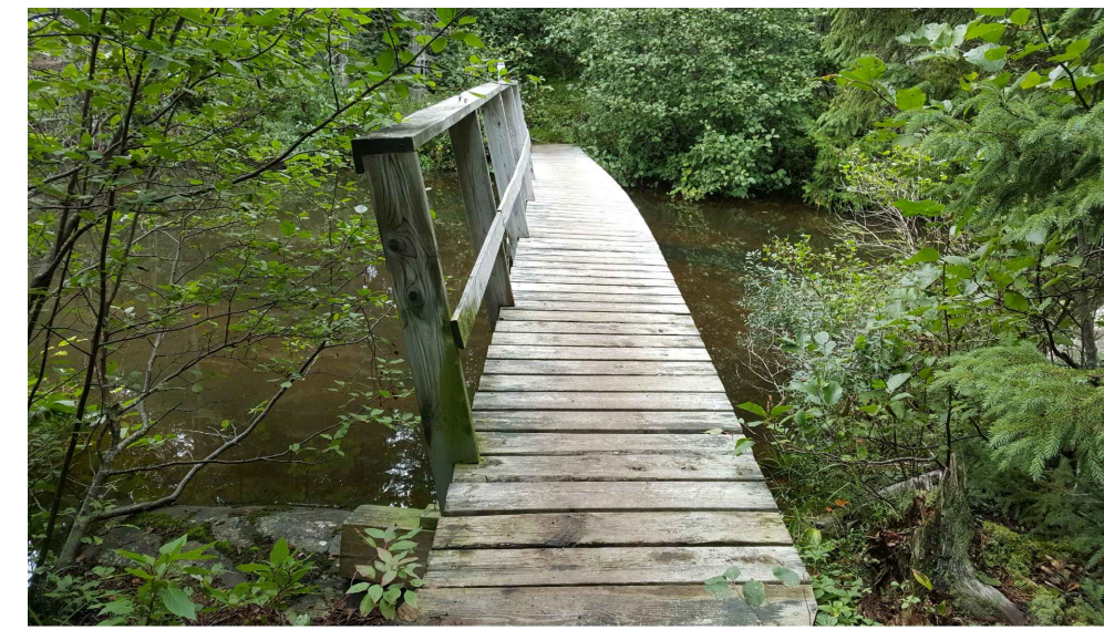
VIEW OF STRUCTURE FACING NORTH
