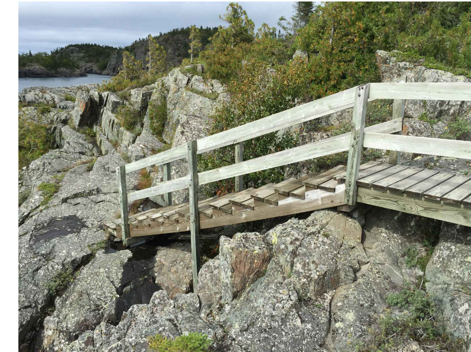
VIEW OF STRUCTURE FACING NORTHEAST
