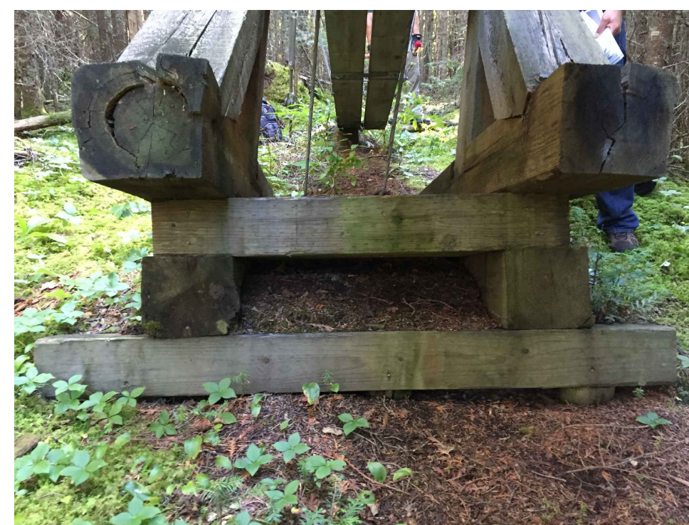
SOUTH ABUTMENT STRUCTURE
