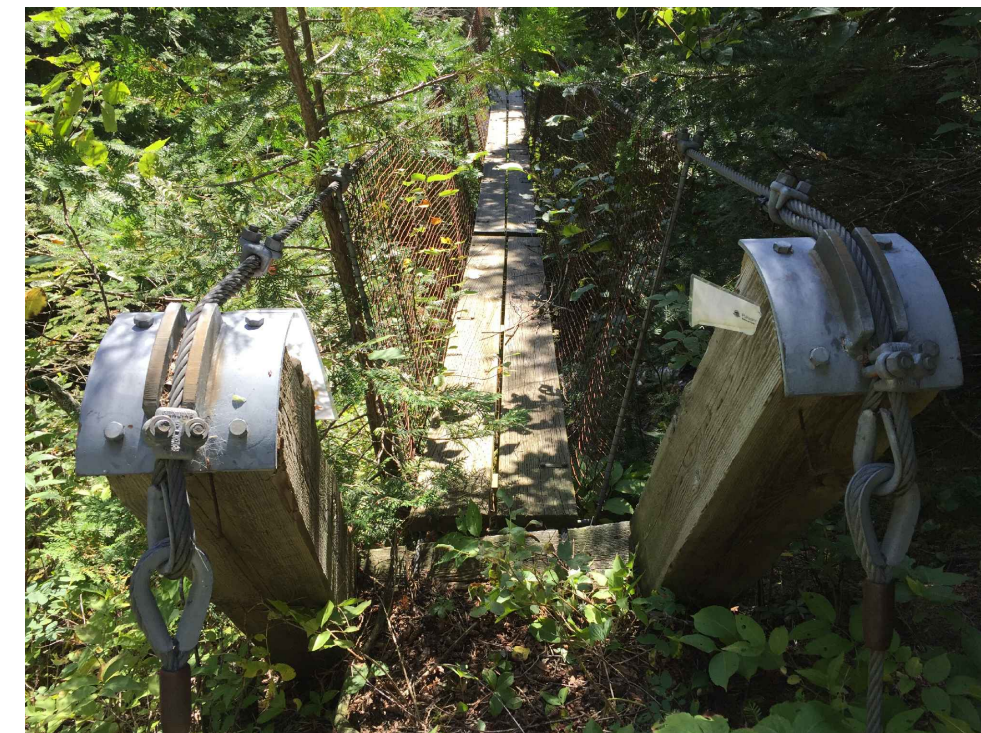
NORTH ABUTMENT STRUCTURE
