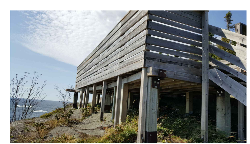
VIEW OF STRUCTURE FACING NORTHEAST
