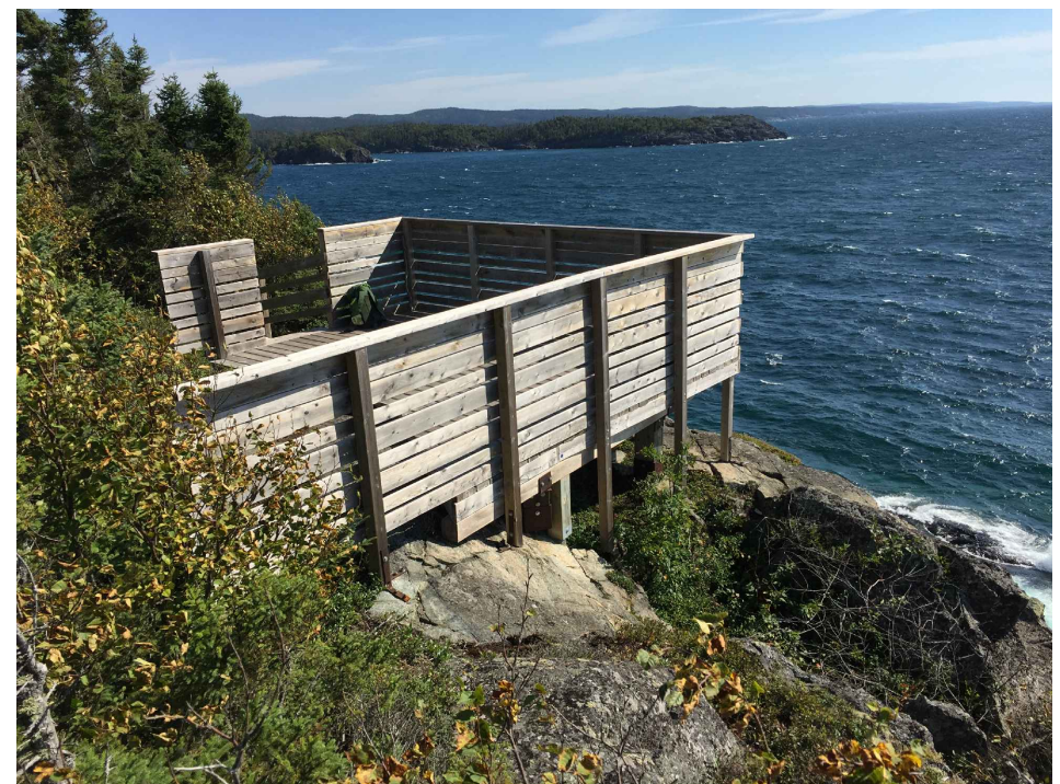
VIEW OF STRUCTURE FACING SOUTHWEST
