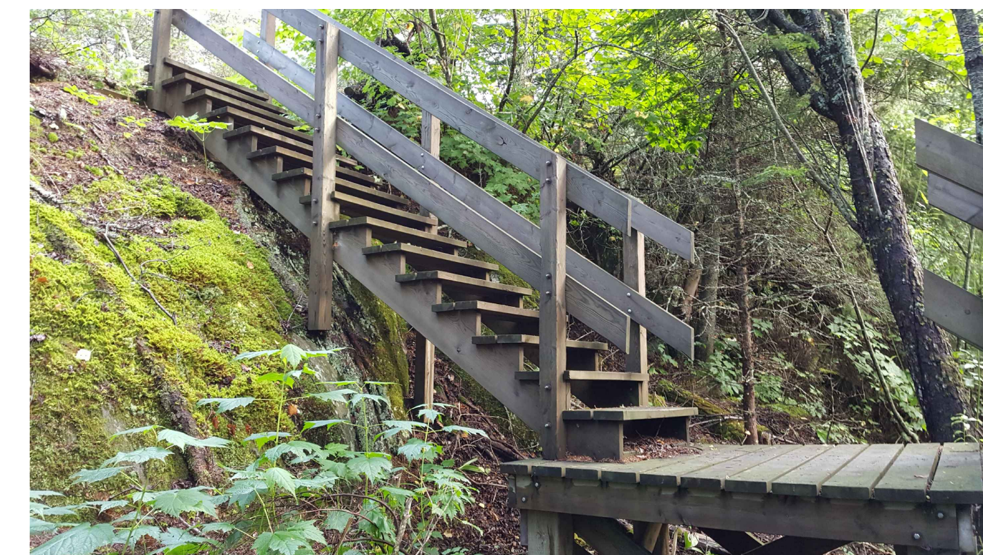
VIEW OF STRUCTURE FACING NORTHEAST
