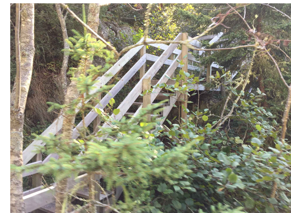
VIEW OF WEST STAIRS FACING NORTHWEST
