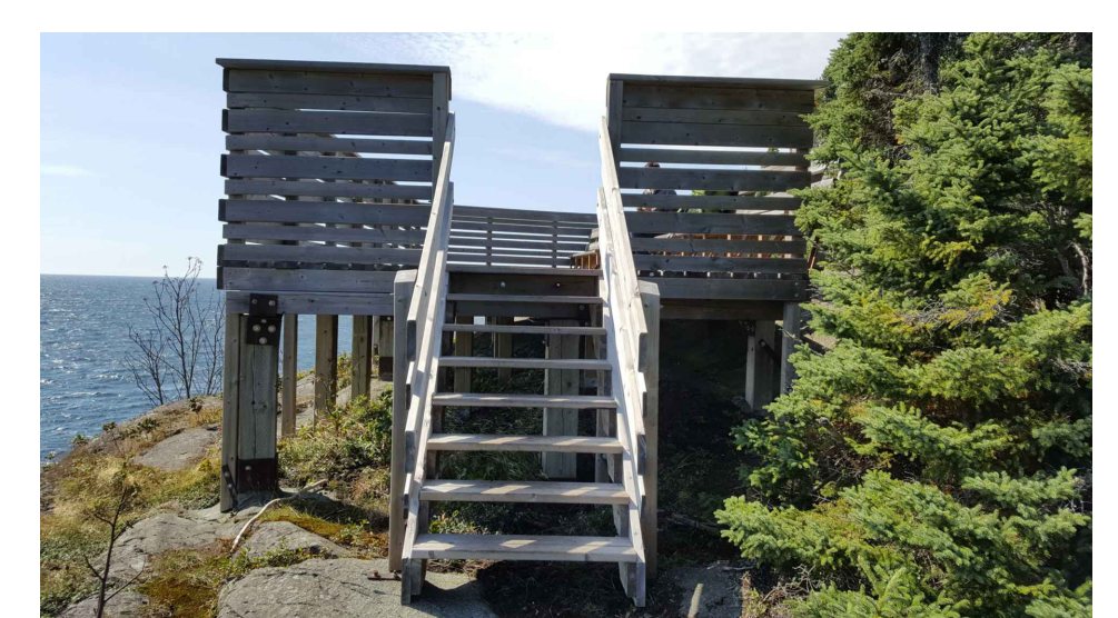
VIEW OF STRUCTURE FACING NORTH
