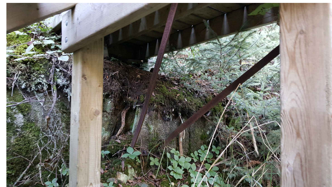
VIEW OF EX. STEEL BRACES TO BE PAINTED
