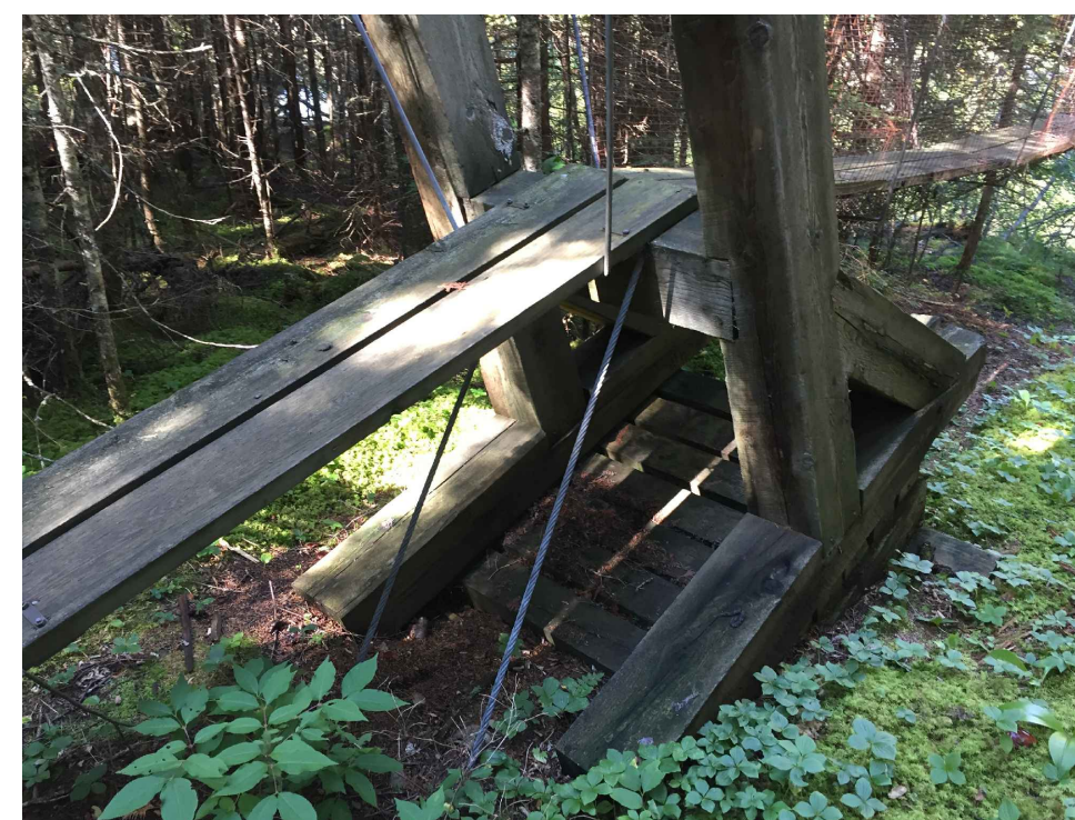
SOUTH ABUTMENT STRUCTURE
