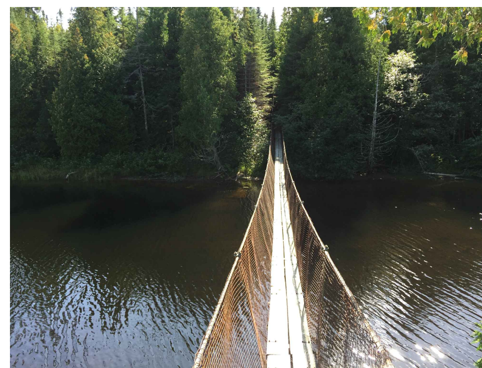
SUSPENSION BRIDGE STRUCTURE
