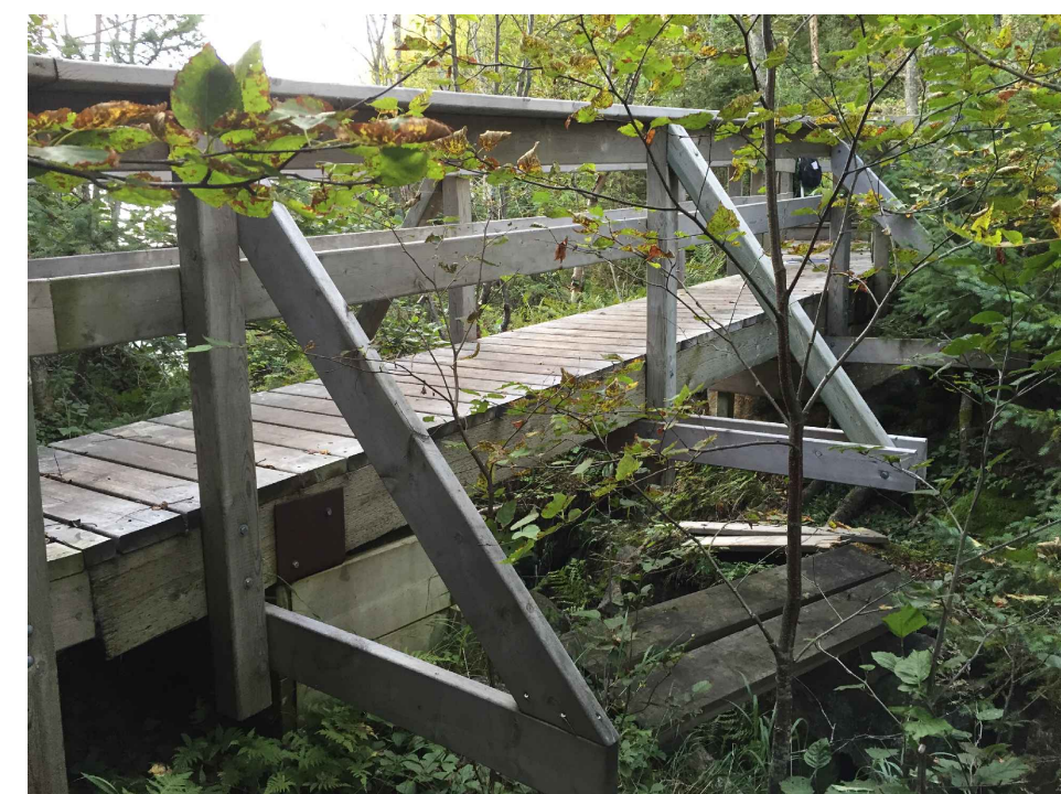
VIEW OF RAVINE CROSSING FACING SOUTHWEST
