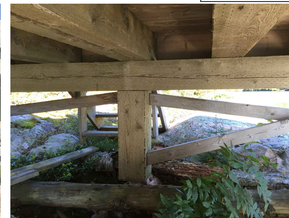
UNDERSIDE VIEW OF STRUCTURE FACING NORTH
