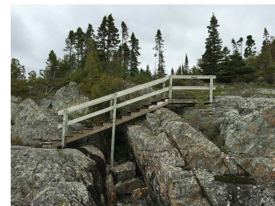
VIEW OF STRUCTURE FACING EAST
