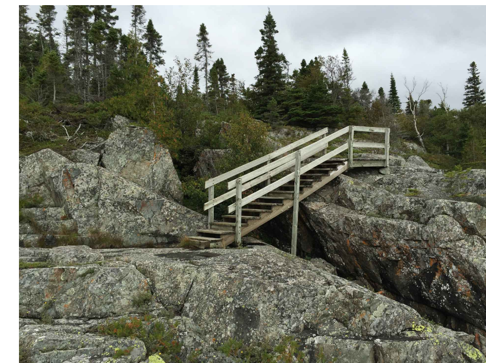
VIEW OF STRUCTURE FACING SOUTHEAST
