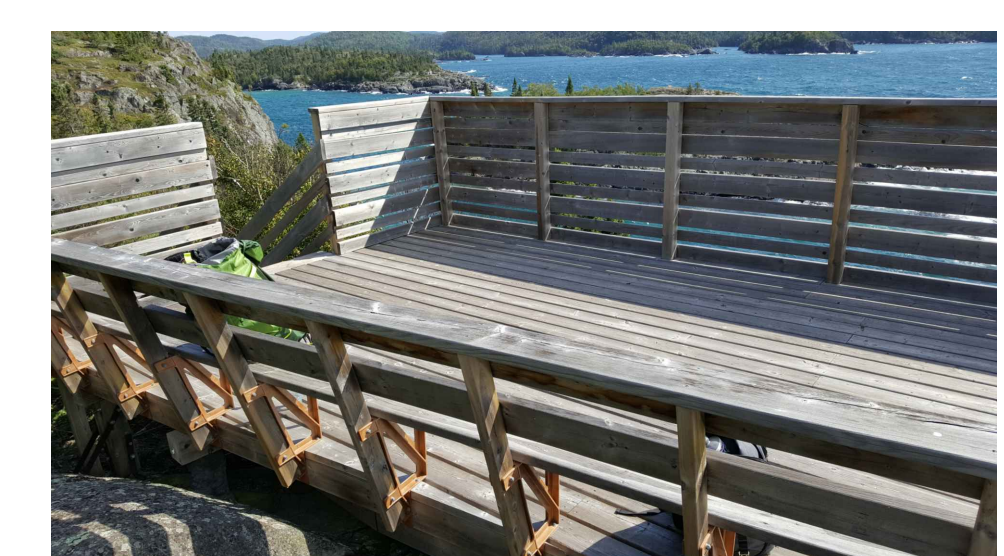
VIEW OF STRUCTURE FACING SOUTHWEST
