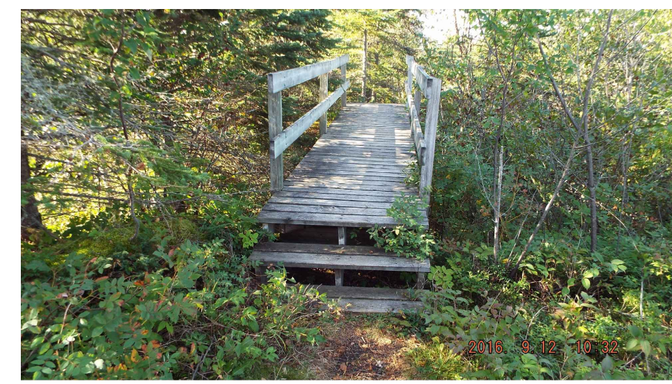
VIEW OF STRUCTURE FACING SOUTH
