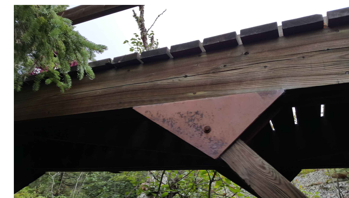
VIEW OF STRUCTURAL KNEE BRACING
