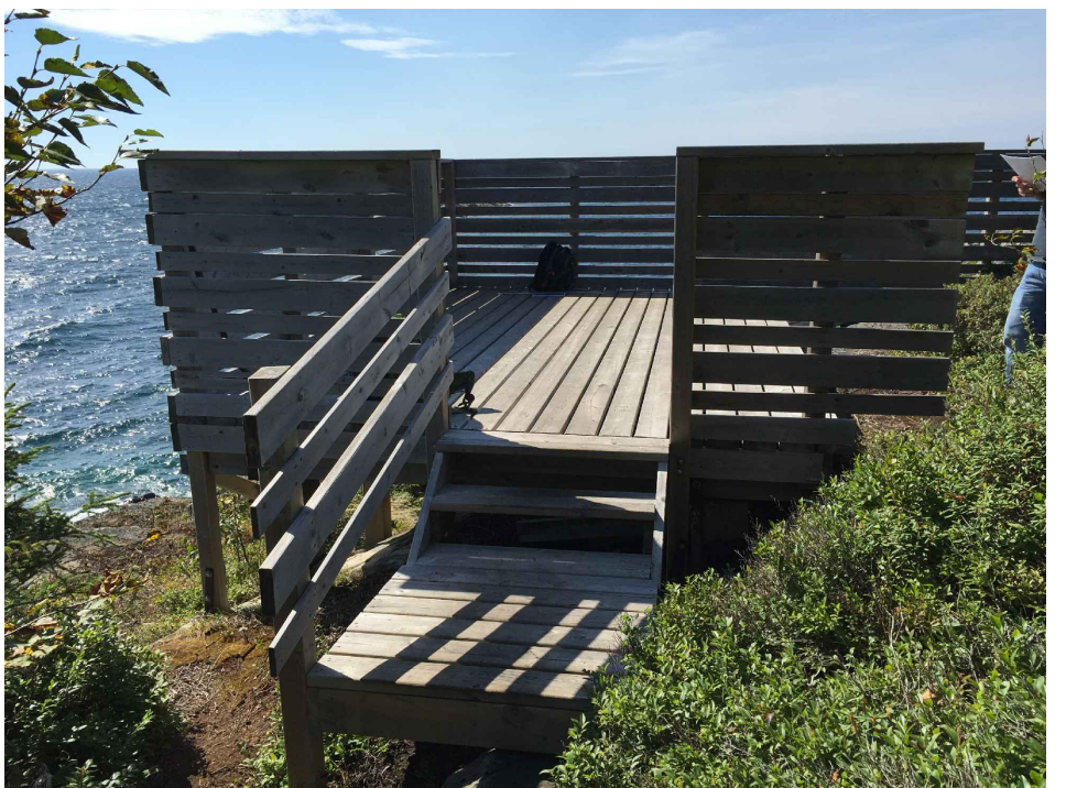
VIEW OF STRUCTURE FACING NORTH
