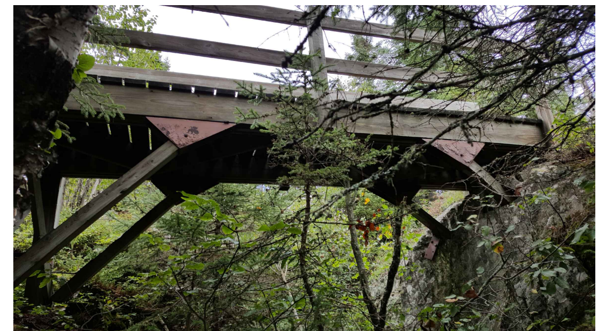
UNDERSIDE VIEW OF STRUCTURE
