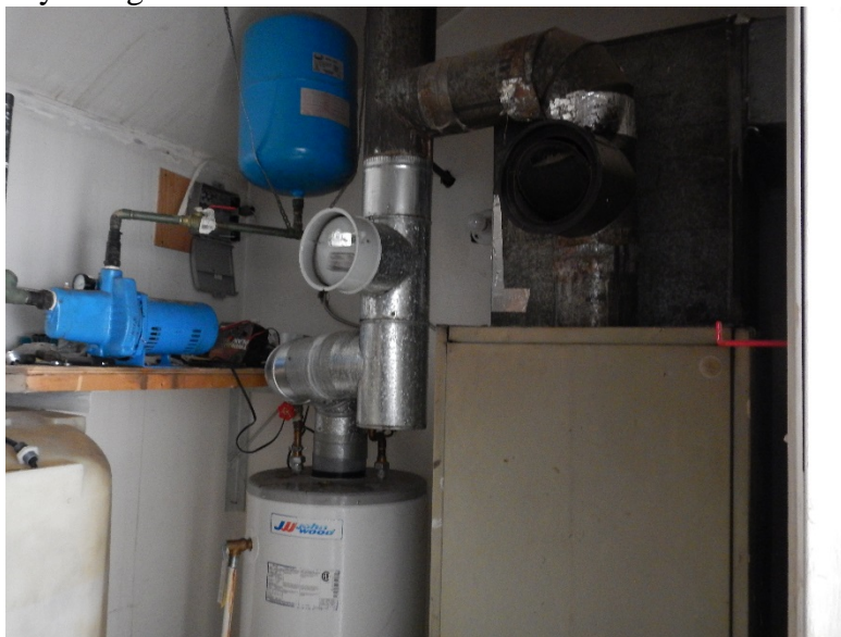
Figure 4 Pump and pressure tank
