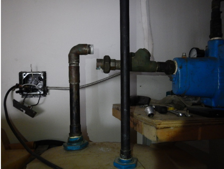
Figure 3 Replace pump and reconnect all piping.
