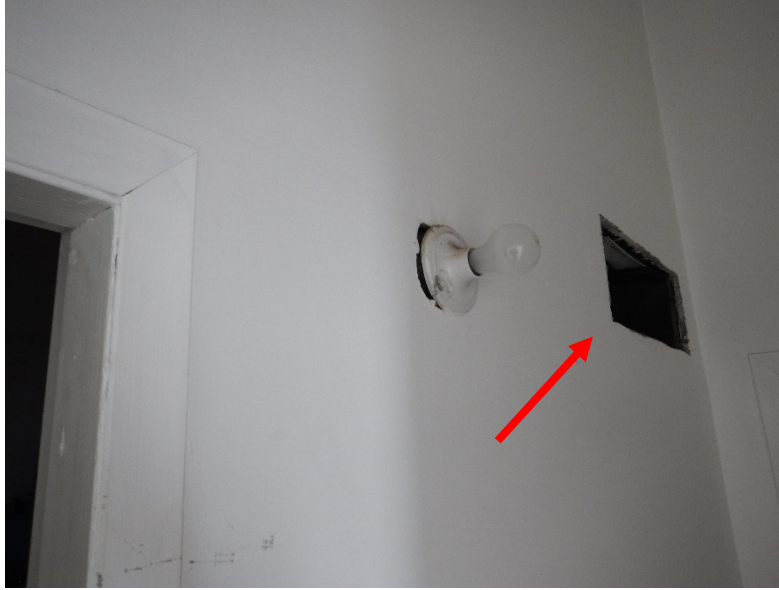
Figure 1 Supply and install missing grill on return air duct.
