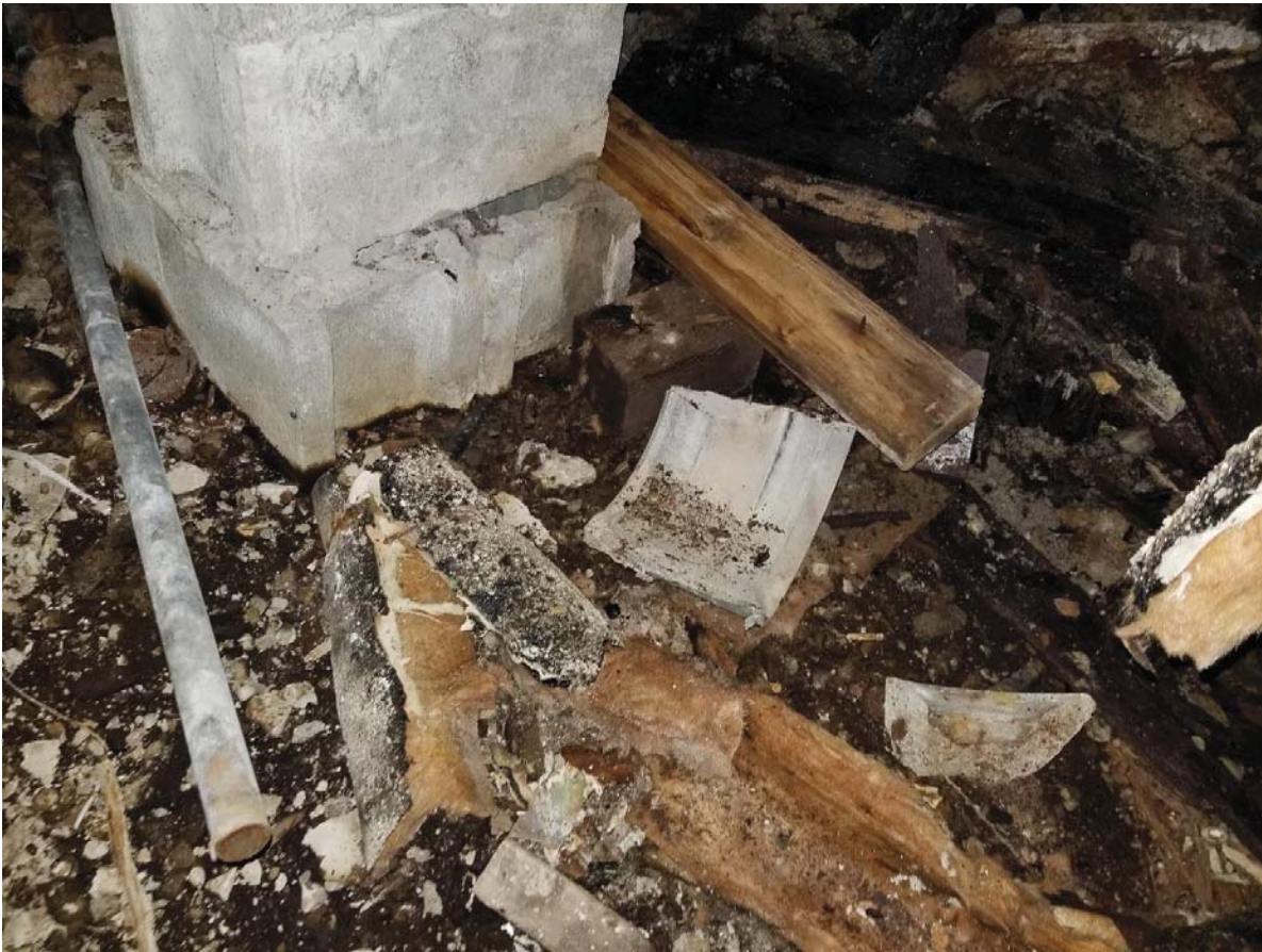
Photograph 1: Historic Bridge Tie-in Transite Pipe Debris
