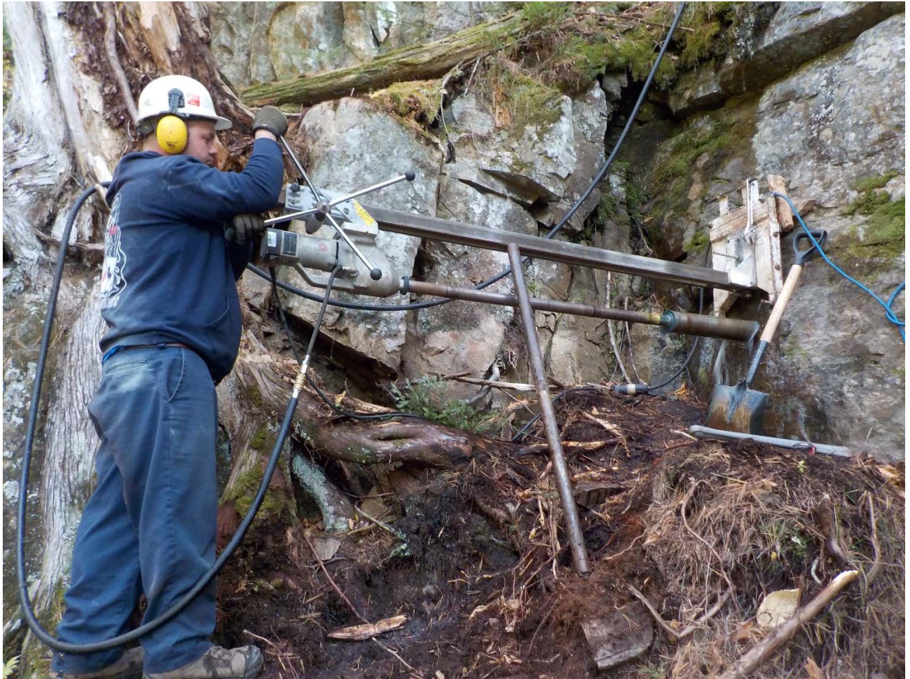
Figure 2 Drilling of a horizontal borehole (BH-03-16)
