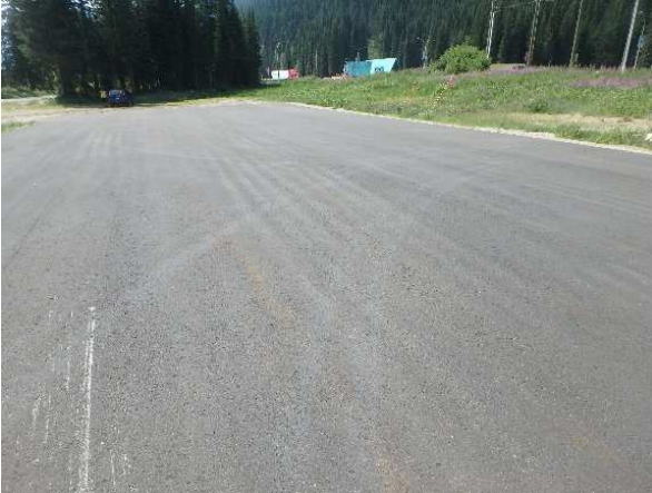
Photo 15 – Helipad / Snow Storage Area
