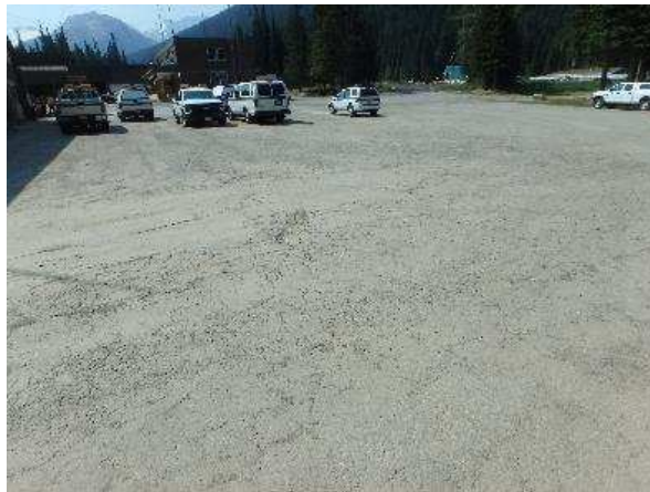
Photo 10 – West of Office Building
