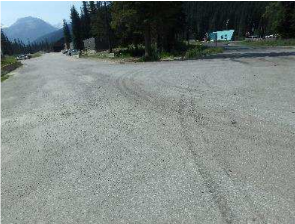
Photo 7 – At Office Building
