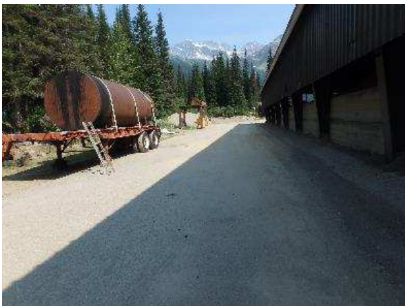
Photo 1 – West of Abrasives Storage Shed
