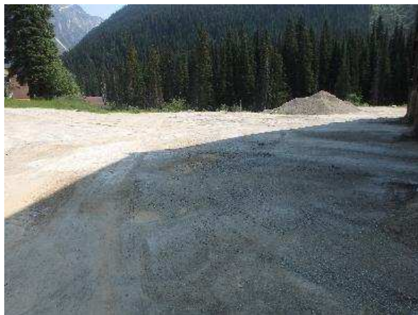
Photo 2 – North of Abrasives Storage Shed
