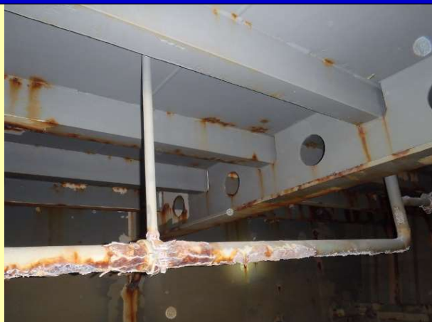
Typical breakdown along the edges and welds, brackets and pipes are also in poor repair
