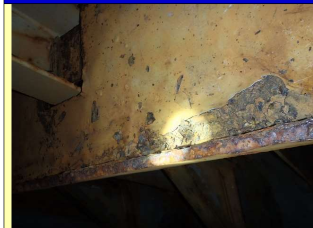
Close up of typical breakdown and steel loss
