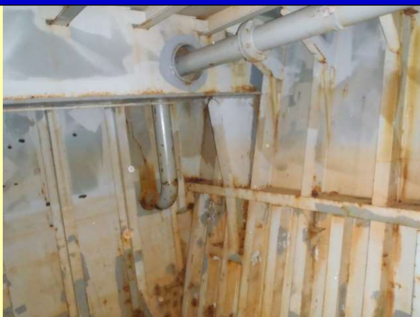
General condition with breakdown on the edges and welds resulting in staining
