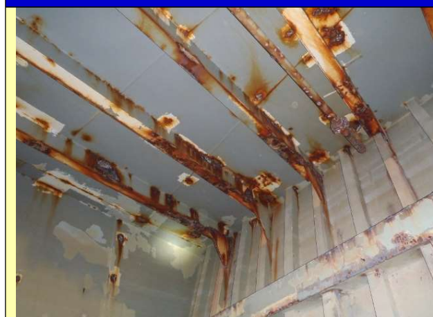
Typical breakdown along the edges and welds, brackets and pipes are also in poor repair. Flat areas are in average condition
