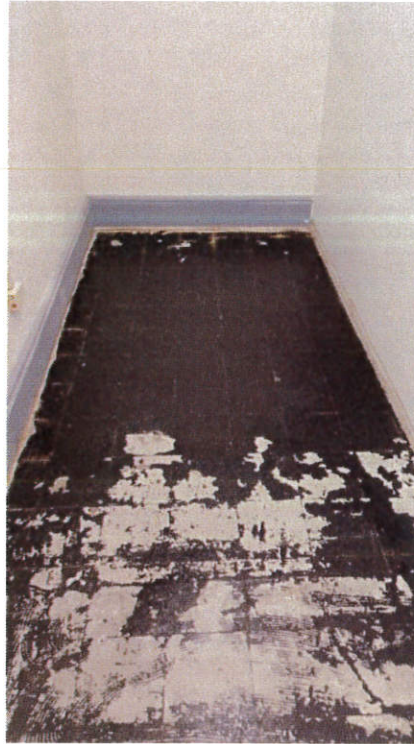
Photo 1: Asbestos-containing remnant mastic and floor levelling compound in Room 133 at the M-2 Building.
