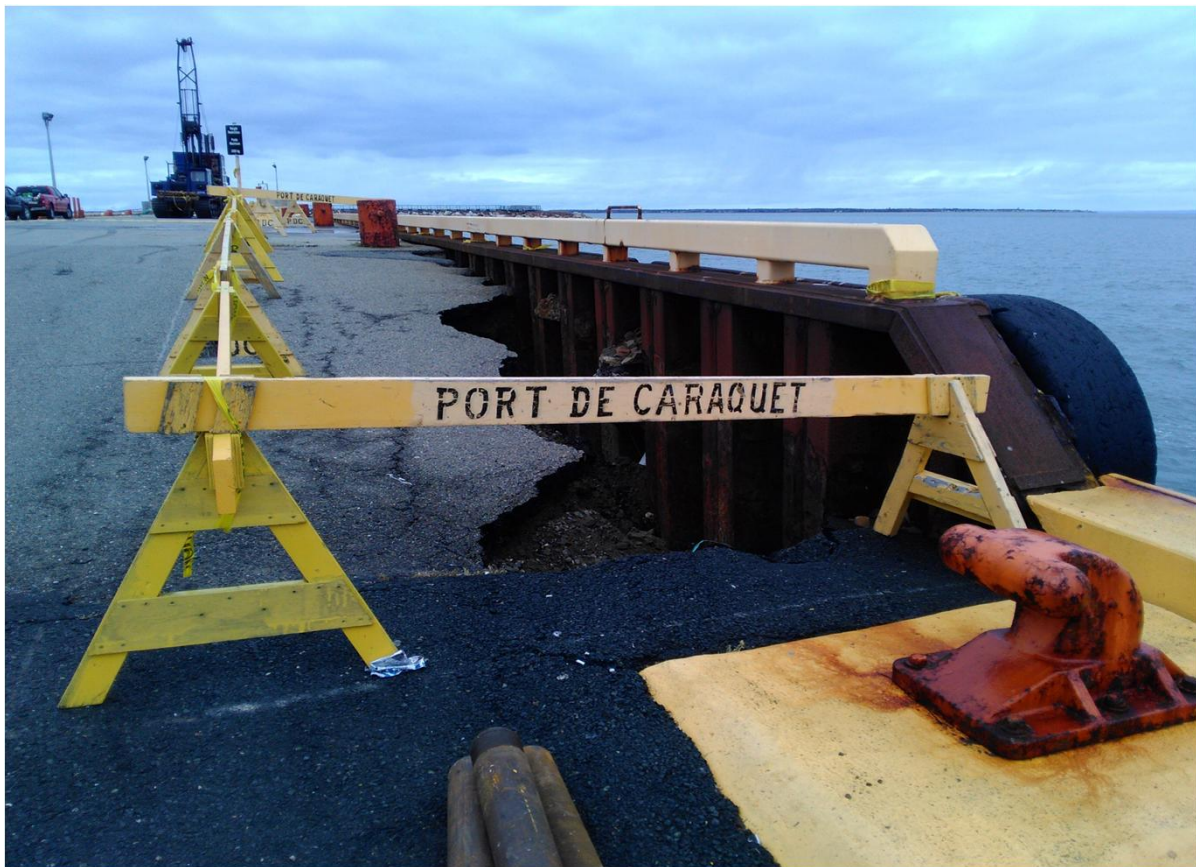
Photo 4: Deterioration of Wharf 405 observed along northern edge, looking west.
