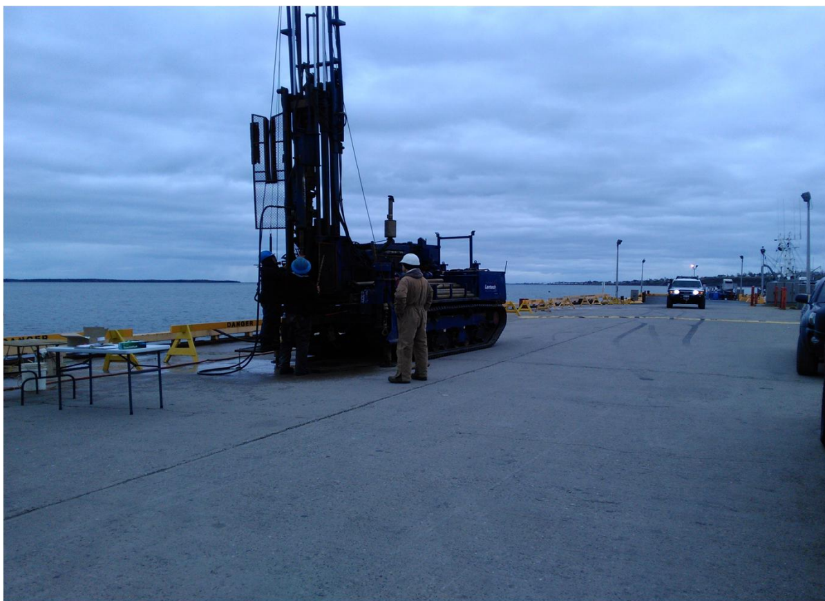
Photo 2: Looking east at the track mounted drill rig at sample location BH16-06.
