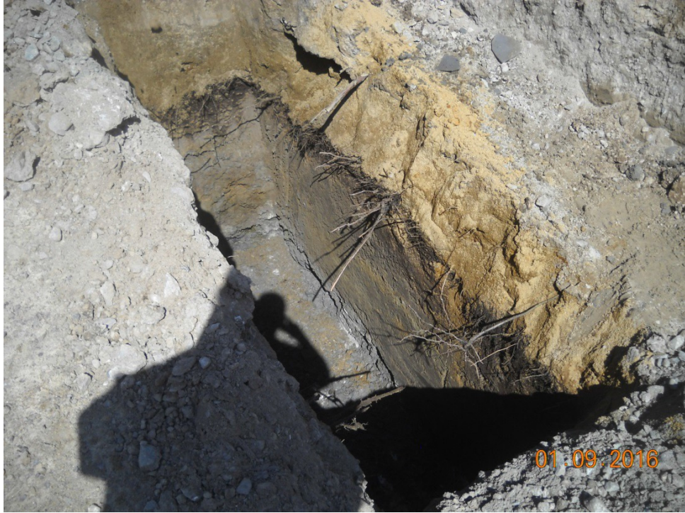
Picture 9 : Example of exploration well walls (2/2)
