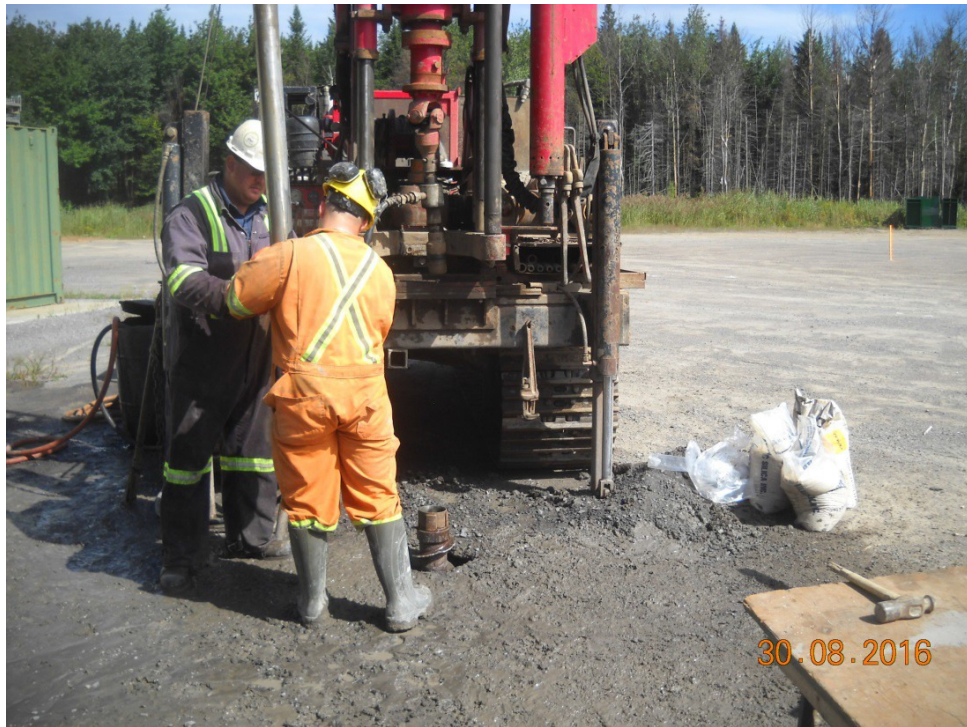
Picture 3 : Realization of hollow auger boreholes
