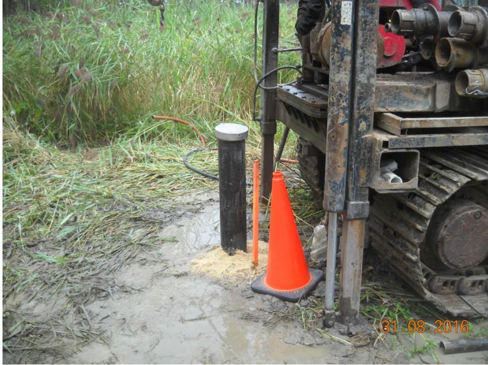
Picture 5 : Development of an observation well – Above-ground protection
