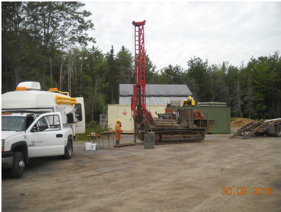
Picture 2 : Diedrich Model D-50 Crawler mounted drill rig
