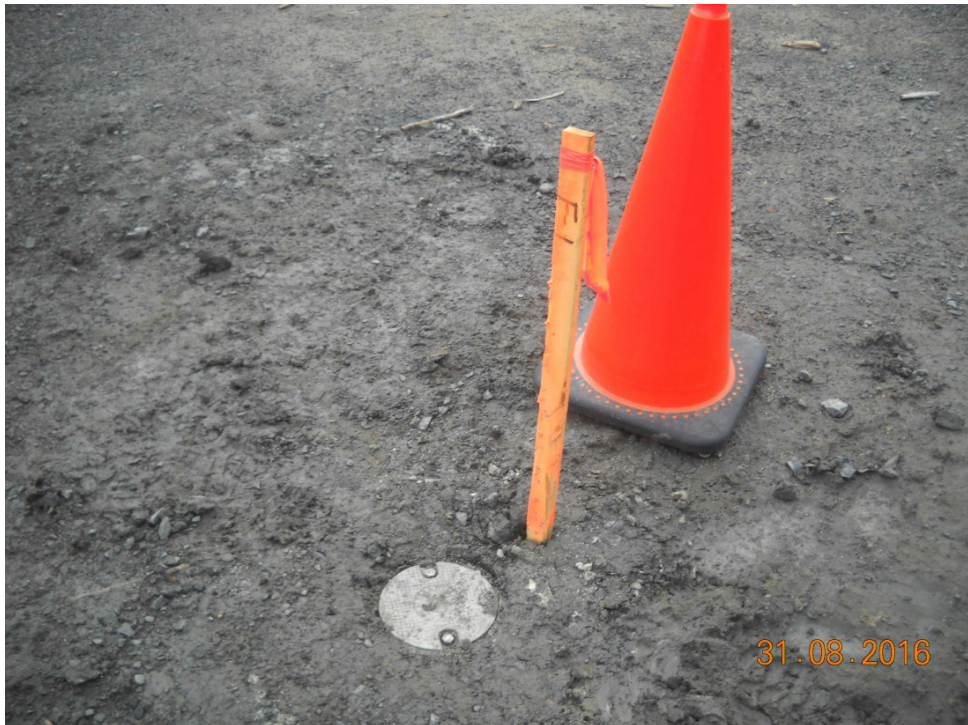
Picture 6 : Development of an observation well – Low level protection
