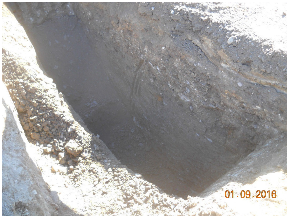
Picture 8 : Example of exploration well walls (1/2)
