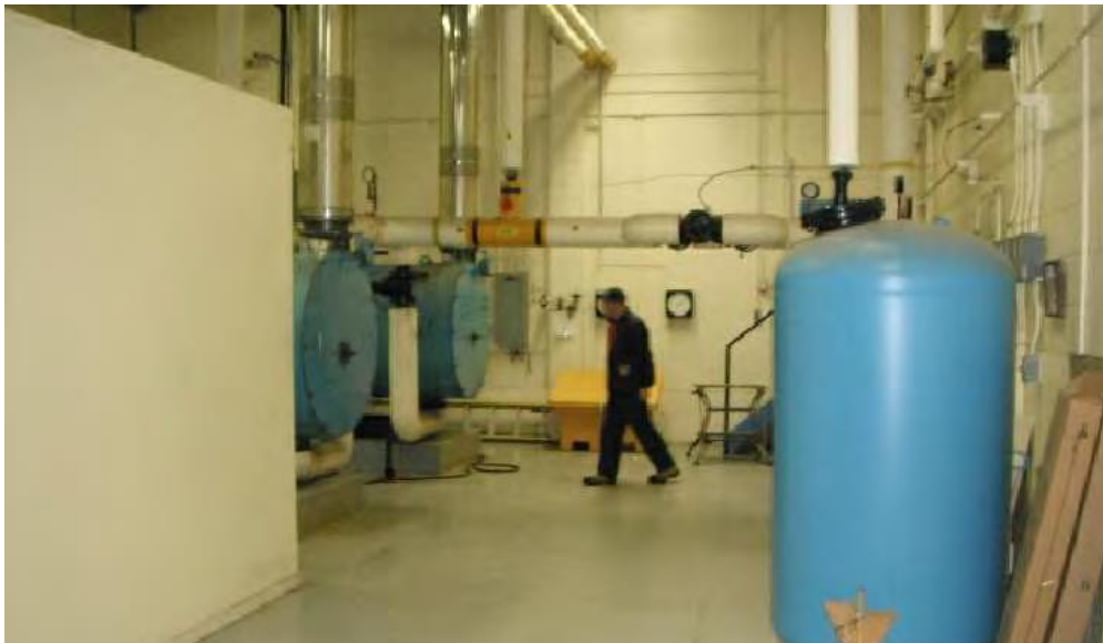
Mechanical Room in Combined Services Building – the Pipe Insulation contains Asbestos
