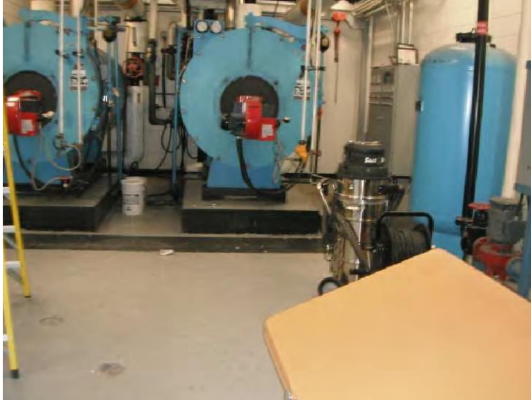
Mechanical Room in Air Terminal Building – the Pipe Insulation contains Asbestos
